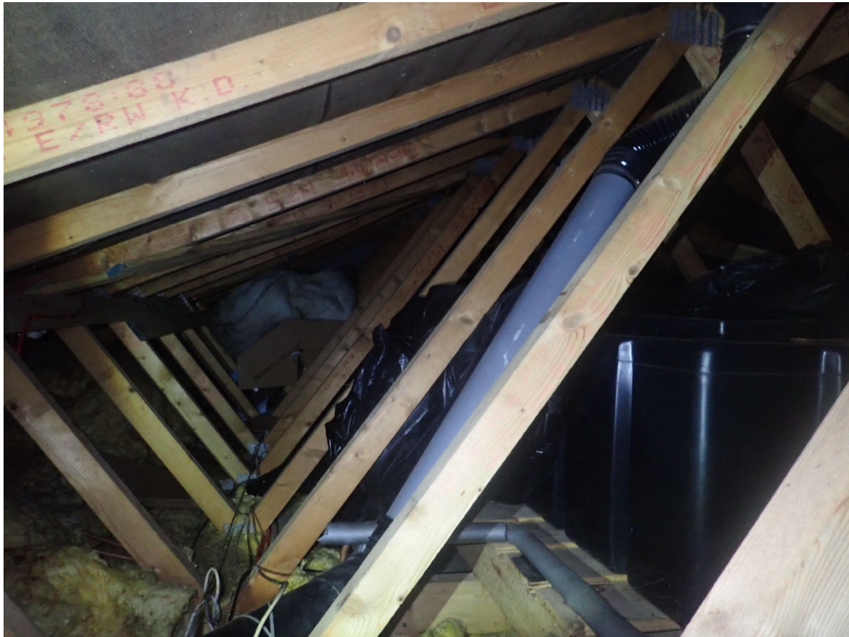
3.2a – The roof void.
