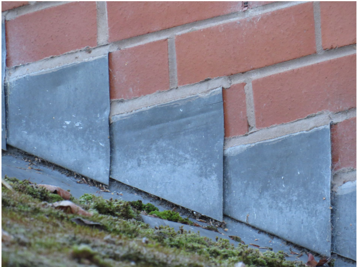
9 – Lead flashing is in good condition with no viable gaps.
