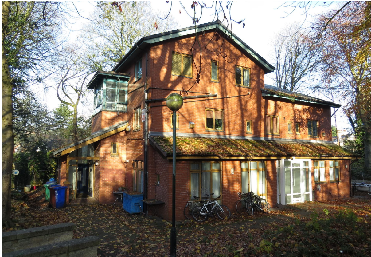
1 – The front of the building.
