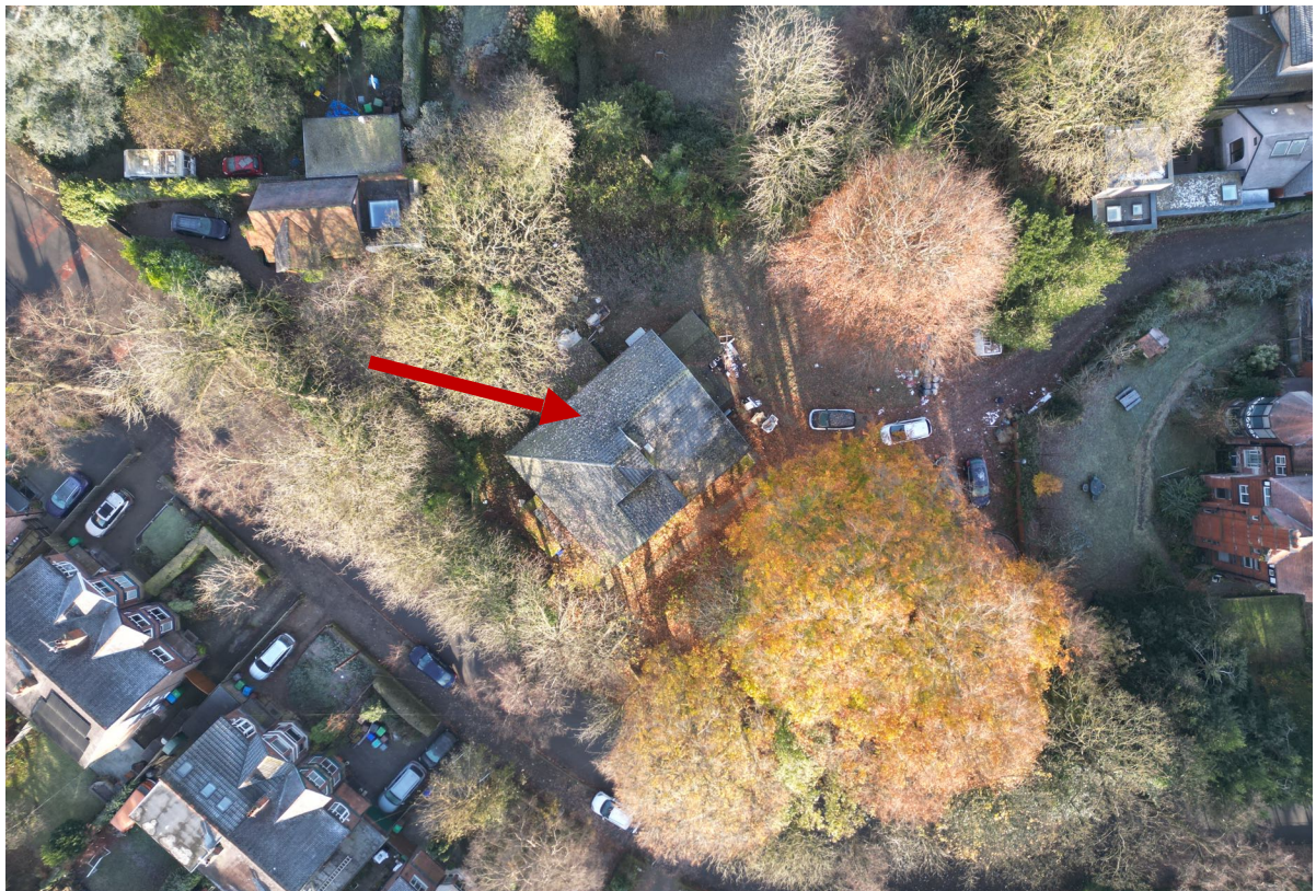
1.6b – 60a Wood Road – aerial photograph.
