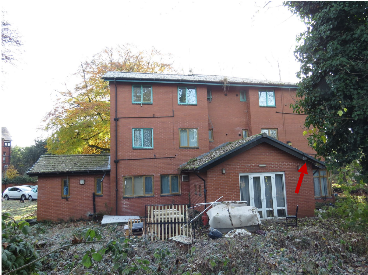
2 – The rear of the building with damaged fascia indicated.
