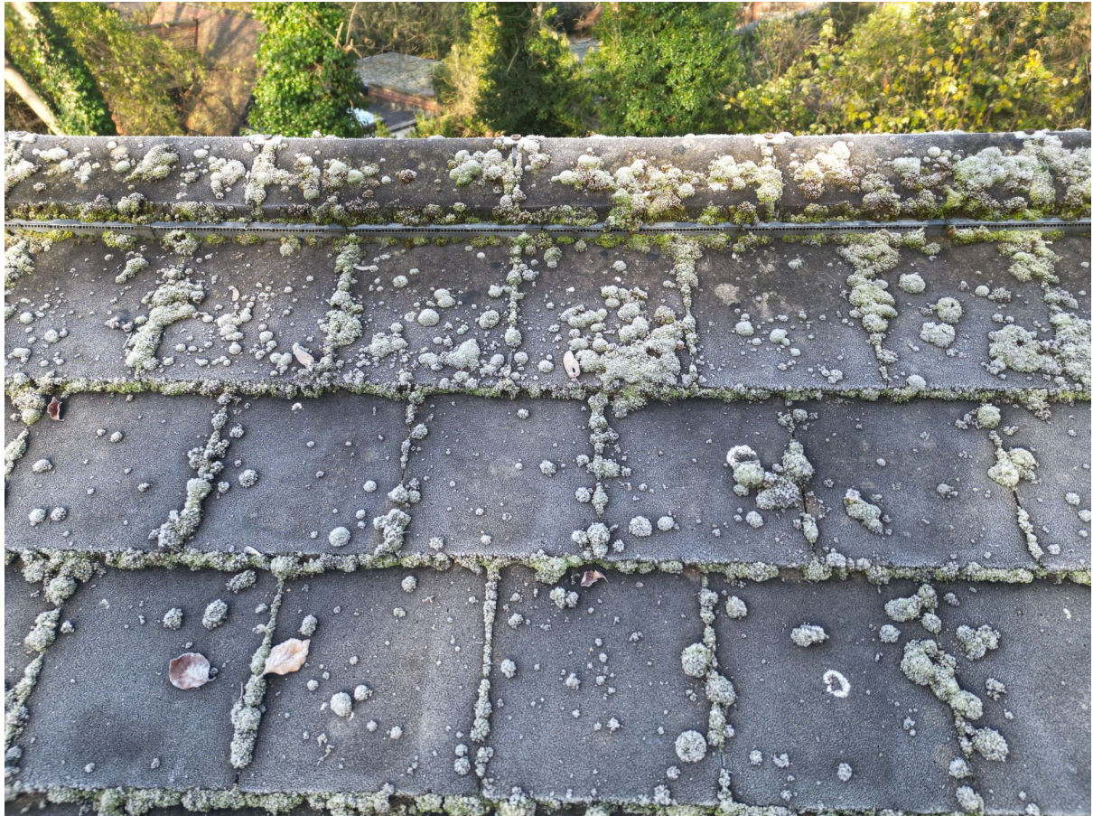
7 – Ridge tiles are mechanically fixed and vented.
