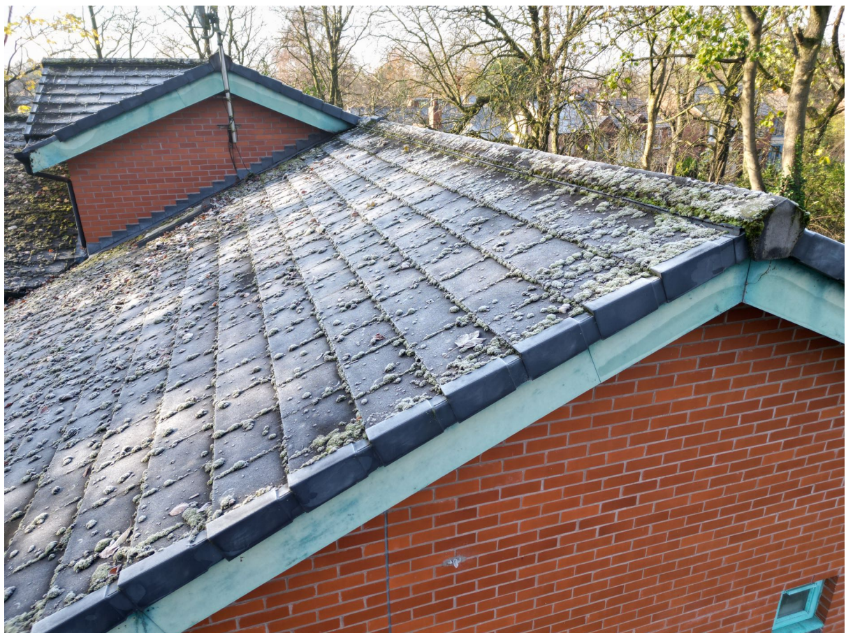
6 – Roof and ridge tiles are in good condition with no viable gaps.
