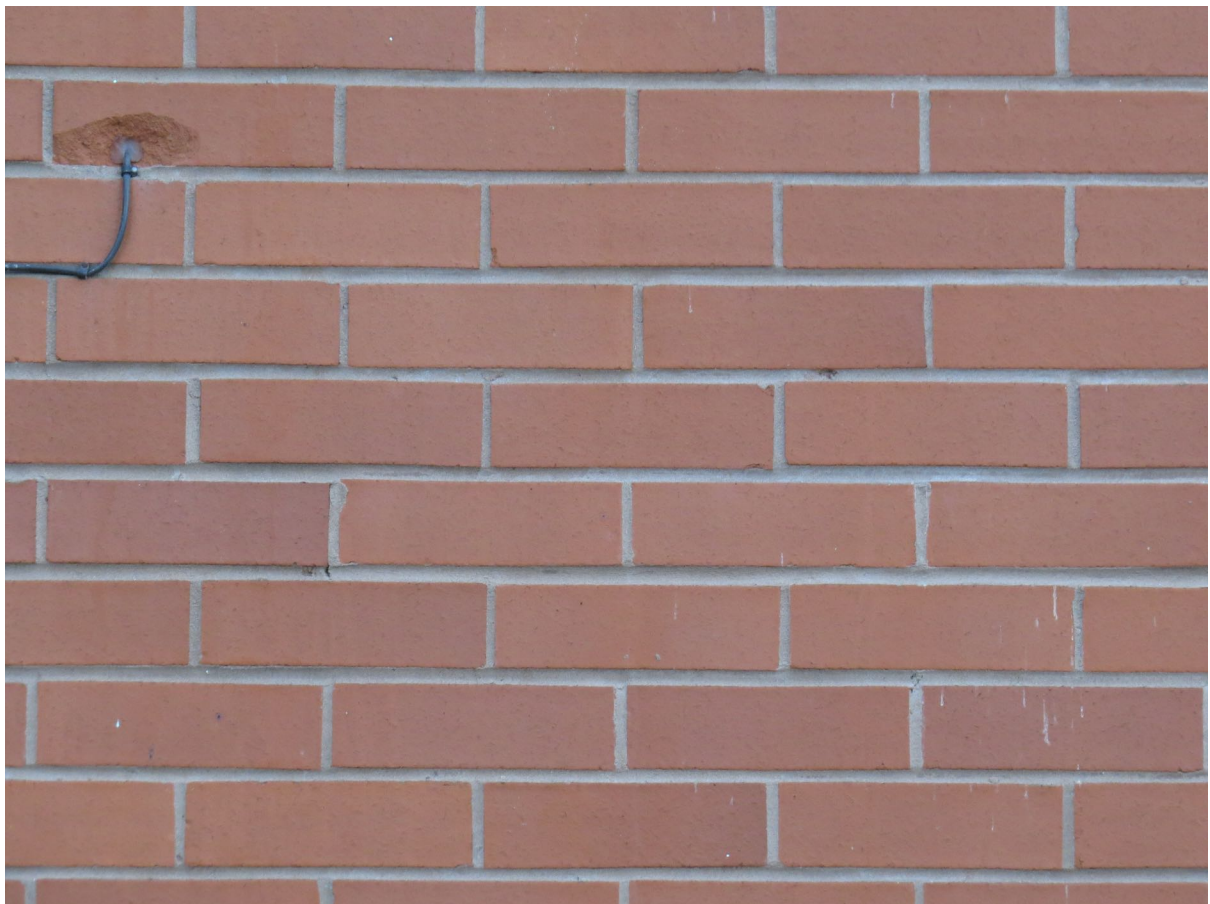
10 – Brickwork is in good condition with no cracks or missing mortar.
