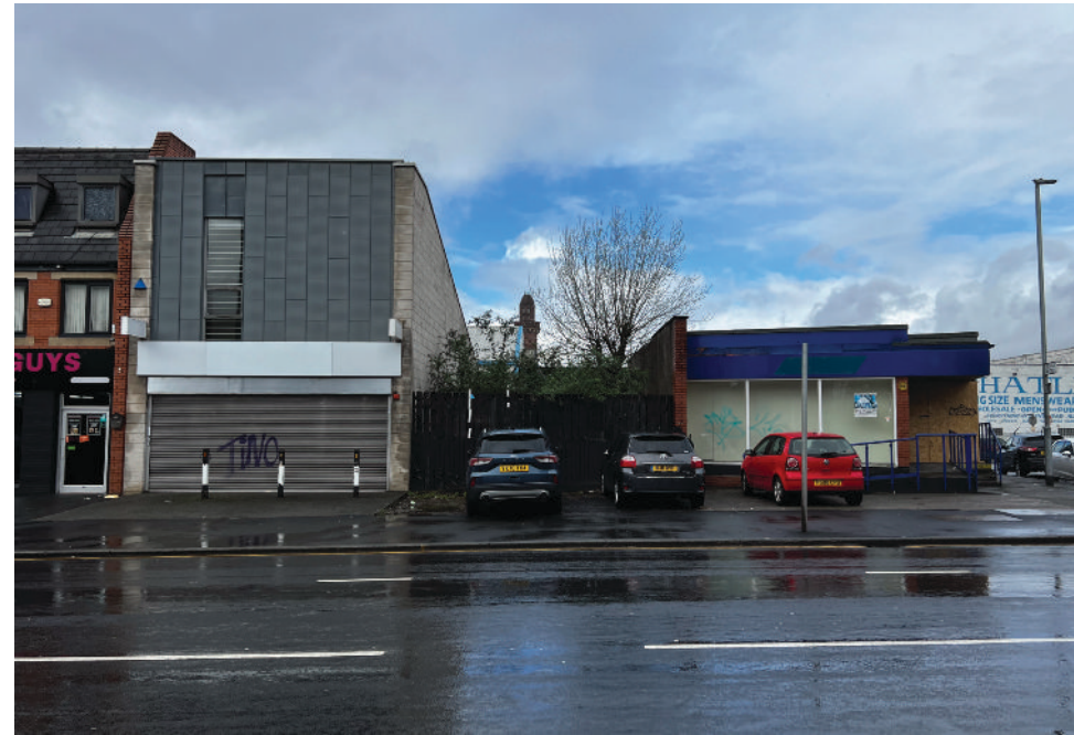
Cheetham Hill road - Site View
