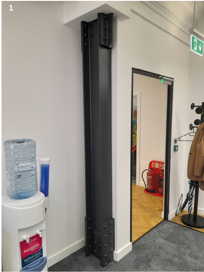
Exposed painted steel column
