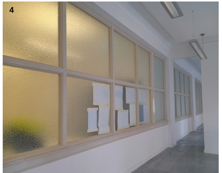
Timber screens and plaster cornices
