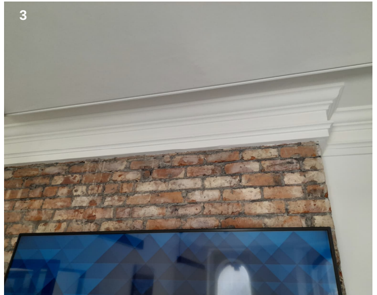
Plaster cornice and exposed brickwork
