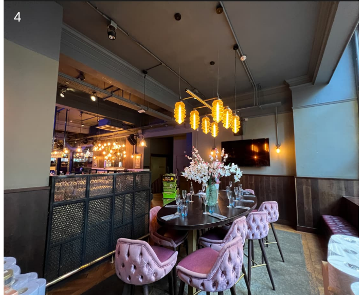
Plaster cornice and ceiling
