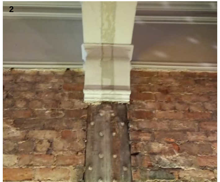
Decorative plaster details to downstands and exposed steel column
