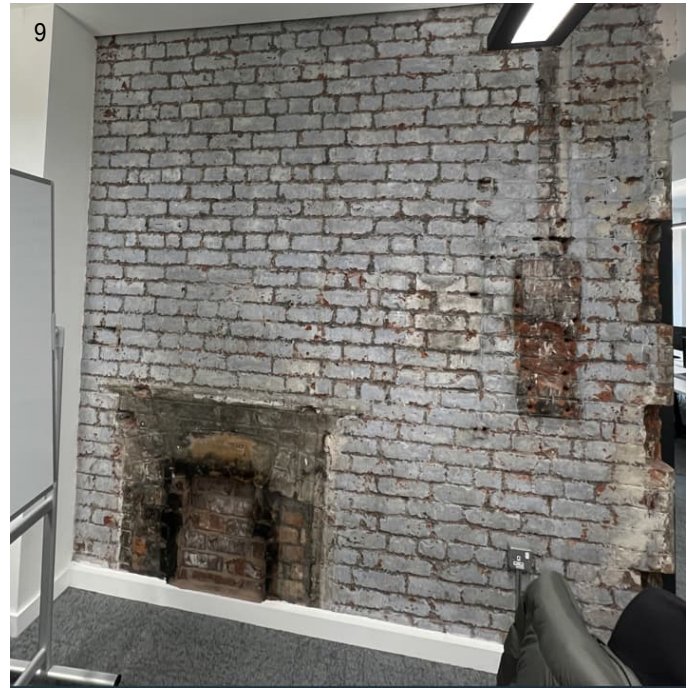
Brickwork with paint removed
