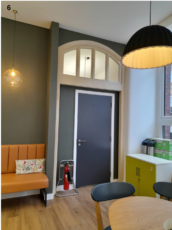
Original fanlight above doorway
