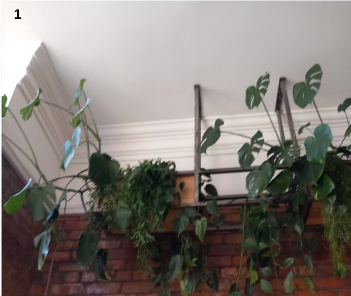
Plaster cornice and exposed brickwork
