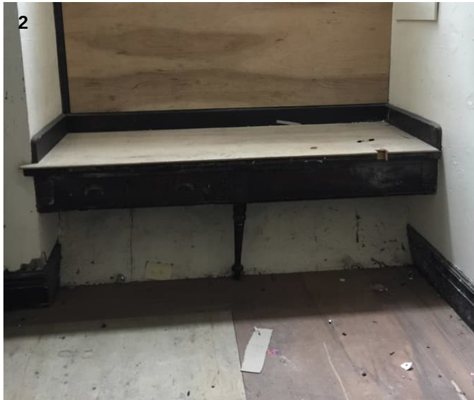
Timber desk built into window reveal ( archive photo )
