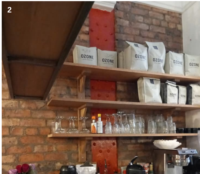
Exposed painted steel columns and decorative details to downstands
