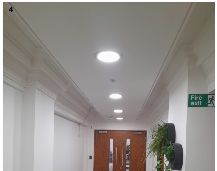
Plaster cornice in corridor
