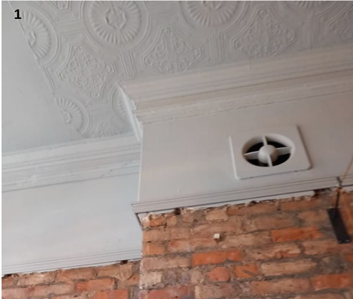
Plaster cornice and exposed brickwork
