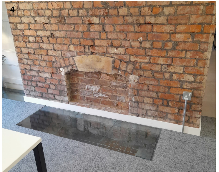
Exposed fireplace and hearth tiles
