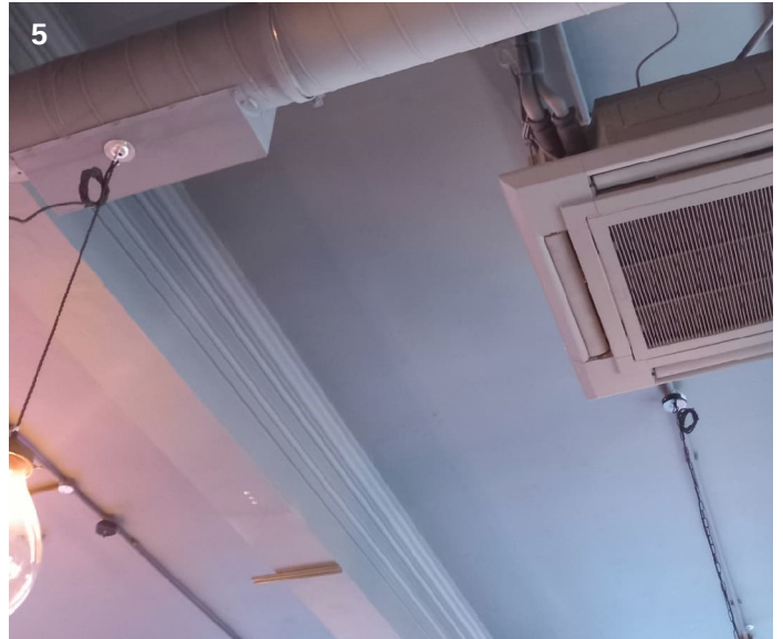
Cornice details to ceiling
