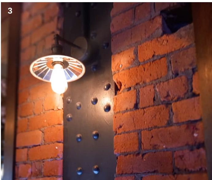
Exposed steel columns
