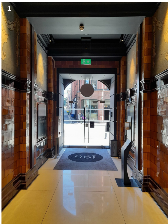
Entrance lobby area from Deansgate, with glazed wall tiles, mosaic tiles and plaster cornice
