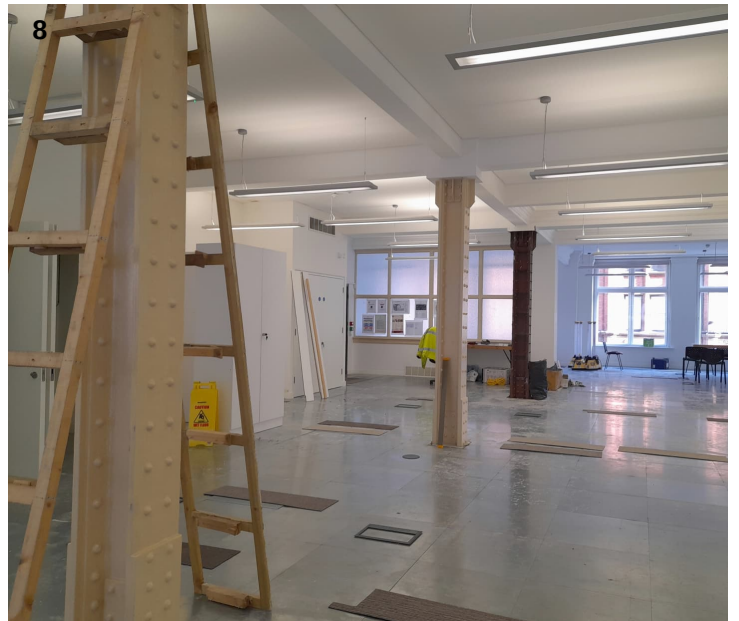
Exposed painted steel columns
