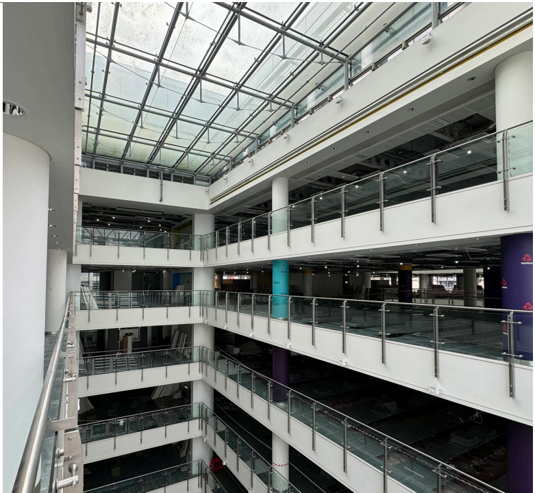
View of Existing Atrium
