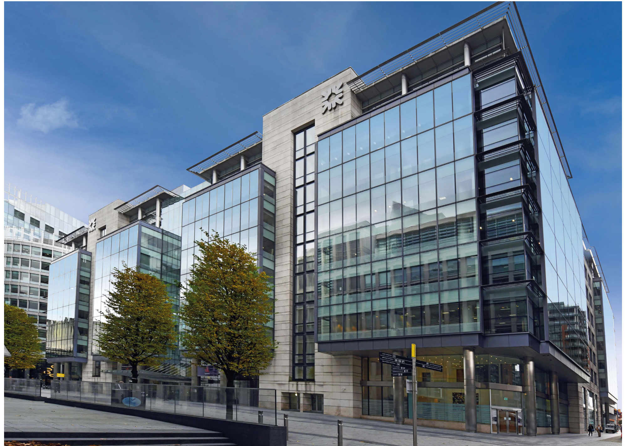
Photograph of existing building from intersection of Hardman Boulevard and Left Bank
