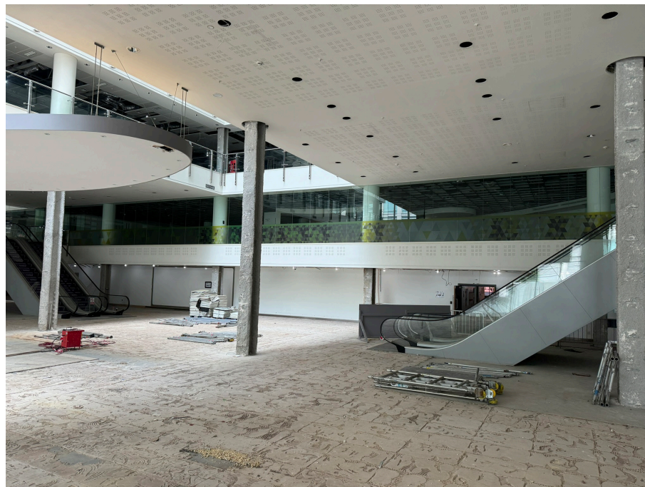
View of Existing Atrium at Ground Floor
