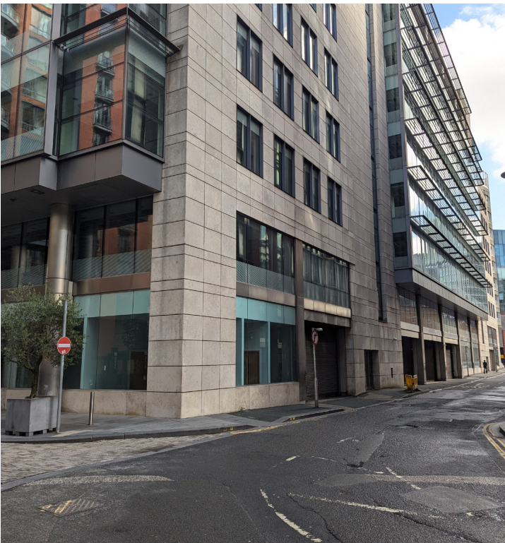
View from corner Left Bank and New College Street
