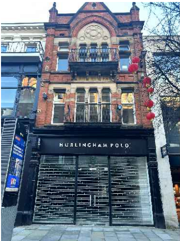
EXISTING STORE FACADE - PHOTOGRAPH
