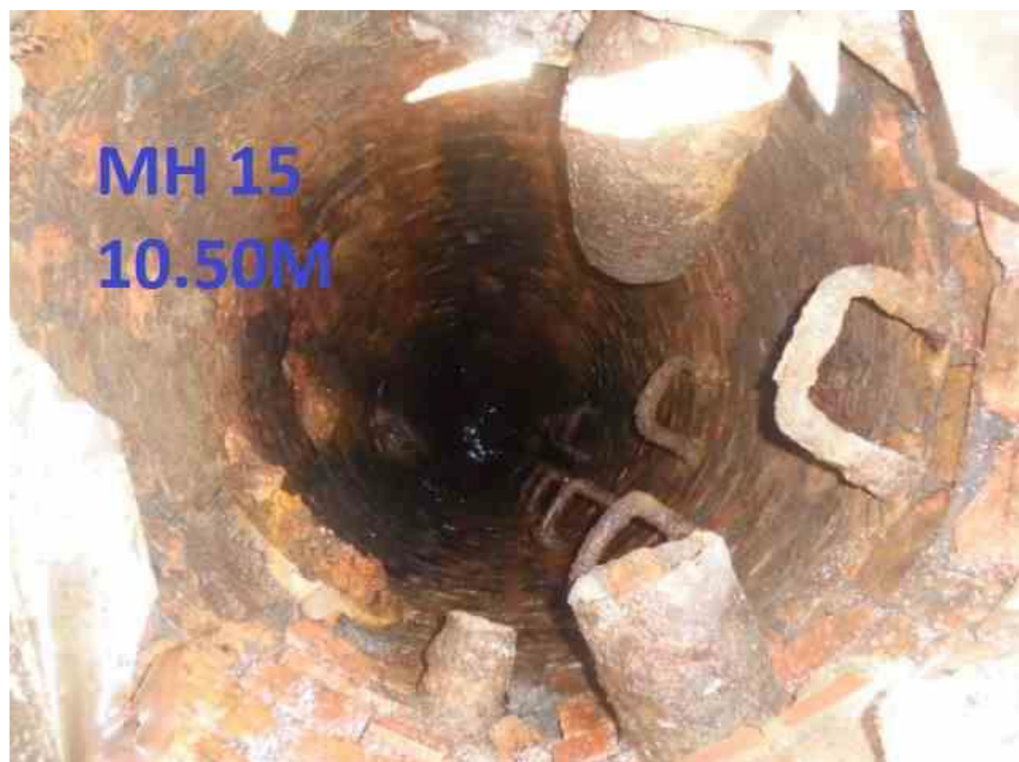
VIEW DOWN MANHOLE 15 FROM SURFACE
