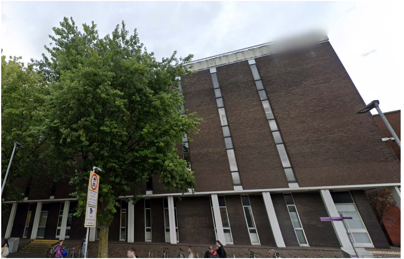
The 2 nd floor windows to which this application relates are obscured by trees
