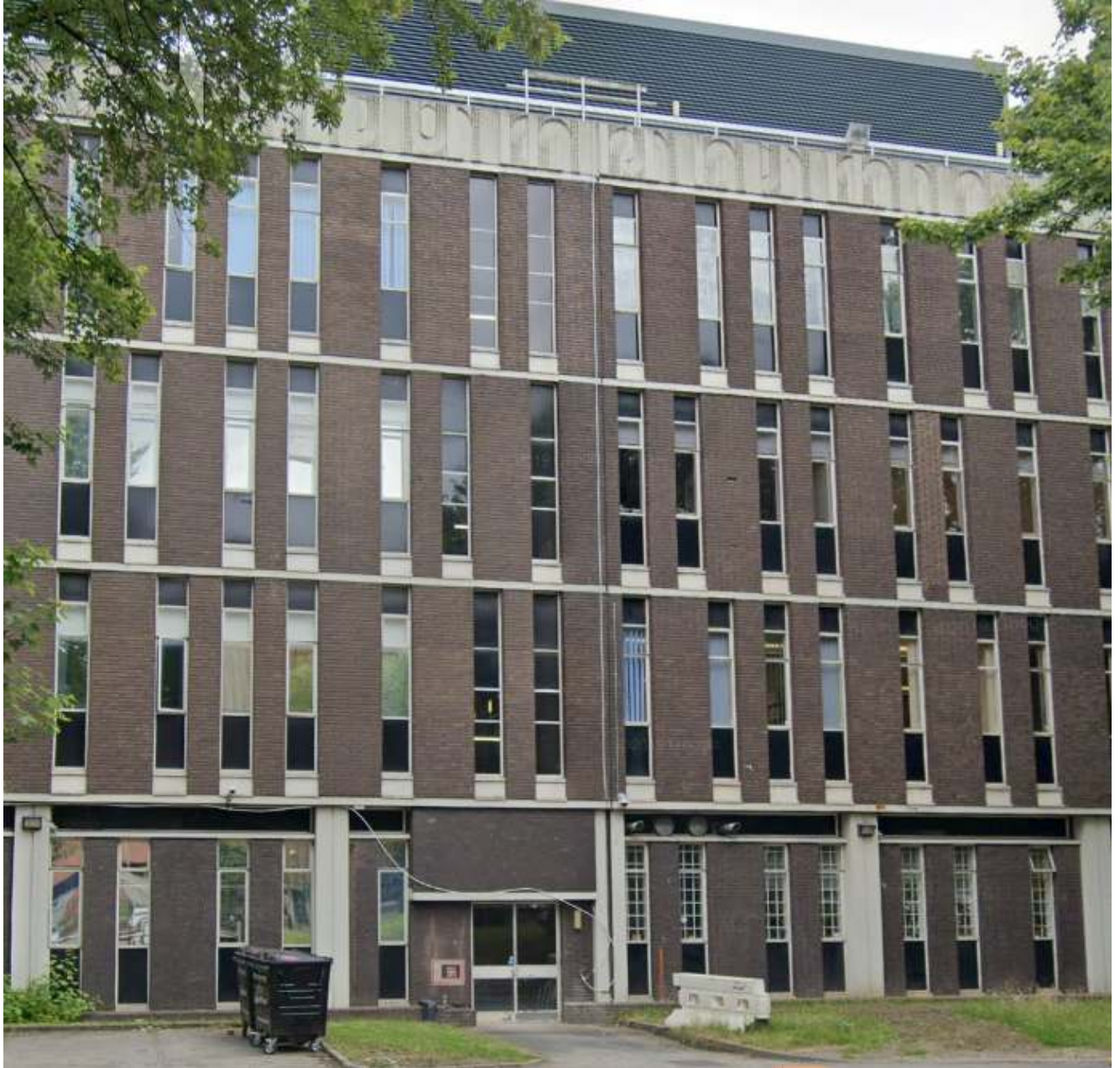
The Stopford Building Grafton Street elevation does not relate to the application but shows the black panel window infills mentioned above.
