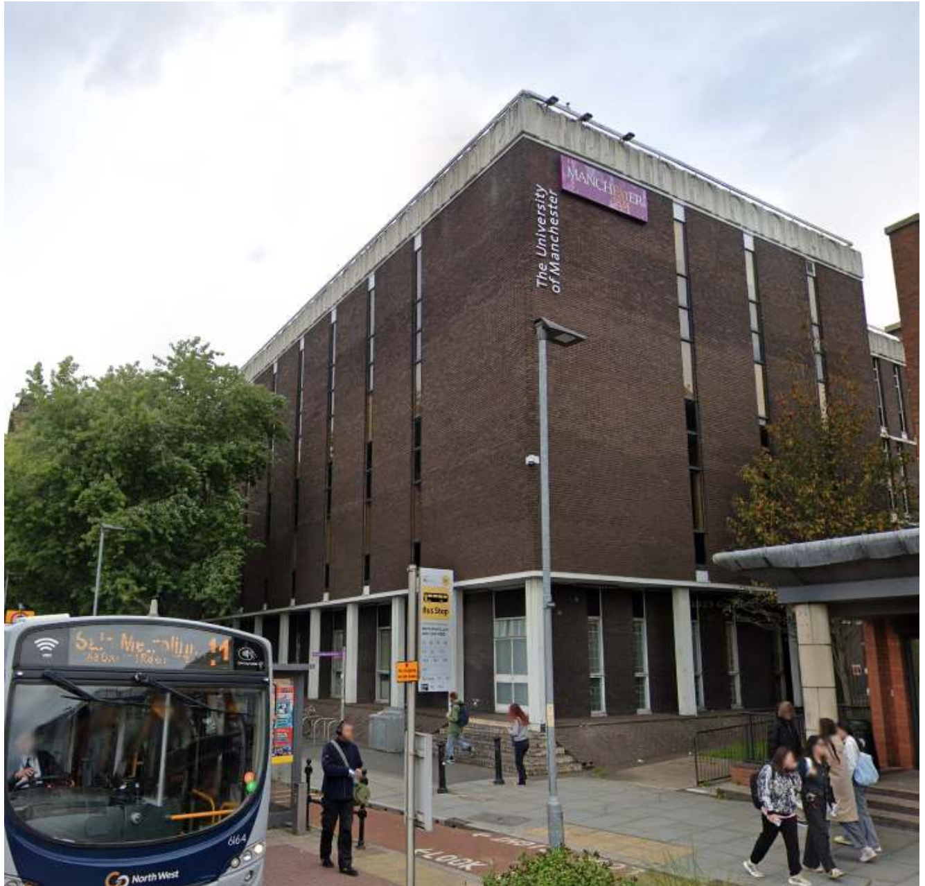
The first 3 windows to the left elevation are unaffected by the works. The 4 th and 5 th can just be seen behind the tree and are affected by the works.
