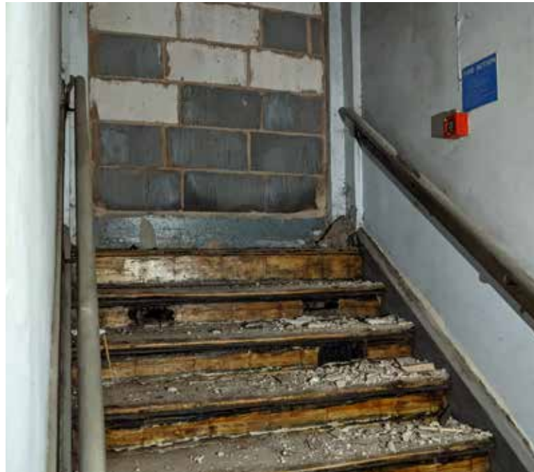
Basement Floor - Page 17 - Image 7
