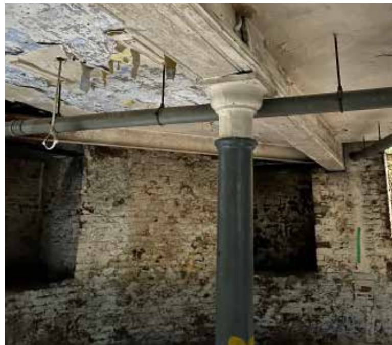
Basement Floor - Page 17 - Image 10
