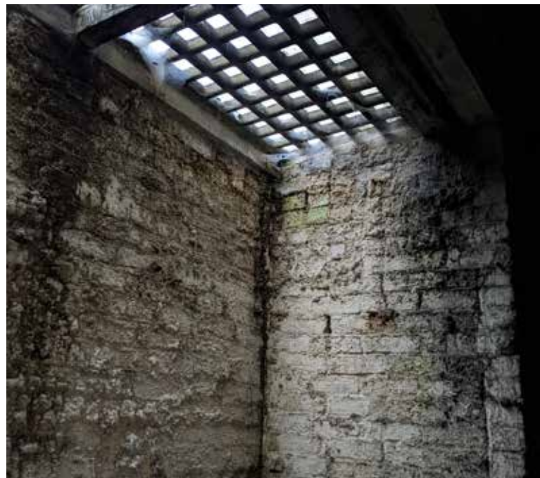
Basement Floor - Page 17 - Image 4
