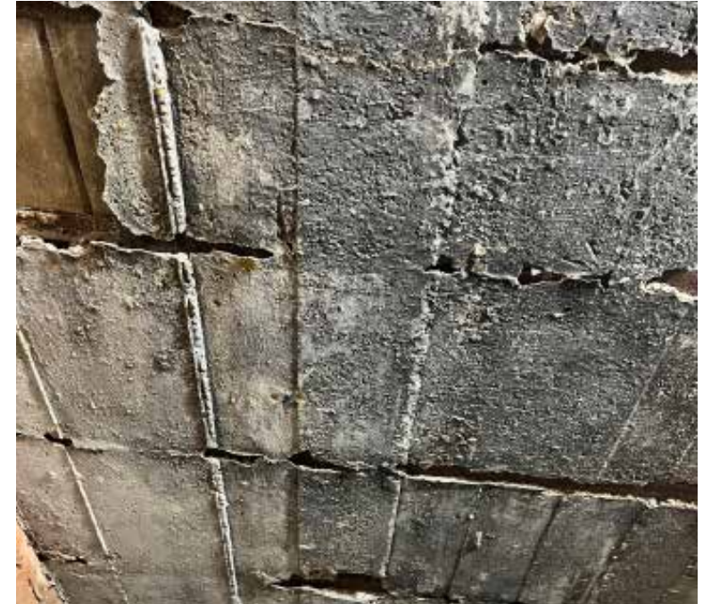
Basement Floor - Page 17 - Image 14
