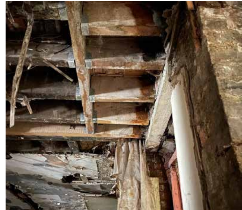
Basement Floor - Page 17 - Image 3
