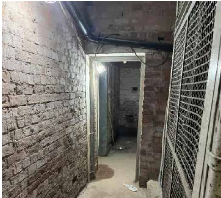
Basement Floor - Page 17 - Image 15
