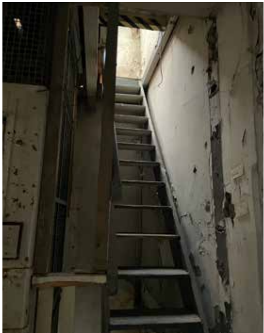
Motor Room – Image 4
