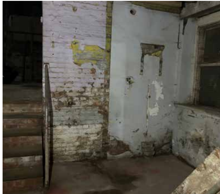
Basement Floor - Page 17 - Image 1
