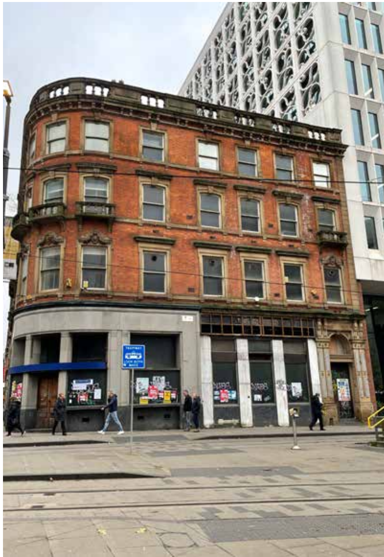
View of Elevation From Mosley Street
