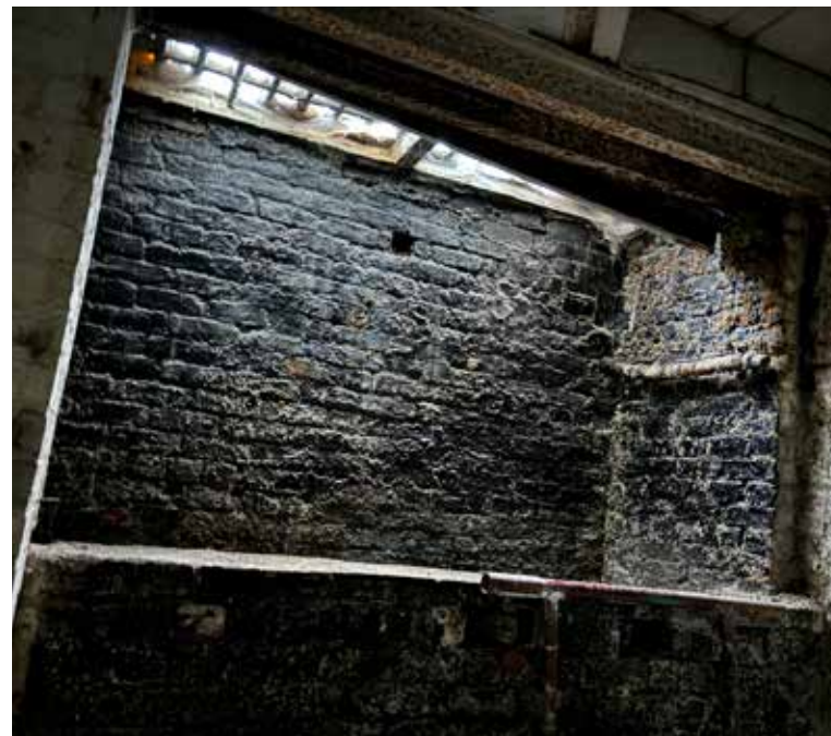
Basement Floor - Page 17 - Image 11
