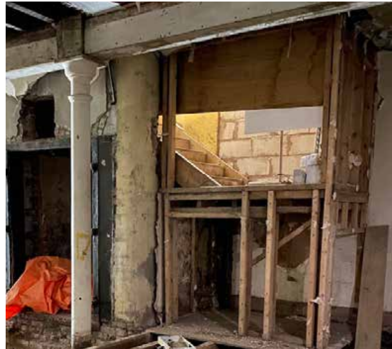
Basement Floor - Page 17 - Image 2
