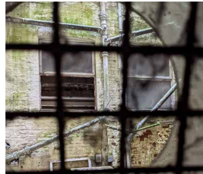
Basement Floor - Page 17- Image 12
