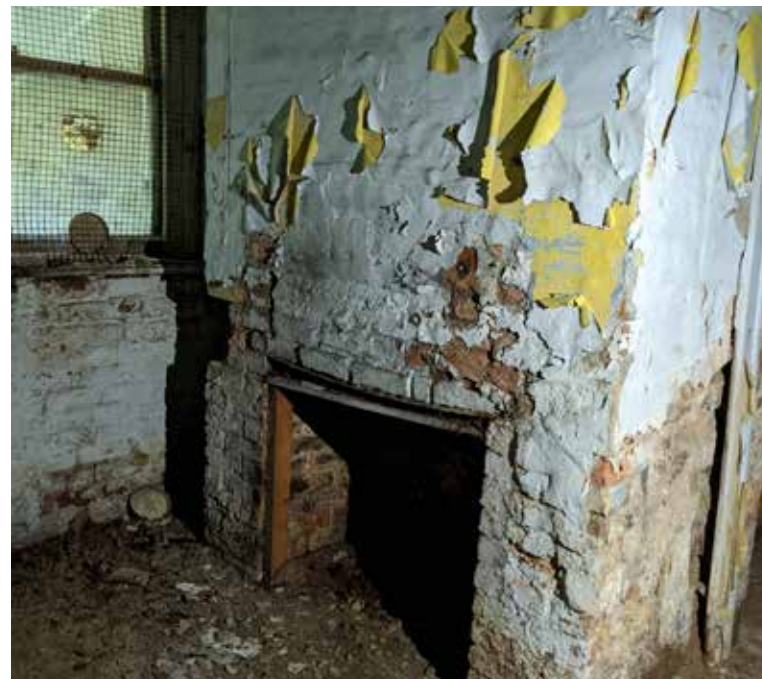
Basement Floor - Page 17 - Image 5
