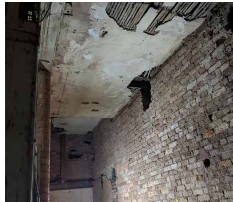
Basement Floor - Page 17 - Image 6
