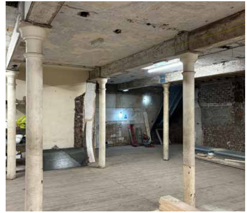
Basement Floor - Page 17 - Image 16
