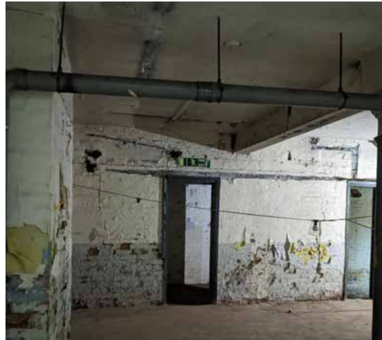
Basement Floor - Page 17- Image 8
