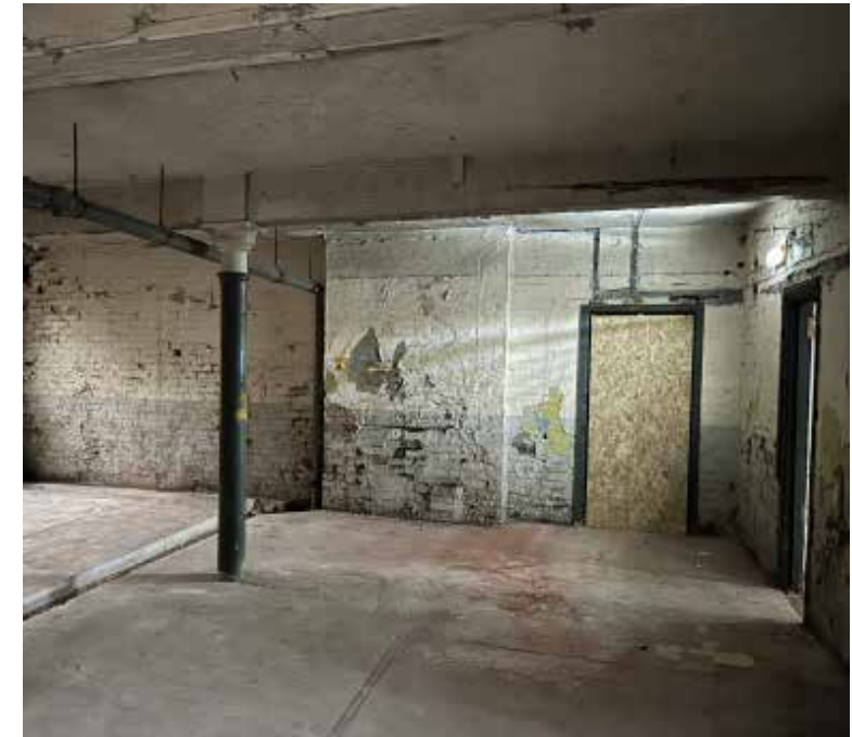
Basement Floor - Page 17 - Image 9
