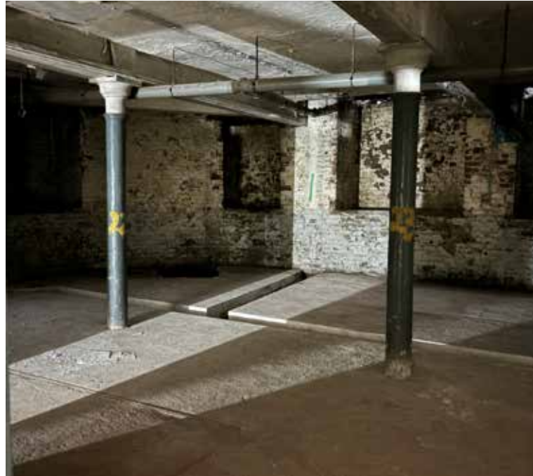
Basement Floor - Page 17 - Image 13
