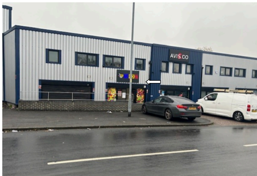
View of application property
