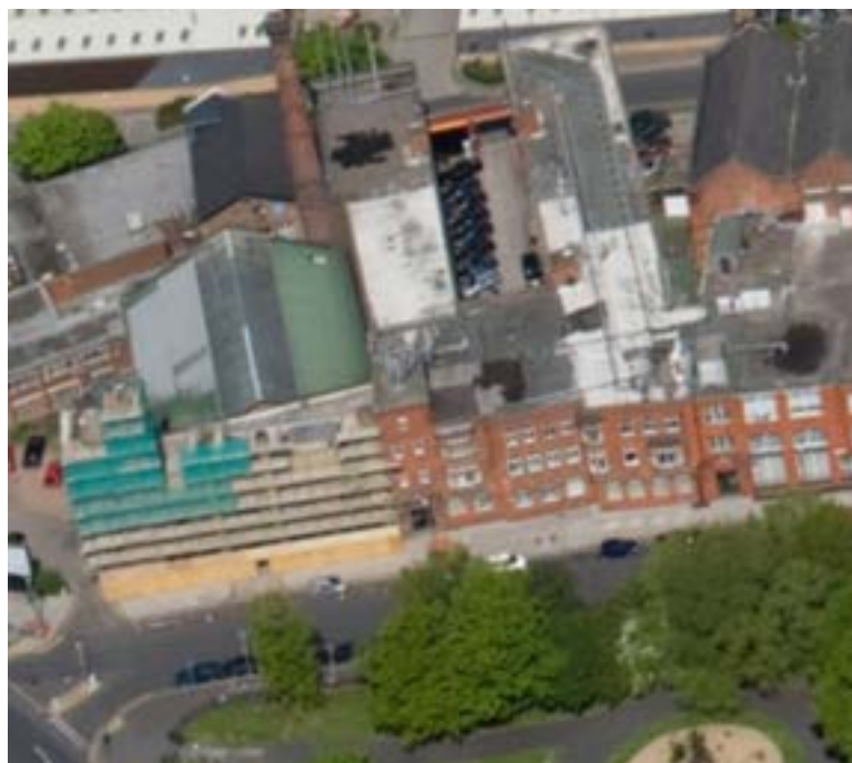
Figure 27: 2008 Aerial Image of Ardwick Drill Hall illustrates the roof is no longer slate, with a new corrugated cladding. Façade repair works appear to be taking place with scaffolding evident to the barracks building. Source: Historic England aerial images.
