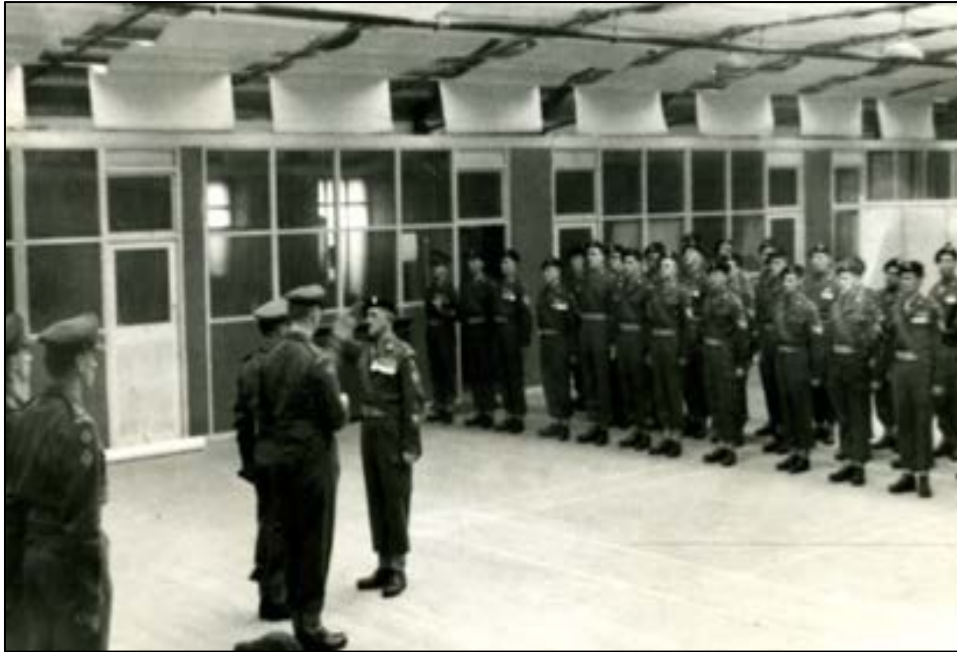
Figure 23: Raised Drill Hall. C1958 within the newly reconstructed/raised drill hall evident. The roof trusses now slightly hidden by temporary material. Source: Manchester Central Archive.
