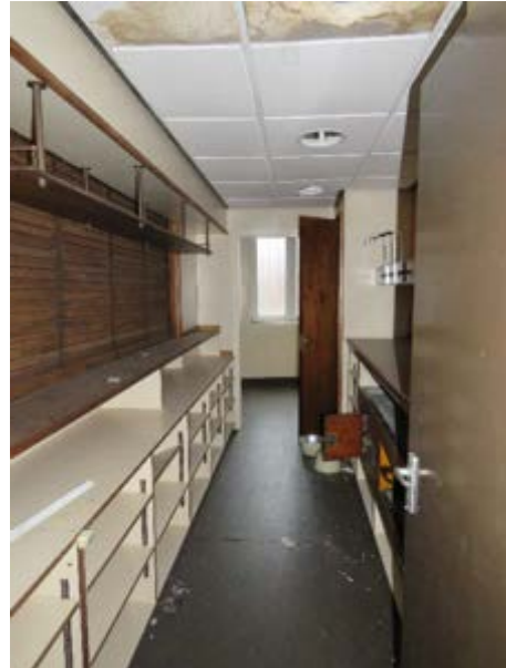
Figure 33: Second Floor to principal building. 1980s bar and stud wall, east aspect.
