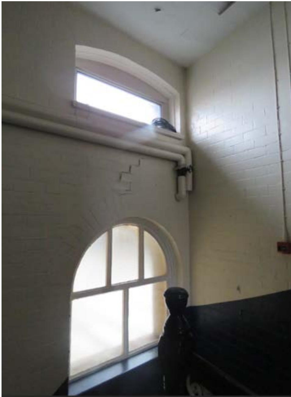
Figure 36: High level window opening to stairwell (upvc infill, no significance ). Original walls and window openings are of high significance .
