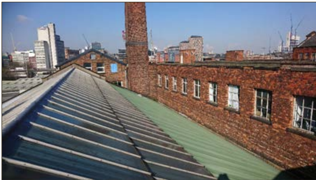
Figure 34: Skylight over Drill Hall (NE aspect). Glazing, glazing bars and corrugated sheeting are of no heritage significance .
