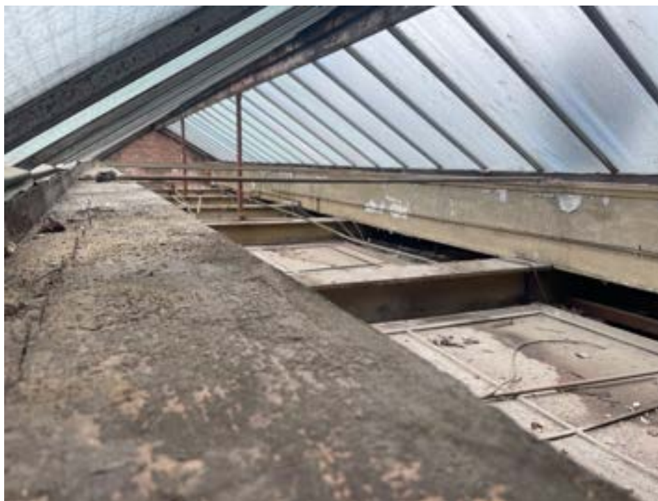
Figure 30: Skylight over principal building, glazing and glazing bars are a later addition (c.late 20 th century). Suspended ceiling to second floor blocks light coming through into the building, this false ceiling is also a late-20 th century addition and is of no heritage significance .
