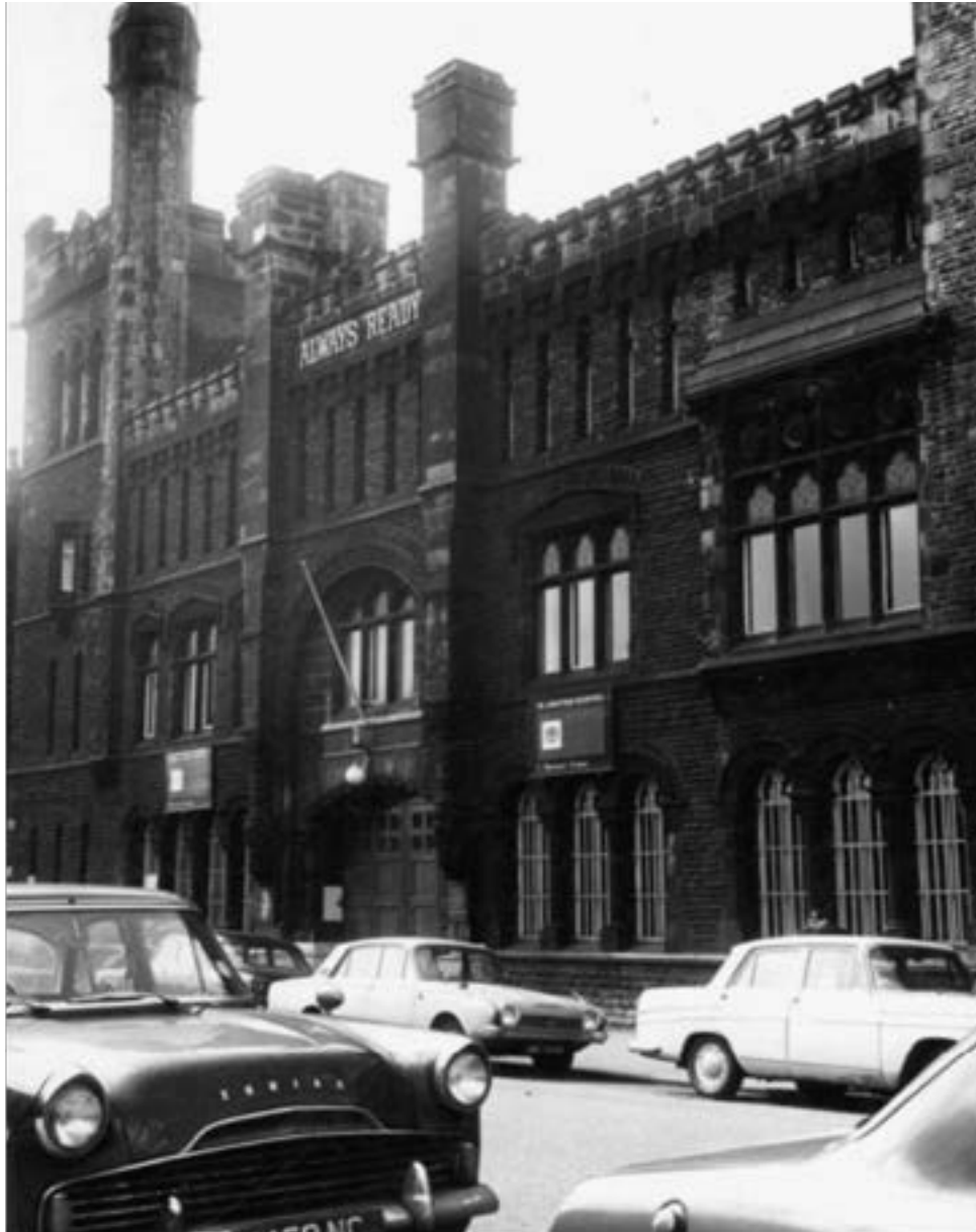
Figure 24: Historic Image of Ardwick Green Drill Hall, pictured 1969. Note the original door is still extant. Source: Manchester Central Archive. ref: m10817.
