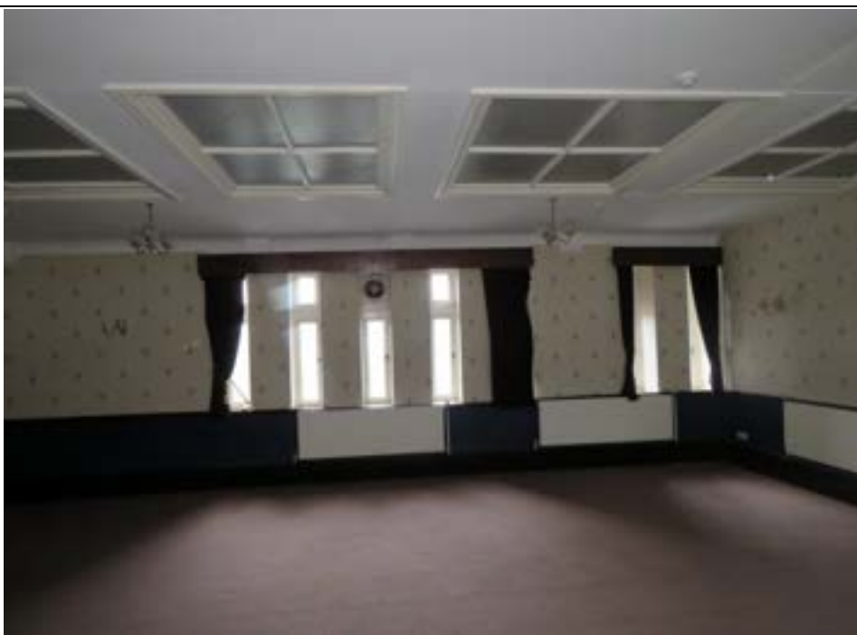
Figure 31: Second Floor to principal building. Suspended ceiling to second floor blocks light coming through into the building, the ceiling is presumed to be mid-late-20 th century addition with the extent of original fabric above unknown (subject to intrusive investigation works).
