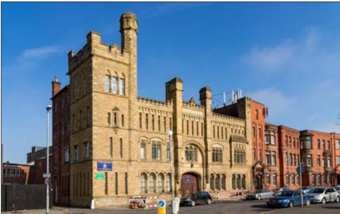
Figure 1: Photo of the Subject Site, 'Drill Hall at Ardwick Green North'. Source: SLHA 2024
