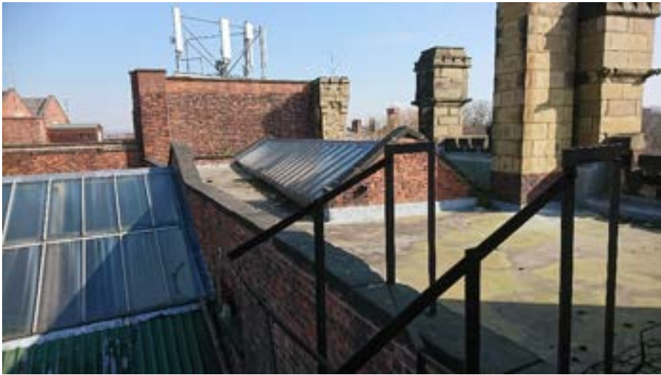
Figure 29: Flat roof to principal building, original form of the skylight and chimneys feature. Glazing and glazing bars are a later addition (c.late 20 th century / early 21 st century) and are of no heritage significance.
