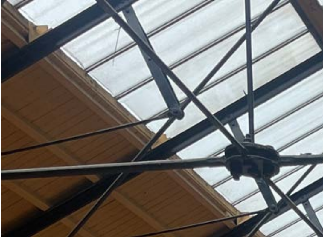
Figure 38: Close range view of Drill Hall roof, illustrating original late-19 th century wrought iron truss arrangement and timber batons / purlins. Glazing and glazing bars all late-20 th c.
