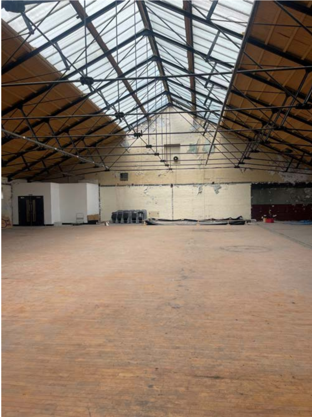
Figure 37: Drill Hall interior, looking north across the space. The 1930s raised floor has altered the original double height space ( medium significance ). Original late-19 th century trusses, purlins and timber batons survive – high significance . Glazing and glazing bars appear to be late-20 th century, following inspections from roof level ( no significance ).
