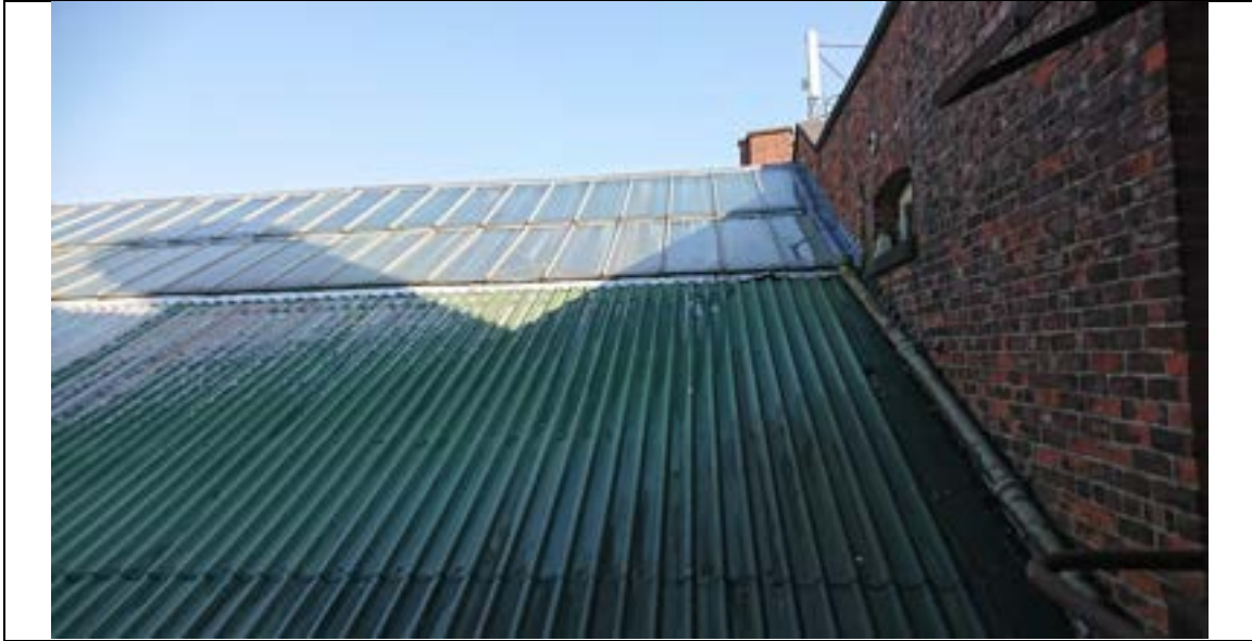
Figure 35: Skylight over Drill Hall (SW aspect). Note, window to the north-west elevation of the barracks building is proposed to be blocked up as part of the proposals (window infill is upvc and of no significance ). Original gable wall is of high significance .
