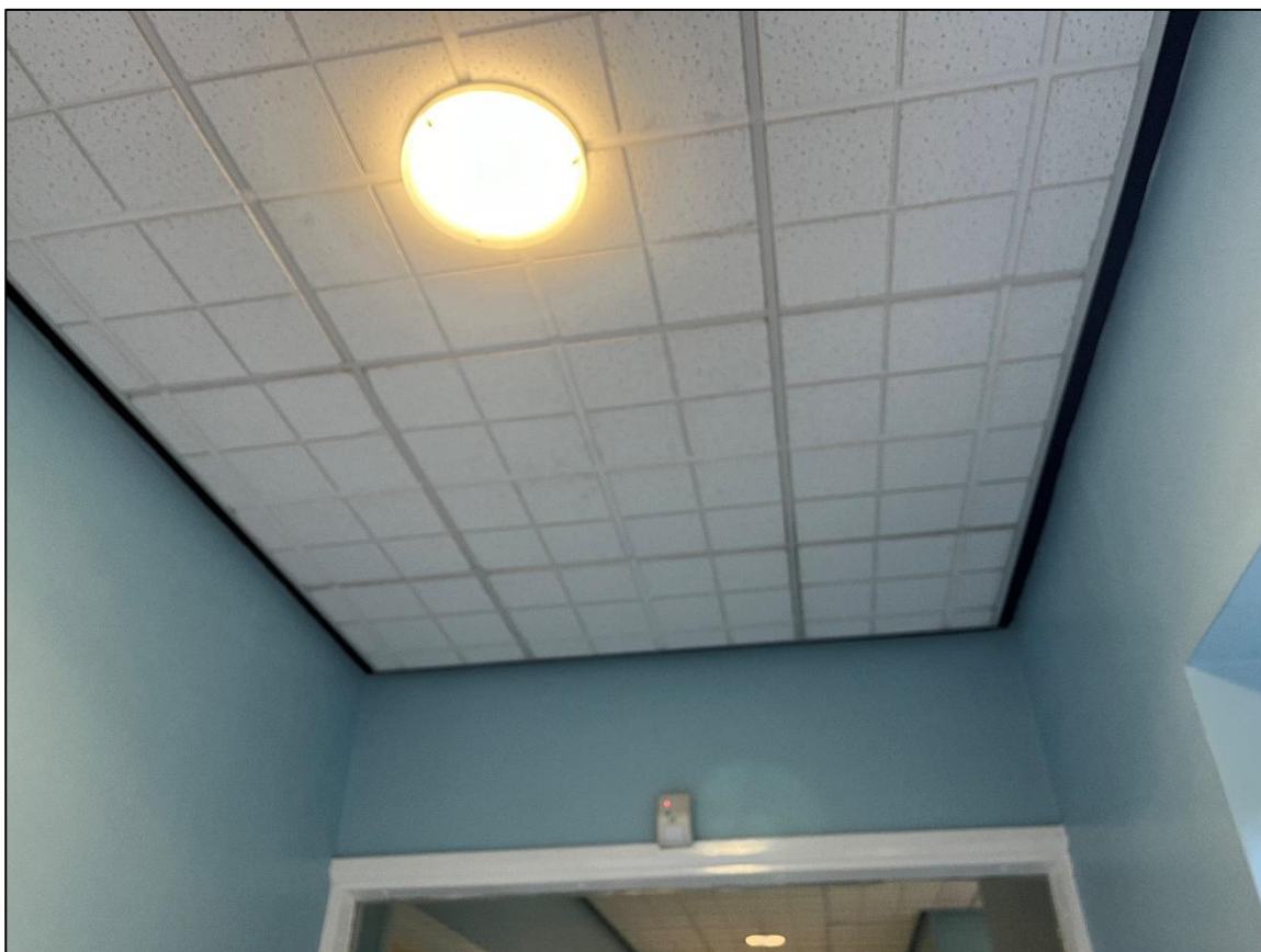
Plate 7 – Character of false ceilings within pitched areas of the building
