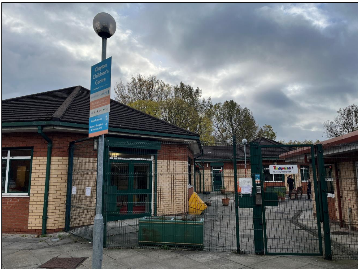
Plate 4 – Western aspect of the structure
