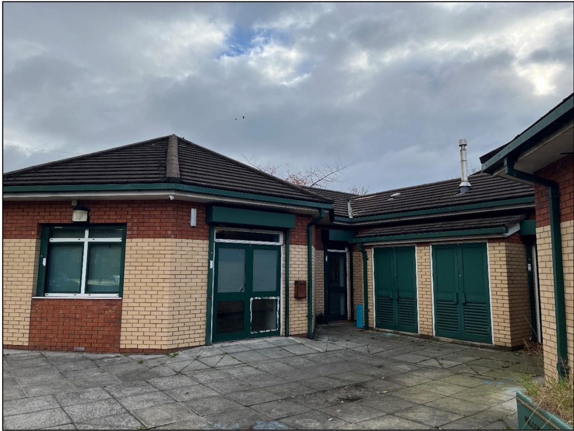
Plate 1 – The Wells Centre as seen from the north, where ASHP will be placed
