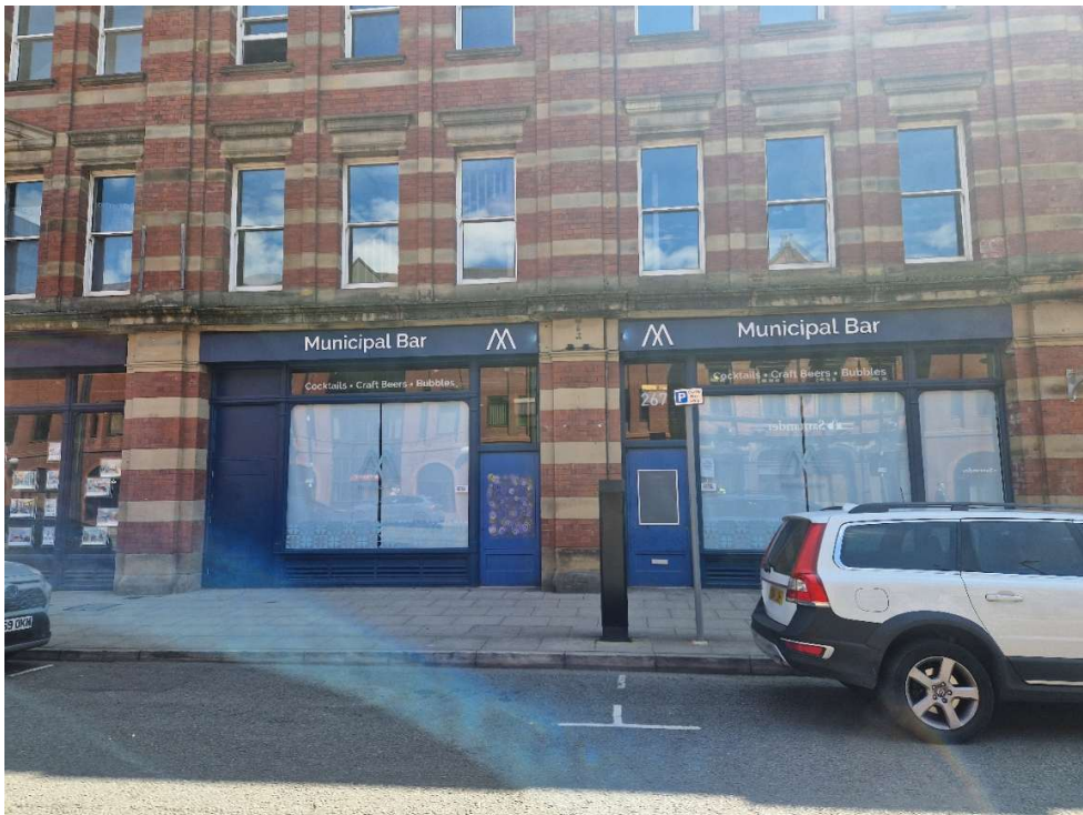
Image 4: Present Shopfront Elevation, Deansgate, Manchester
