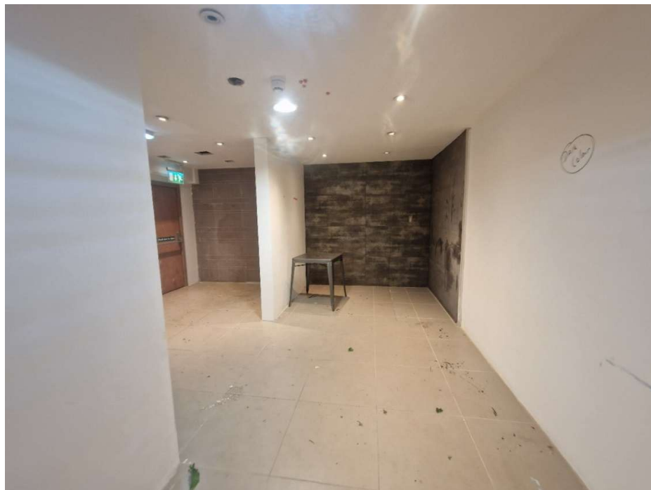
Image 12: Present Ground Floor Interior view, rear of unit 265
