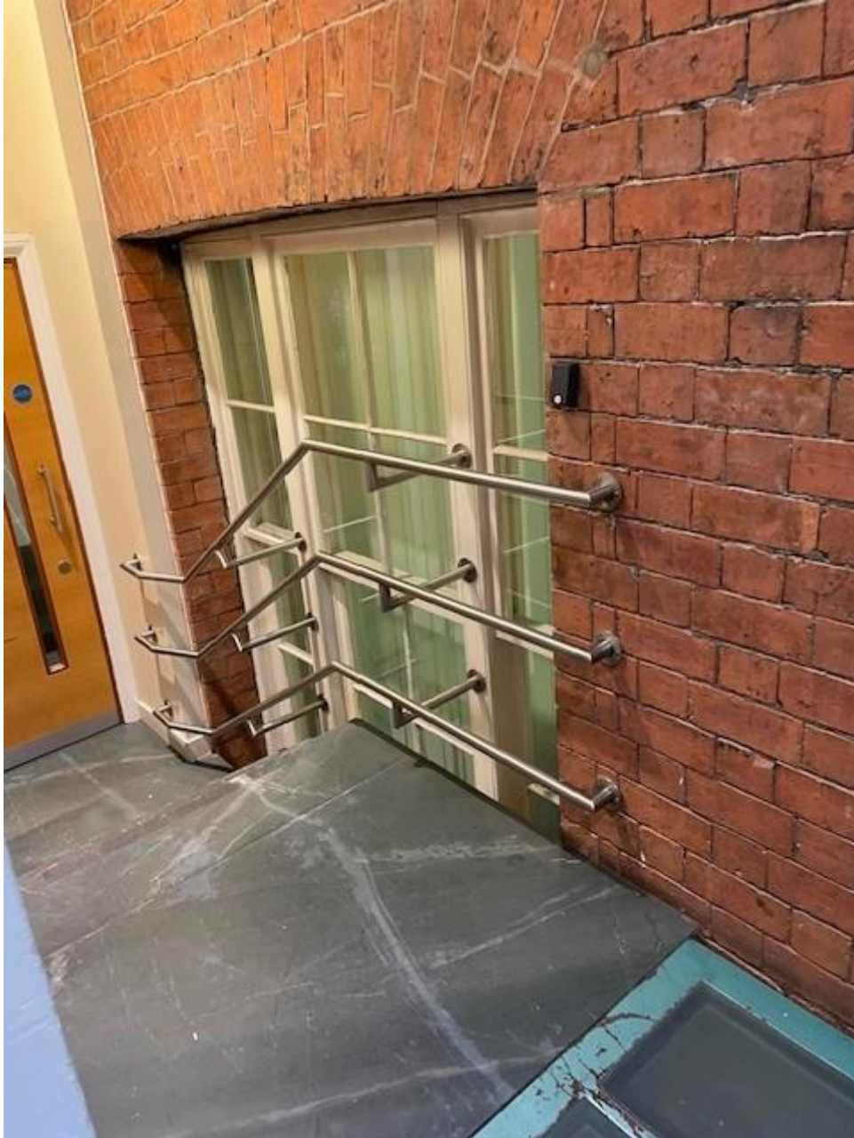
Window 1 (External Before 1995 Refurbishment).
