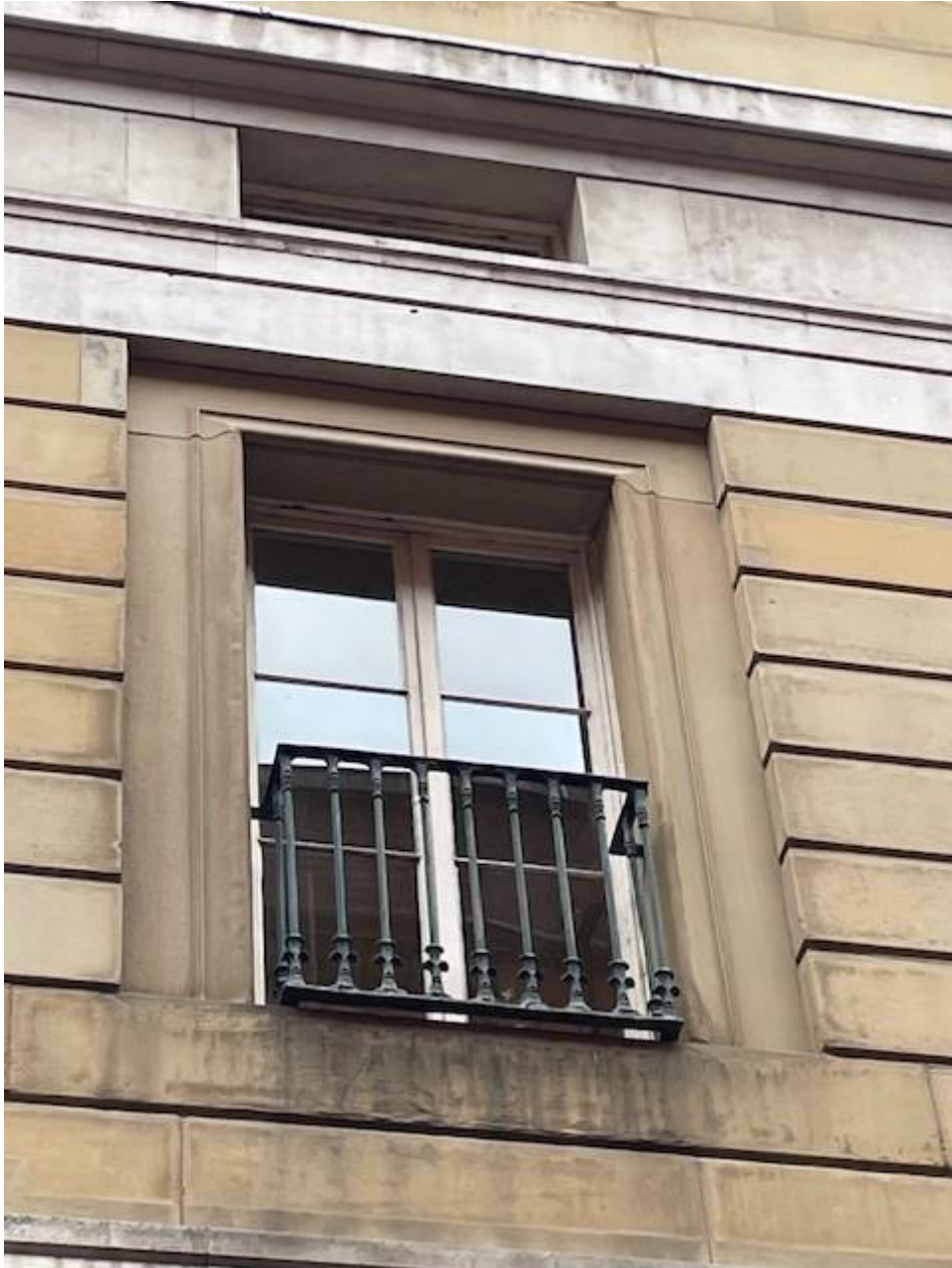
Essex Street Balcony Doors (External)
