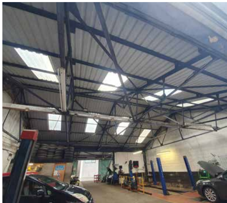
Image: Existing interior with rooflights.
