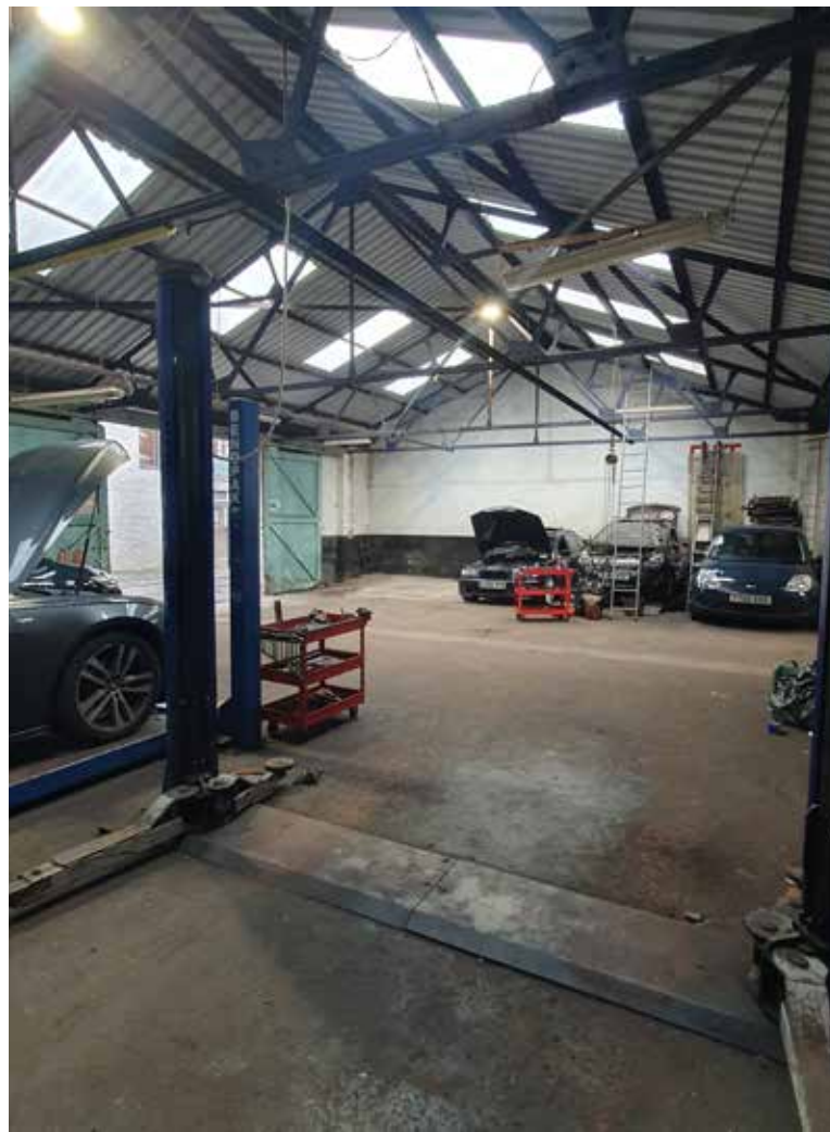
Image: Existing view of garage interior.
