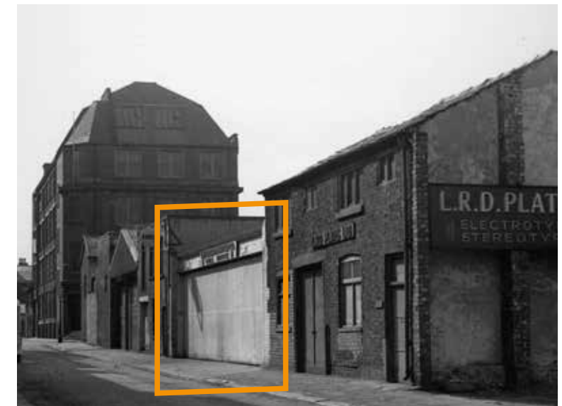
Image: Photograph of Henry Street, 1962, from Manchester Archives, with signage for garage and timber doors evident.
