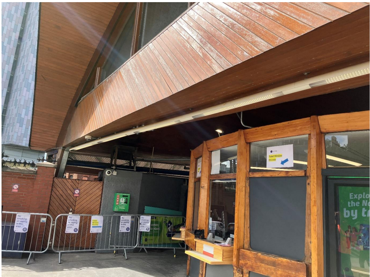
Figure 5 - View of station exterior, second ticket desk is not visible from this angle
