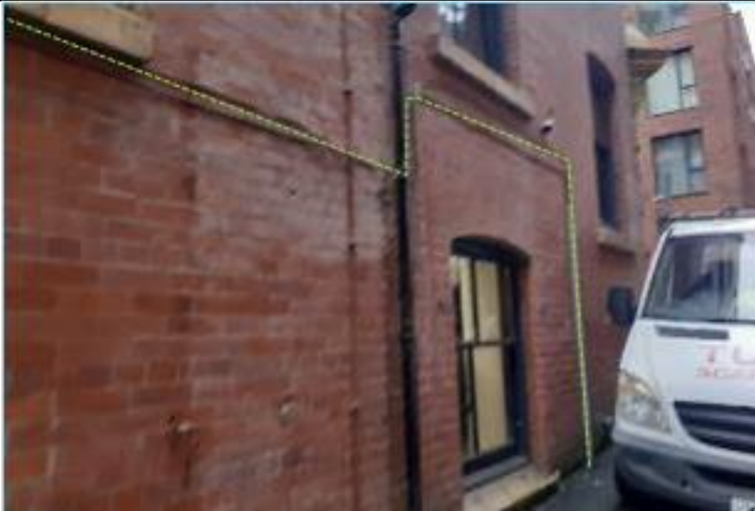
Photo 4: Route of cable following existing cables to the lower ground bin store
