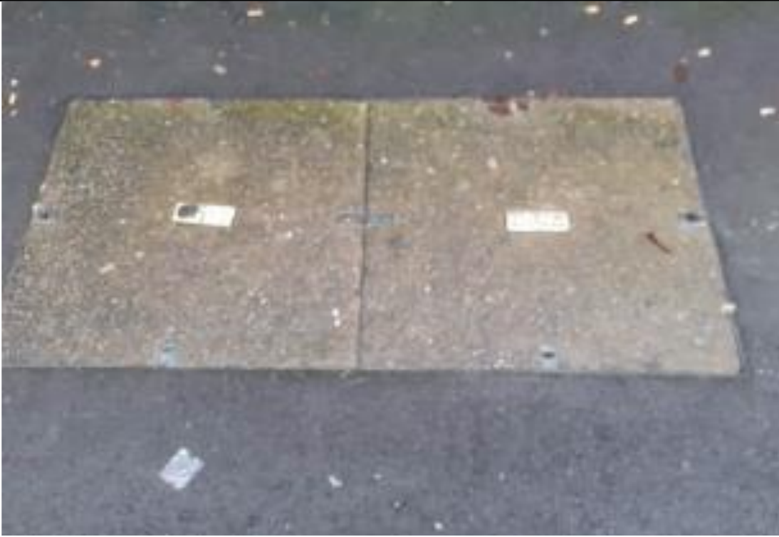
Photo 1: From chamber on New Mount St to apartments
