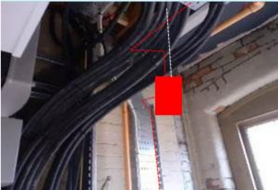
Photo 7: Discreet cabling going through ceiling using existing cable routes
