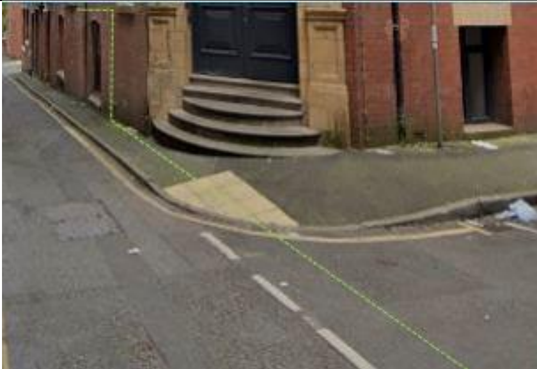
Photo 2: Cable running underground on Ludgate Street
