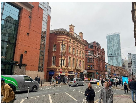
Figure 2.2 – The site building within its wider context along Deansgate
