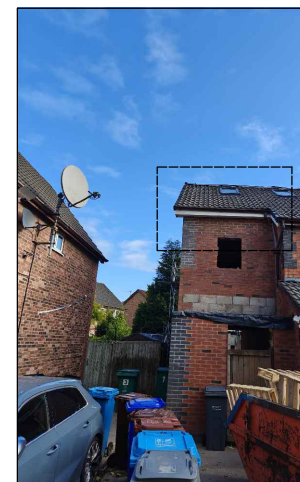
Existing roof building error
