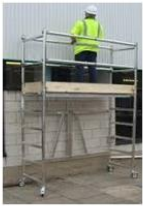
Low-level Access tower <2.5metres
