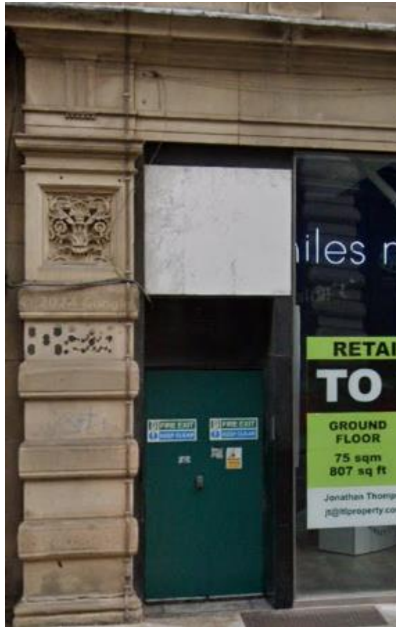
Marble section above fire door
