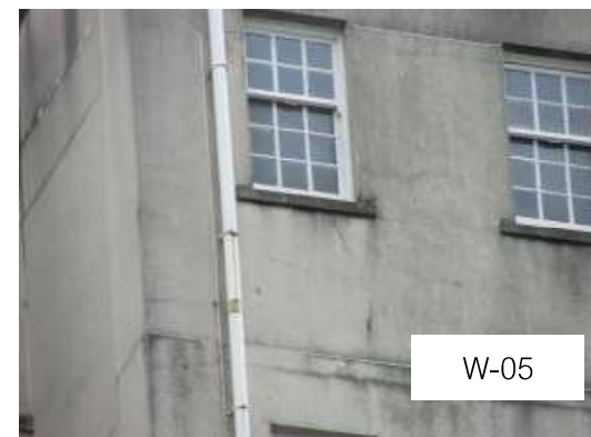
Common typical defect photographs; missing pointing, staining, hairline cracks to rendered facades
