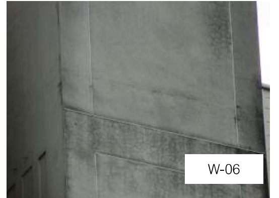
Common typical defect photographs; missing pointing, staining, hairline cracks to rendered facades
