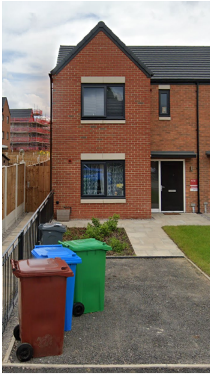
Figure. Front elevation (photo dated July 2019)
