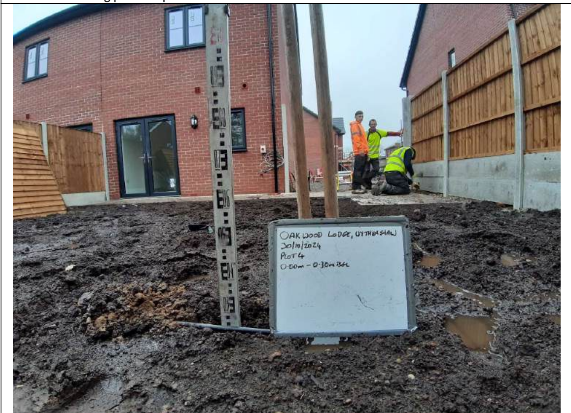
Photo 6 – Showing plot 4 depth validation to 0.30m.
