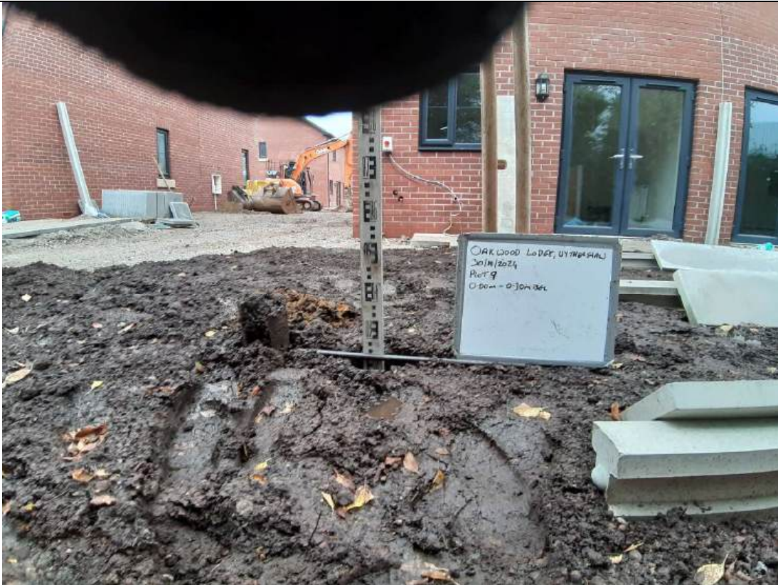
Photo 16 – Showing plot 9 depth validation to 0.30m
