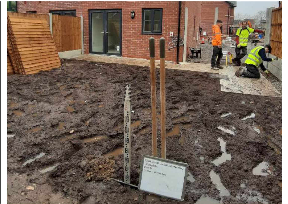
Photo 5 – Showing plot 4 depth validation to 0.30m.
