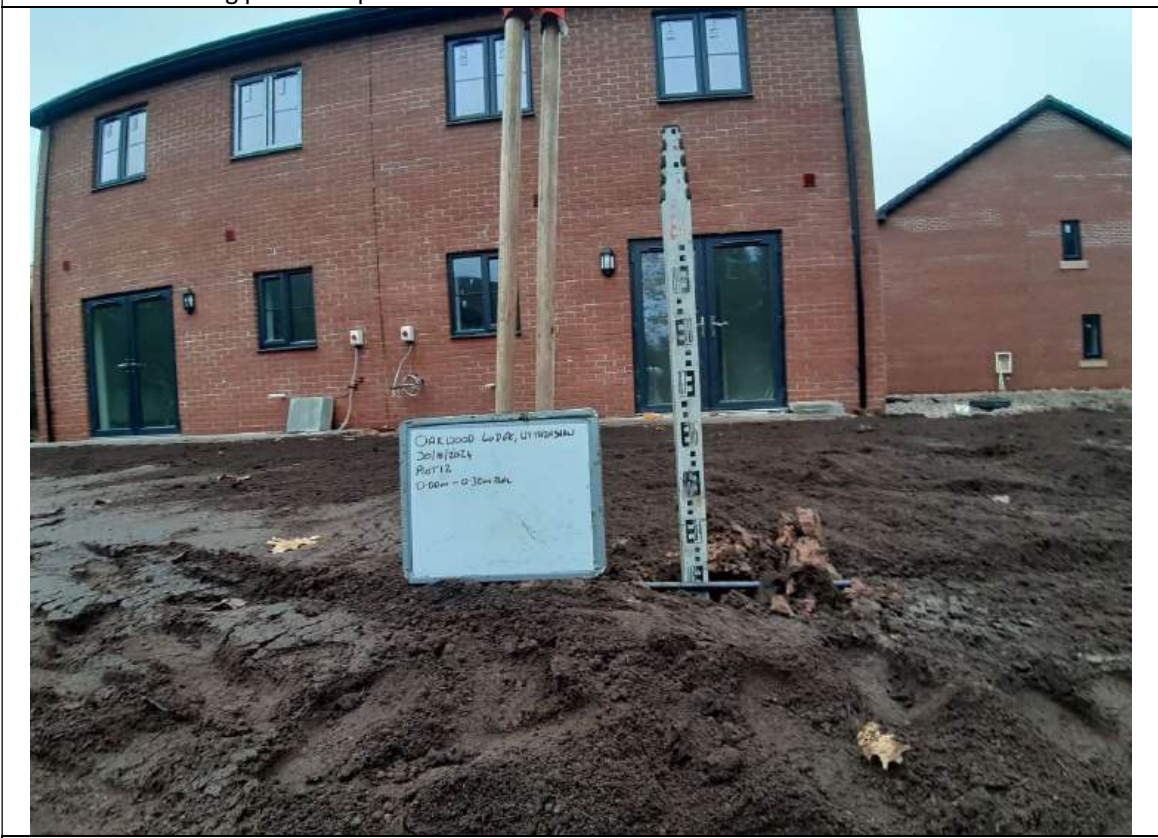
Photo 22 – Showing plot 12 depth validation to 0.30m.
