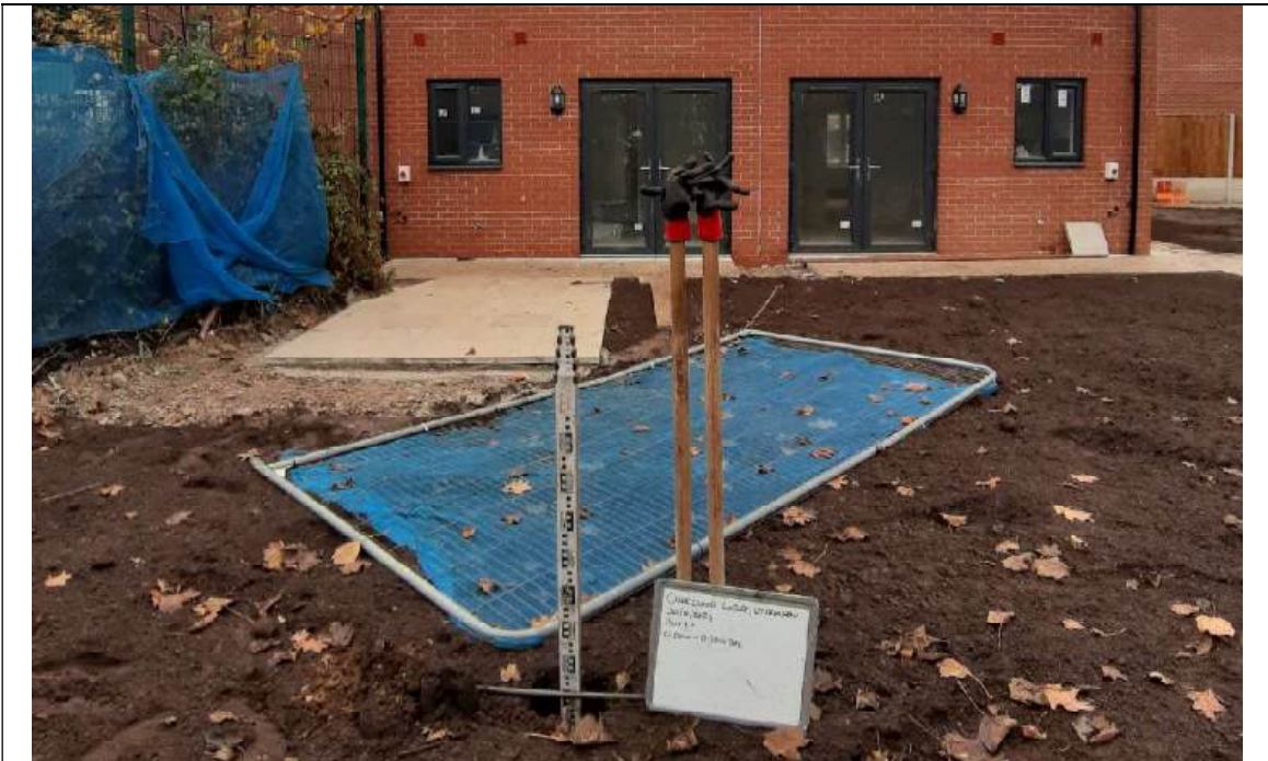
Photo 23 – Showing plot 13 depth validation to 0.30m
