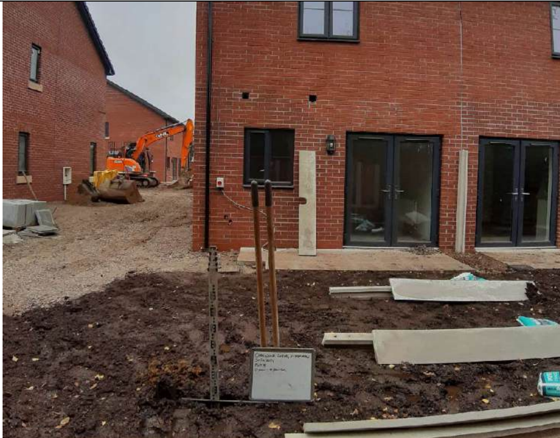
Photo 15 – Showing plot 9 depth validation to 0.30m.
