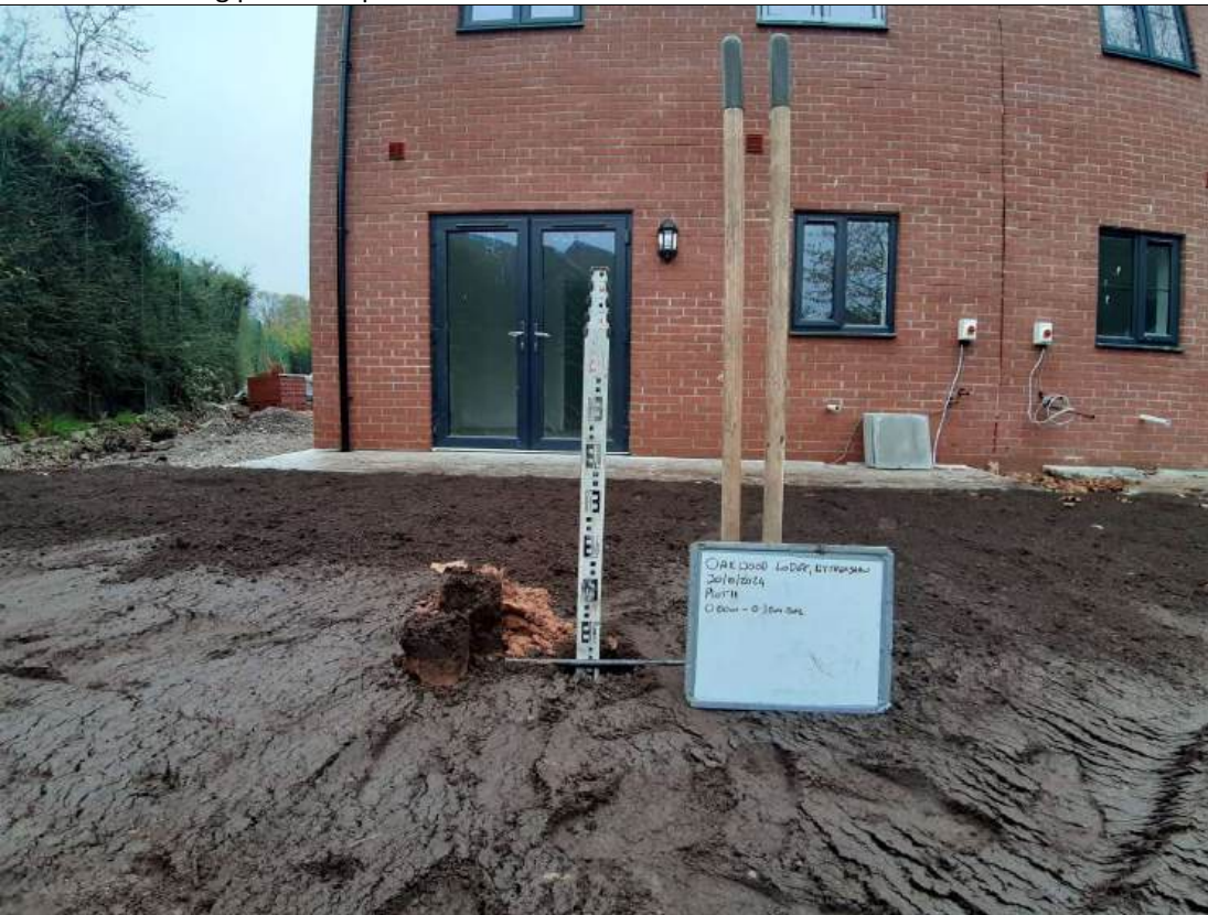
Photo 20 – Showing plot 11 depth validation to 0.30m.
