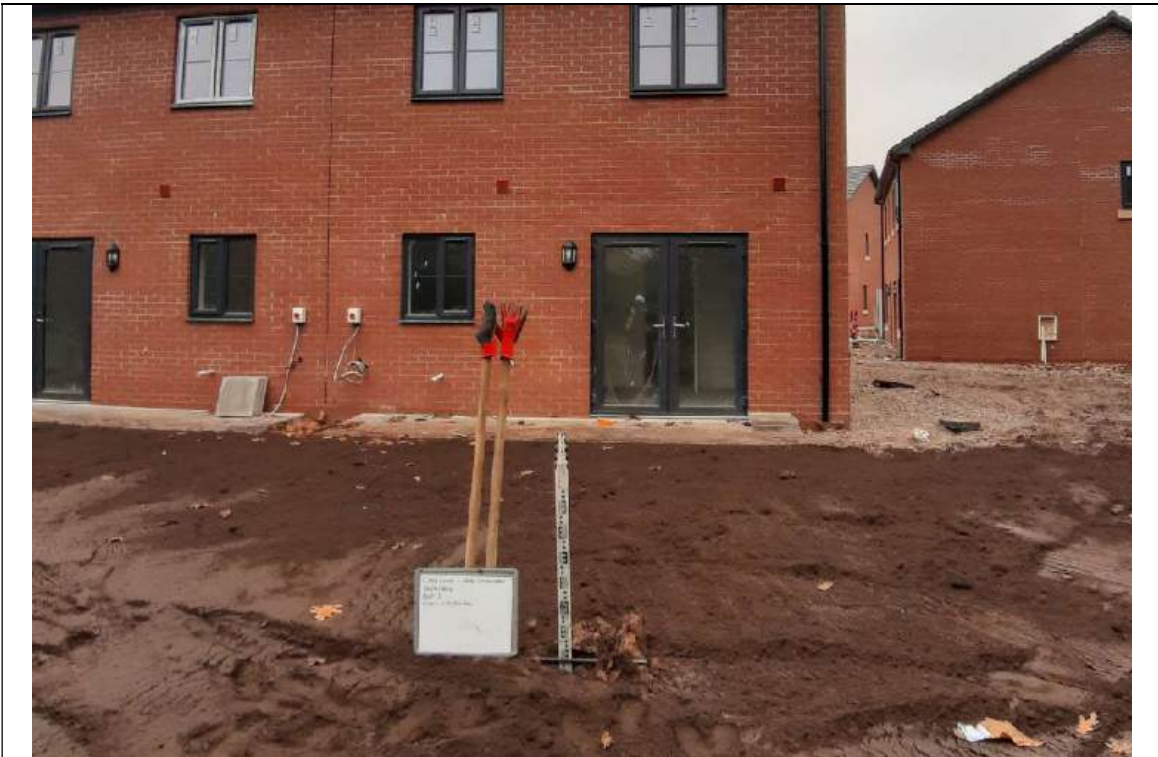
Photo 21 – Showing plot 12 depth validation to 0.30m.
