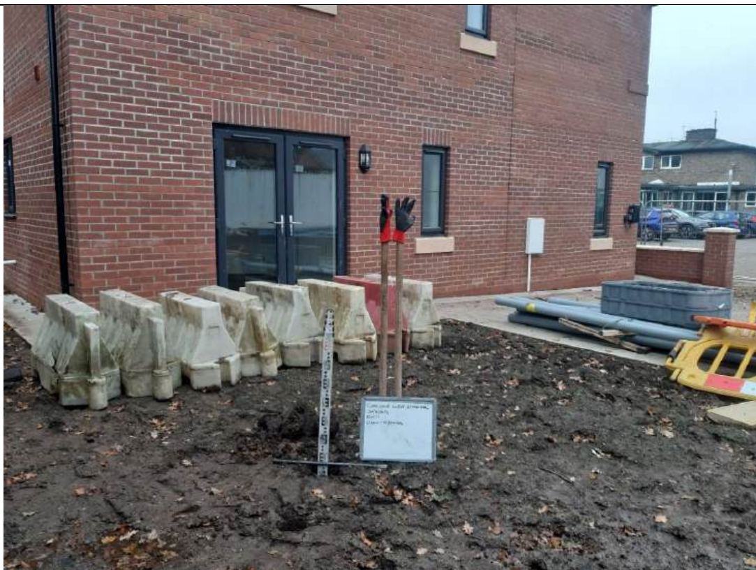
Photo 31 – Showing Plot 19 depth validation to 0.30m.
