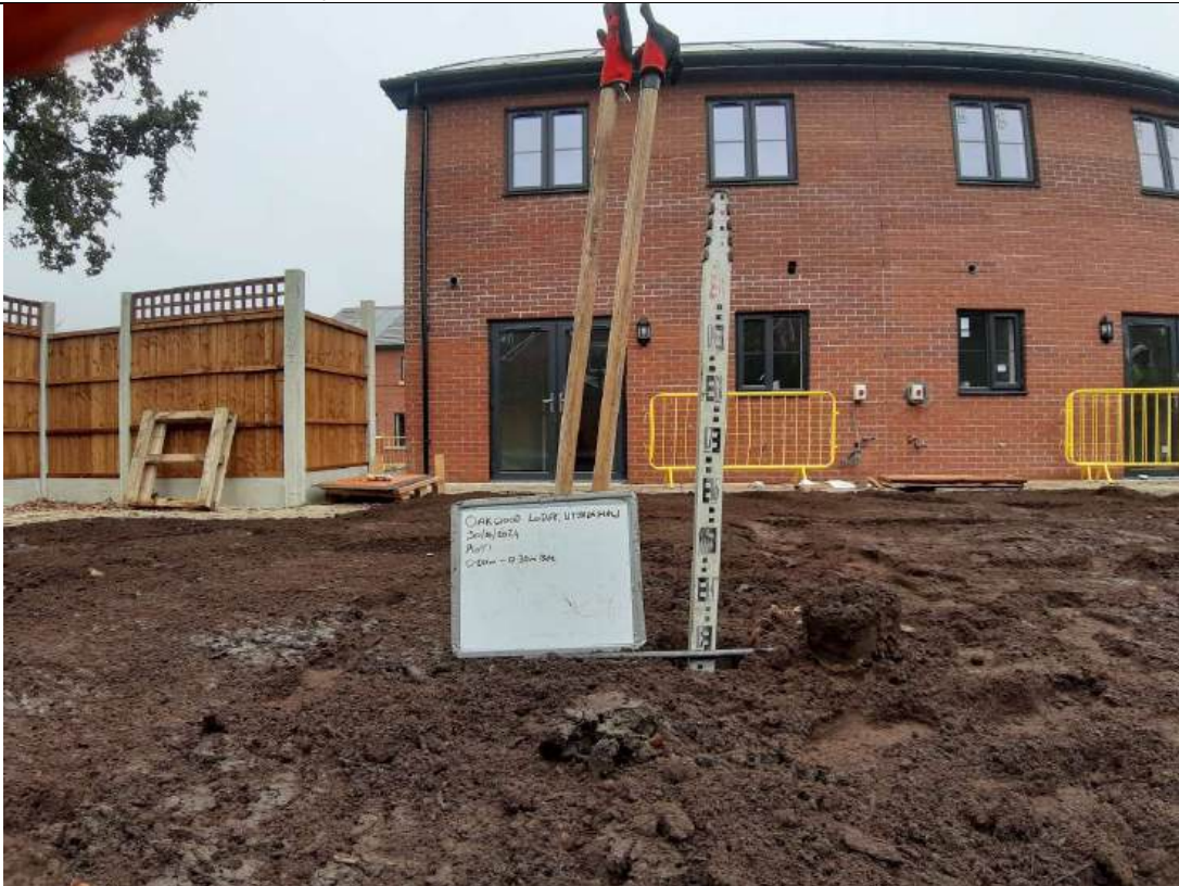
Photo 2 – Showing Plot 1 depth validation to 0.30m.
