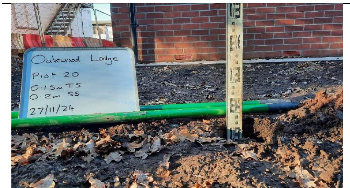
Photo 7 – Showing Plot 20 depth validation to 0.35m.
