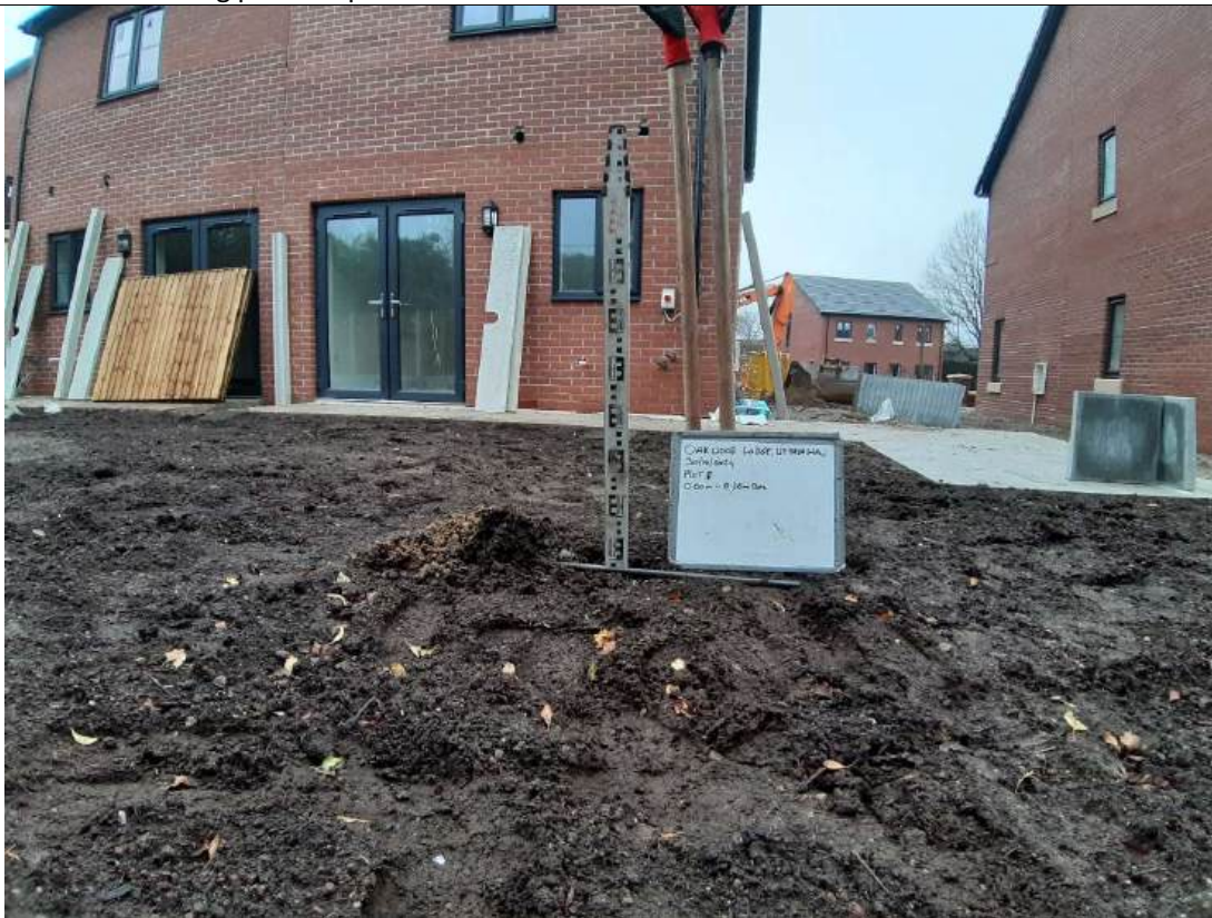
Photo 14 – Showing plot 8 depth validation to 0.30m.
