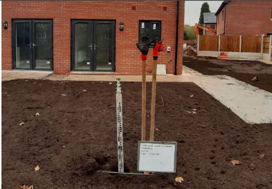
Photo 25: Showing plot 14 depth validation to 0.30m.
