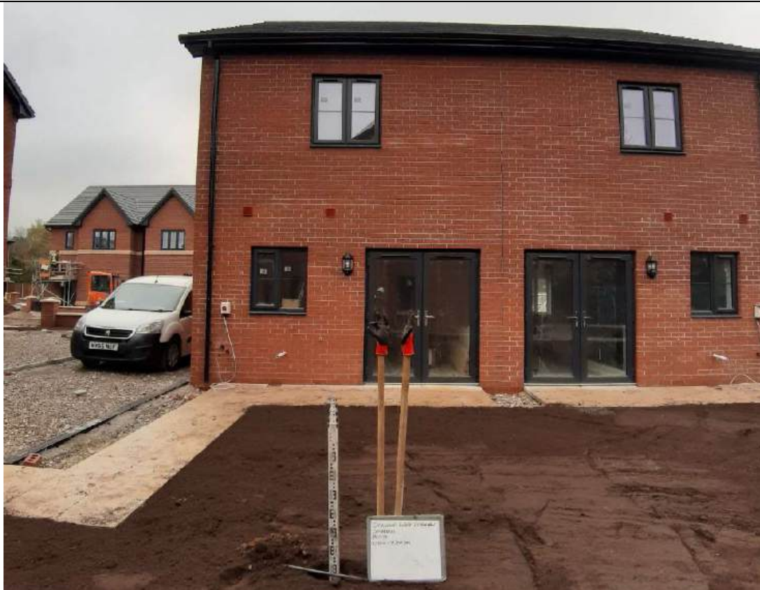
Photo 27 – Showing Plot 17 depth validation to 0.30m.
