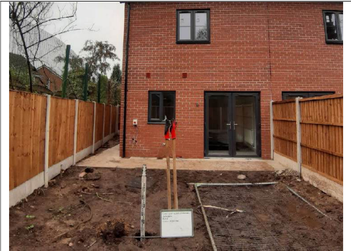
Photo 3 – Showing plot 3 depth validation to 0.30m.
