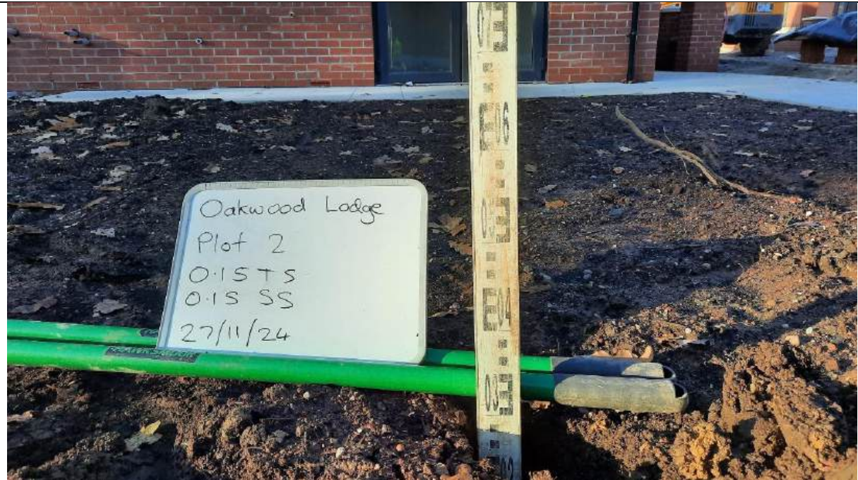
Photo 1 – Showing Plot 2 depth validation to 0.30m.
