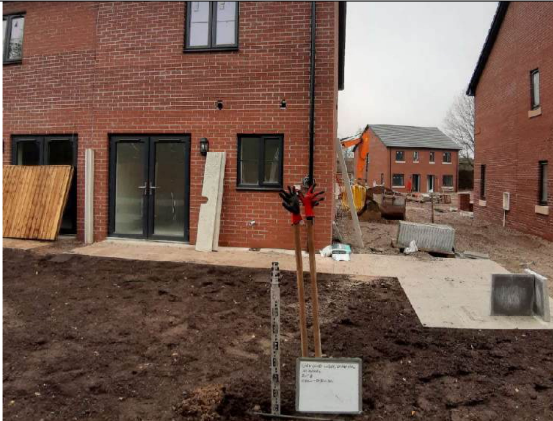
Photo 13 – Showing plot 8 depth validation to 0.30m
