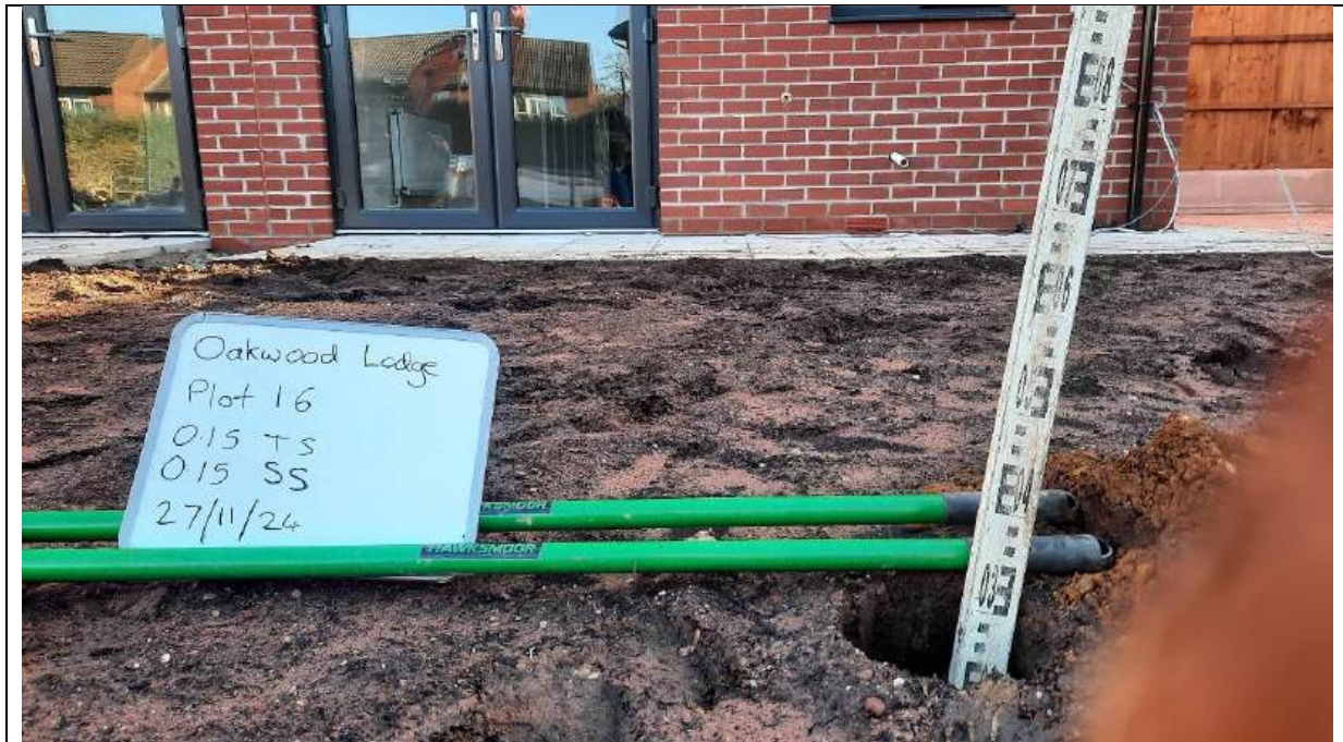
Photo 5 – Showing Plot 16 depth validation to 0.30m.
