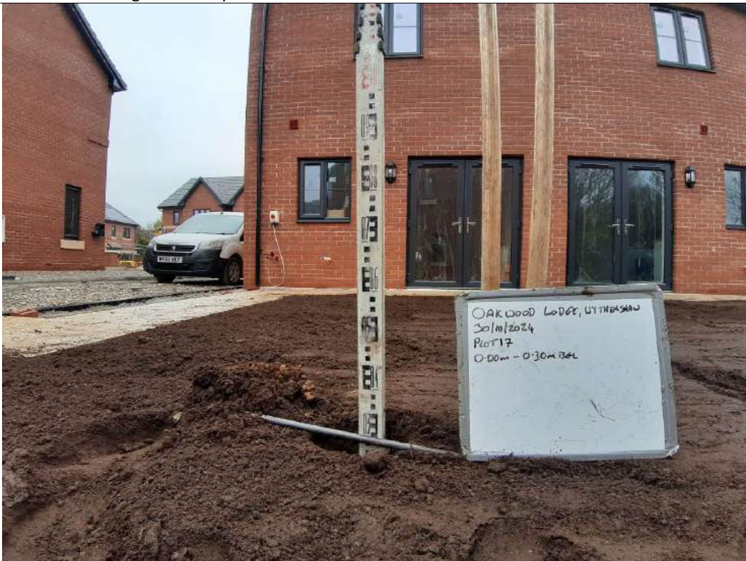
Photo 28 – Showing plot 17 depth validation to 0.30m.
