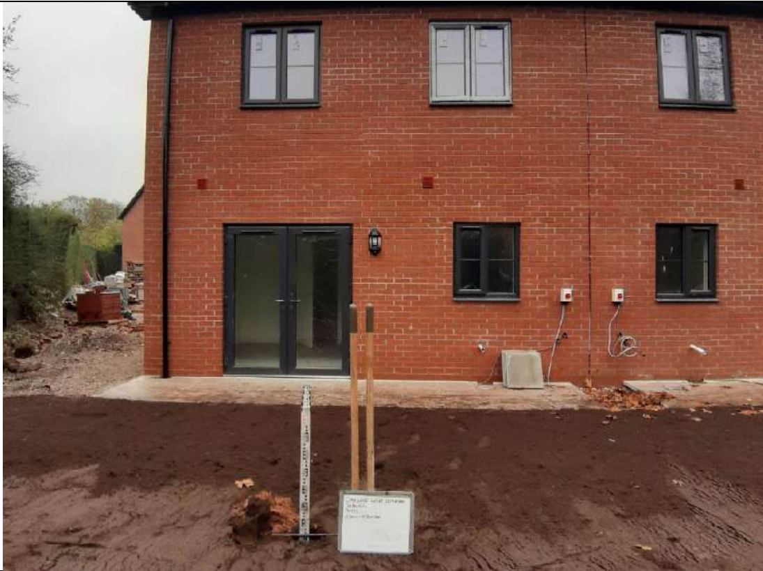
Photo 19 – Showing plot 11 depth validation to 0.30m.
