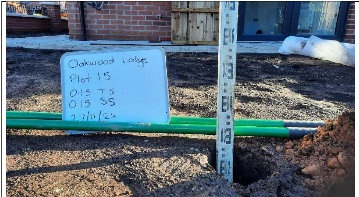
Photo 3 – Showing Plot 15 depth validation to 0.30m.
