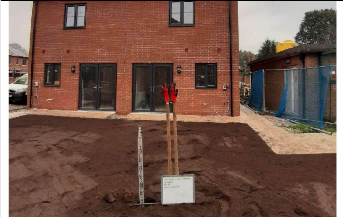
Photo 29 – Showing plot 18 depth validation to 0.30m.
