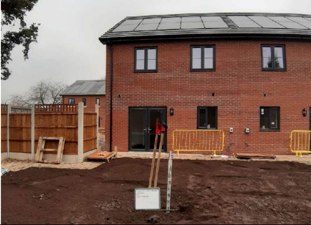
Photo 1 – Showing Plot 1 depth validation to 0.30m.
