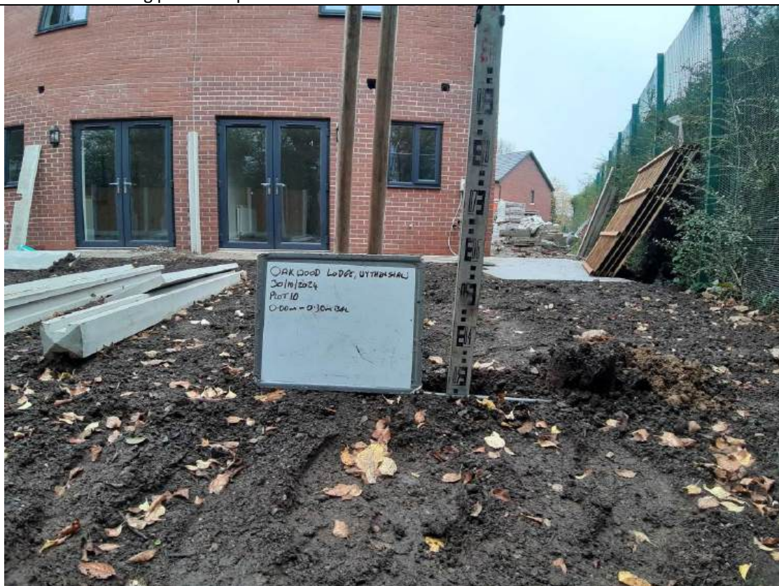
Photo 18 – Showing plot 10 depth validation to 0.30m.
