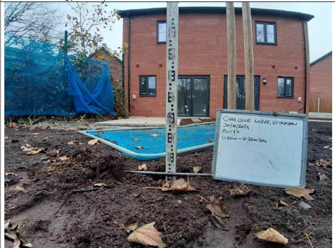
Photo 24: Showing plot 13 depth validation to 0.30m.
