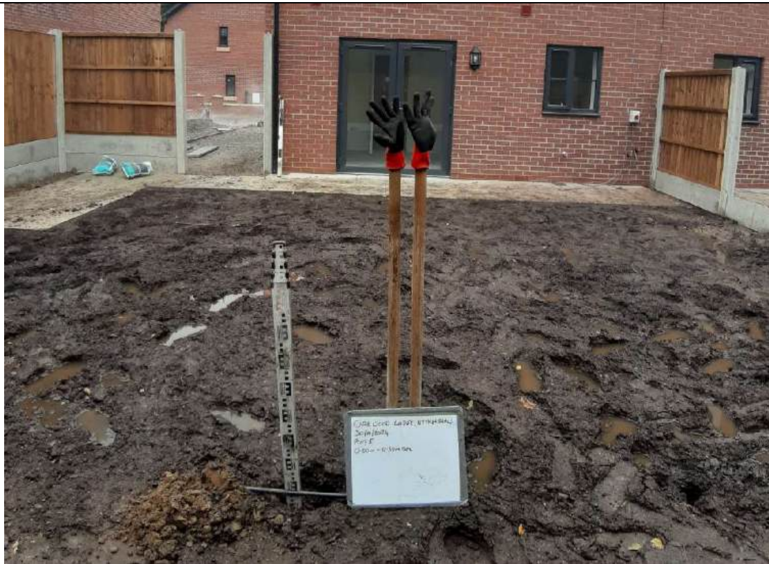
Photo 7 – Showing plot 5 depth validation to 0.30m.
