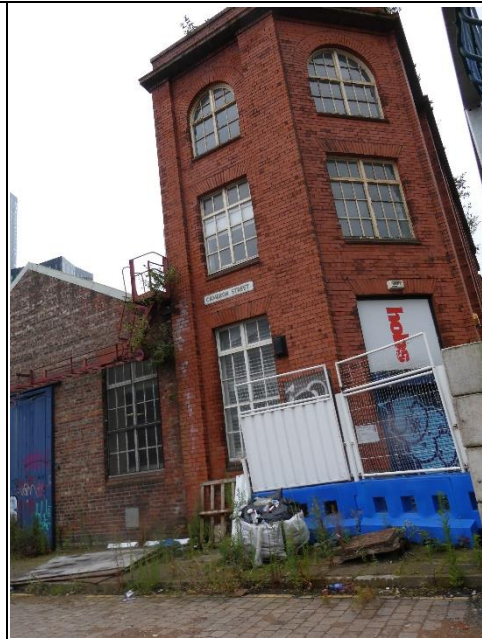
Northeast Elevation of Whitworth House
