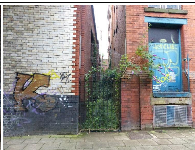
MSJ&A Viaduct to South Whitworth House
