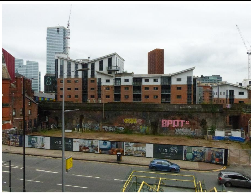
Adjacent Vacant Plot Awaiting Development
