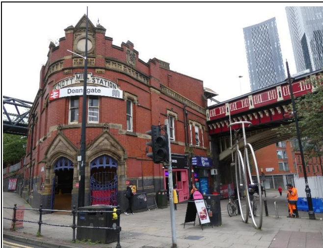
Entrance Deansgate Station
