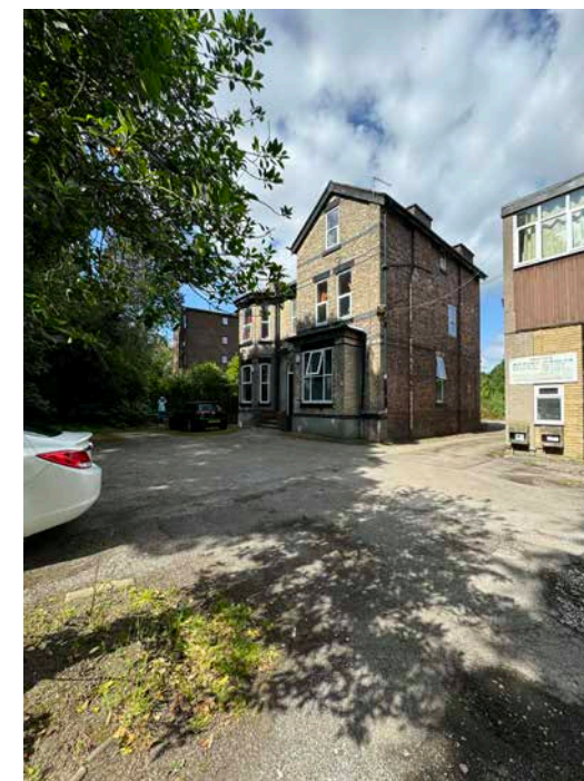
5. View from the site entrance to the existing buildings
