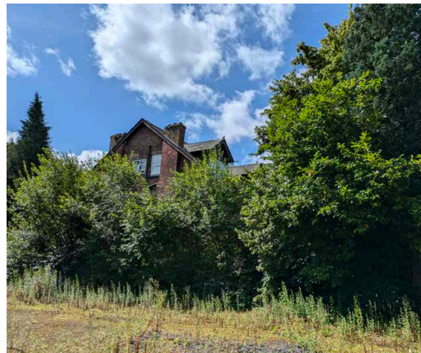
3. View towards the existing buildings from the northern boundary
