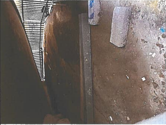
Underside of Access ramp to be propped
