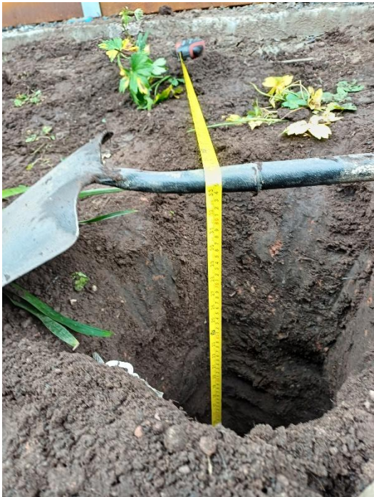
Plate 26: Depth check at MTH109, showing a hole depth of 850 mm.
