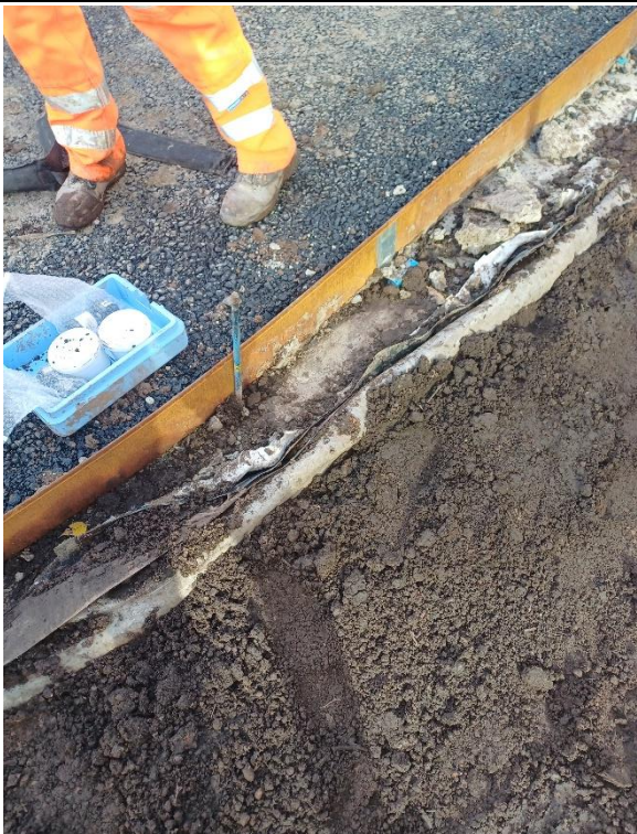
Plate 12: Membrane within raingarden.
