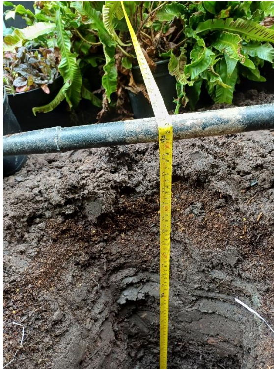
Plate 29: Depth check at MTH110 tree pit, showing a hole depth of 600 mm.
