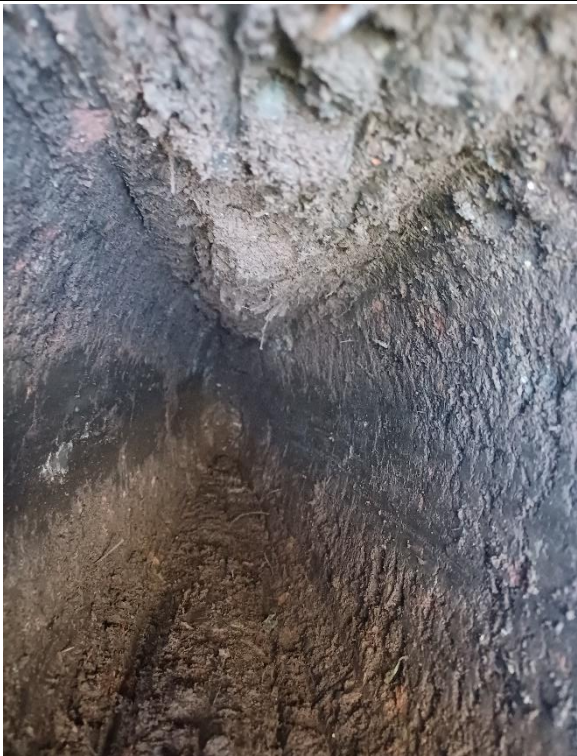
Plate 11: The bottom of MTH102. IDOM verified membrane was indeed present.
