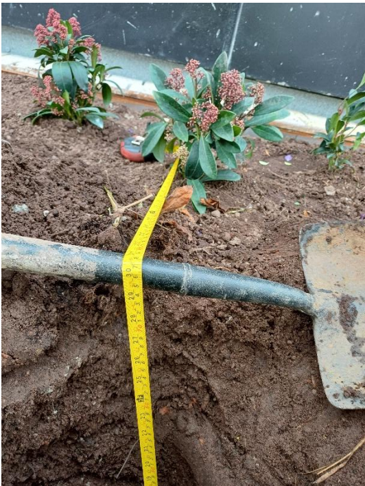
Plate 19: Depth check at MTH106, showing a hole depth of 750 mm.
