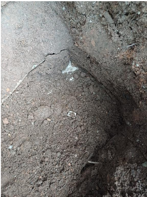
Plate 24: Look downhole at MTH107, showing membrane as the base of the hole.
