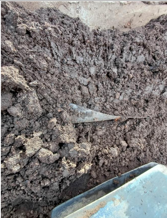
Plate 9: Membrane within raingarden.
