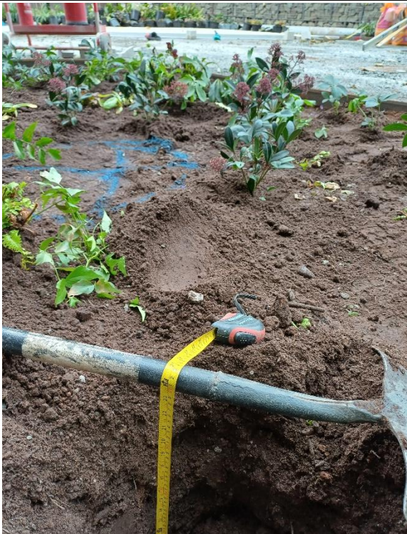
Plate 23: Depth check at MTH107, showing a hole depth of 600 mm.
