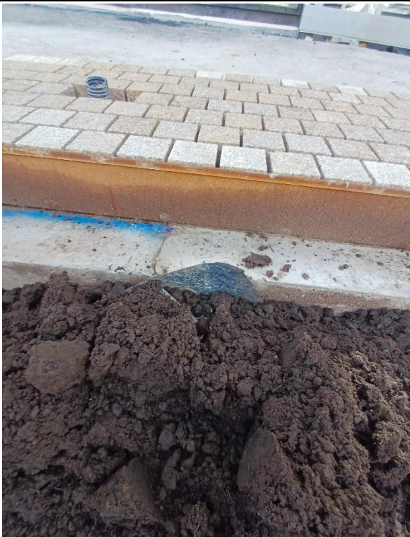
Plate 10: Membrane within raingarden.
