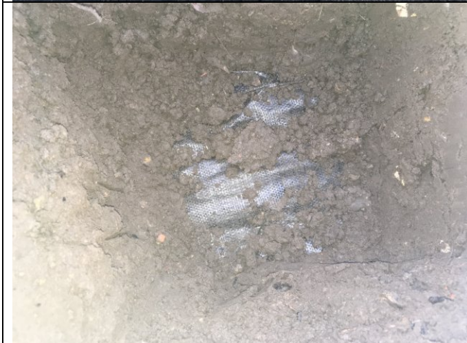
Photograph 9: View of soil in capping layer excavation in rear garden of Plot 27 with geotextile membrane visible.
