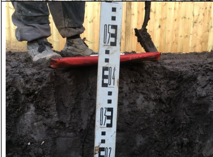
Photograph 16: Depth measurement in rear garden of Plot 28.
