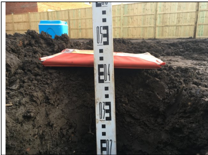
Photograph 4: Depth measurement in rear garden of Plot 26.
