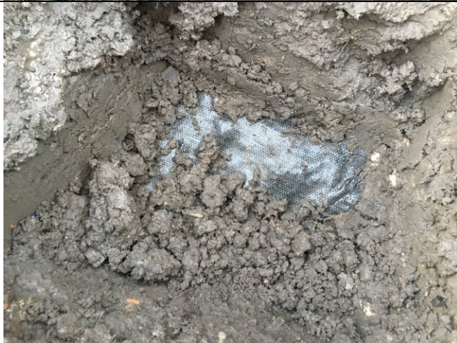
Photograph 12: View of soil in capping layer excavation in front garden of Plot 28 with geotextile membrane visible.
