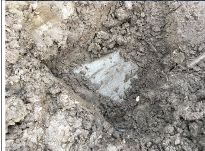
Photograph 15: View of soil in capping layer excavation in rear garden of Plot 28 with geotextile membrane visible.
