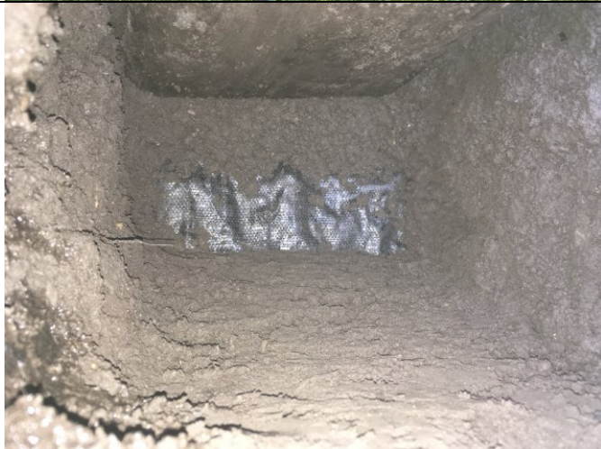
Photograph 6: View of soil in capping layer excavation in front garden of Plot 27 with geotextile membrane visible.
