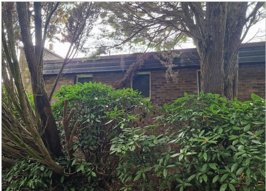
Figure 4.10: Original windows to the south east elevation of the Service Yard building
