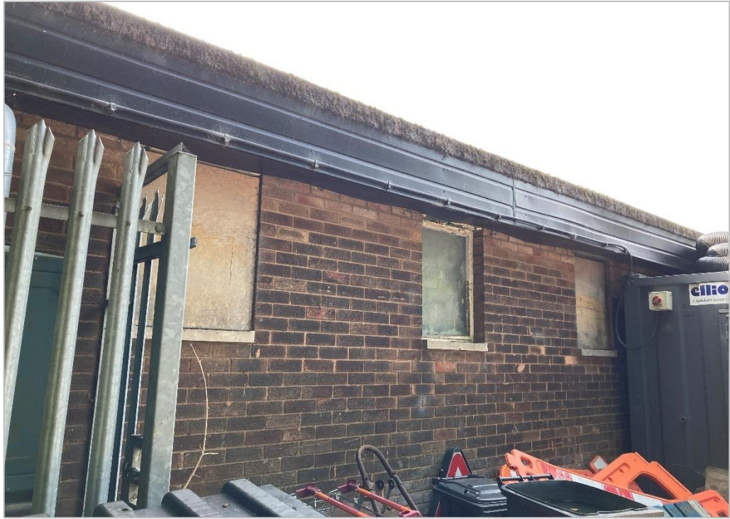
Figure 4.9: Original windows to the north west elevation of the Service Yard building
