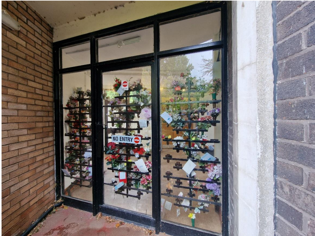
Figure 4.13: Original door to the north west elevation between the Chapel of Remembrance and Offices
