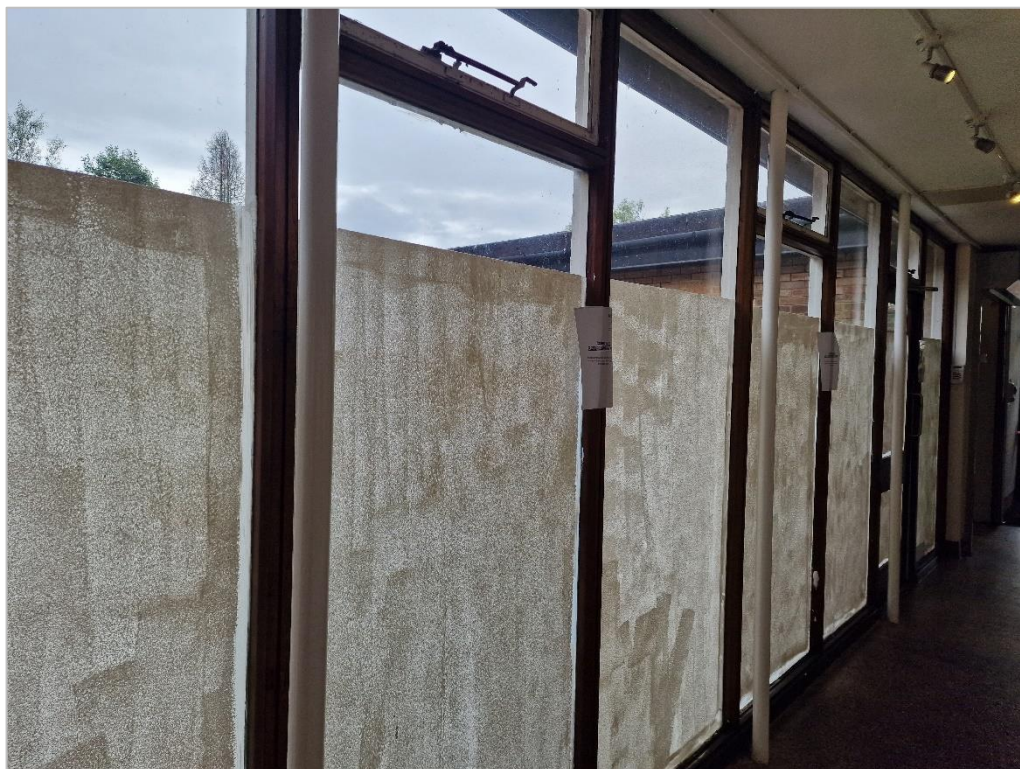
Figure 4.8: Original windows to the courtyard of the Offices
