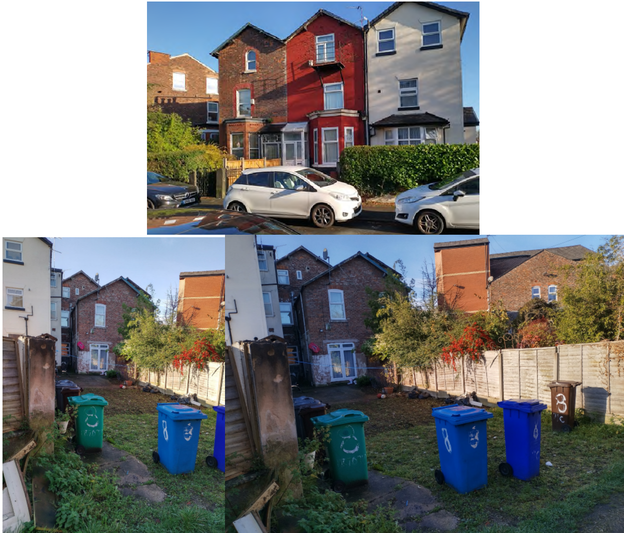
Fig.1 – Views of the front and rear of 8 Victoria Road
