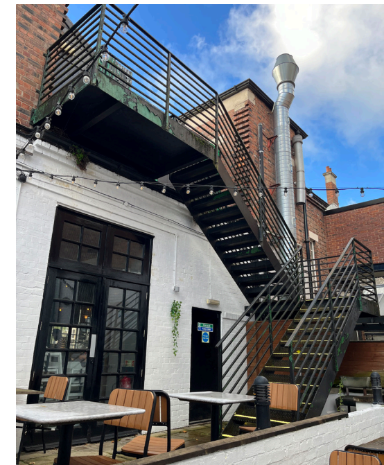
Photograph of rear external stair
