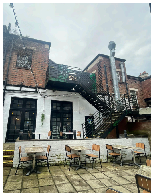
Photograph of rear external space
