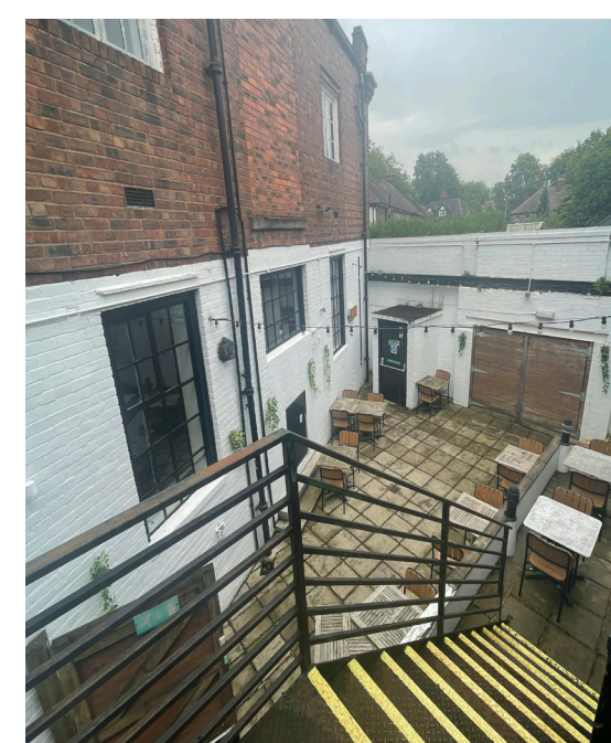
Photograph of rear external space
