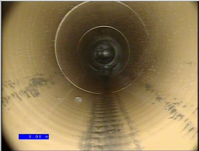
Start node type, manhole, reference S30
