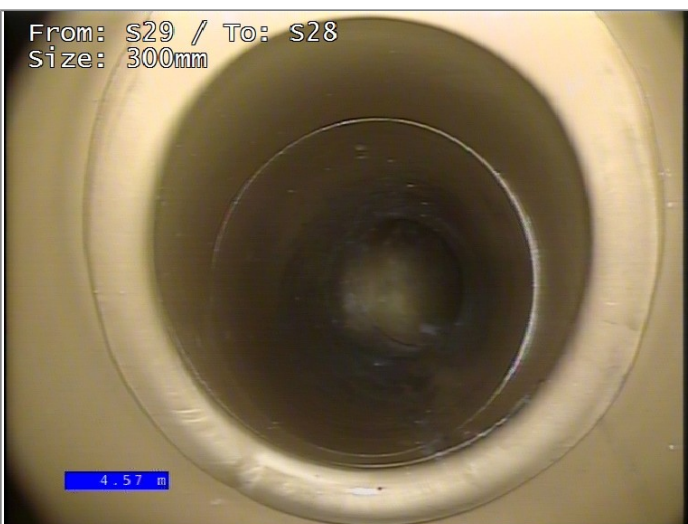
Junction at 2 o'clock, diameter 150mm
