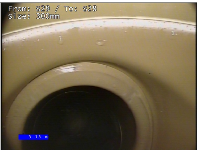
Junction at 10 o'clock, diameter 150mm
