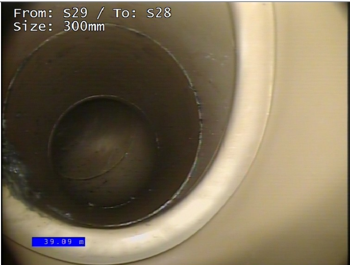
Junction at 10 o'clock, diameter 150mm
