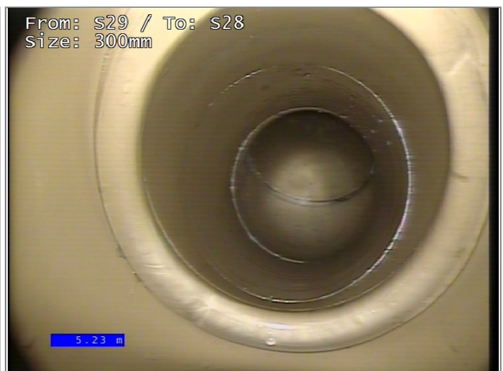
Junction at 2 o'clock, diameter 150mm
