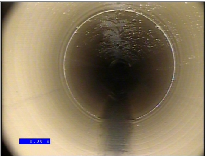
Start node type, manhole, reference S29
