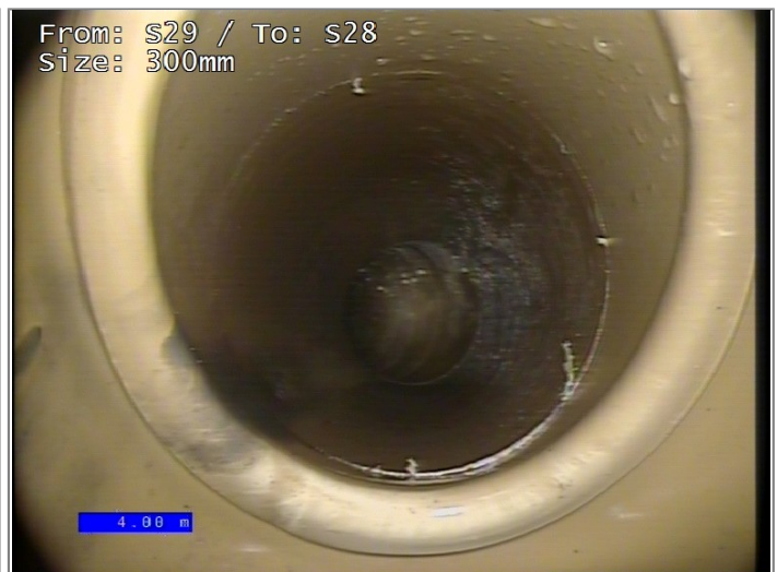
Junction at 10 o'clock, diameter 150mm
