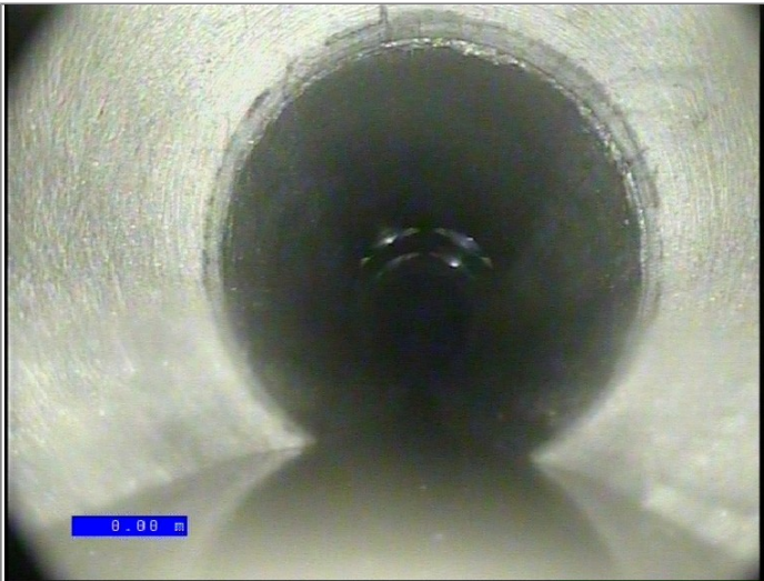
Start node type, manhole, reference S42
