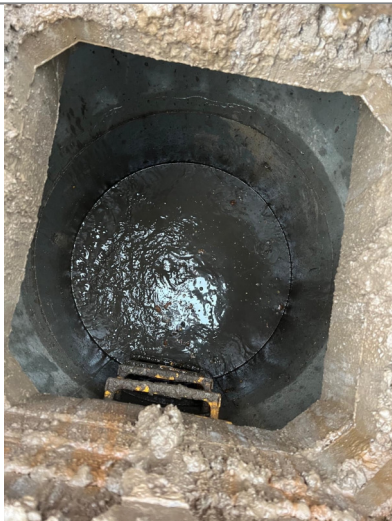
Other Site Photos: F9
