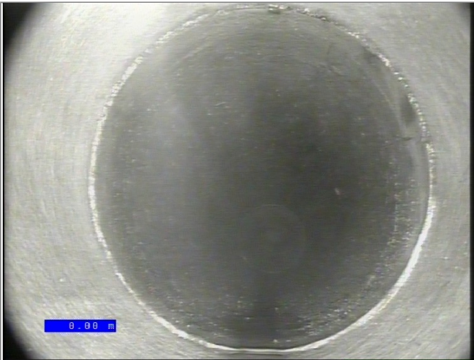
Start node type, manhole, reference S42
