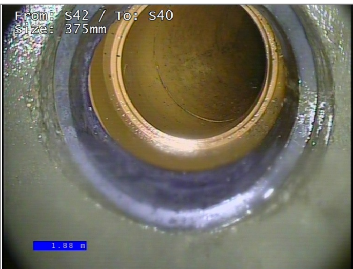
Connection other than junction at 1 o'clock, diameter 150mm
