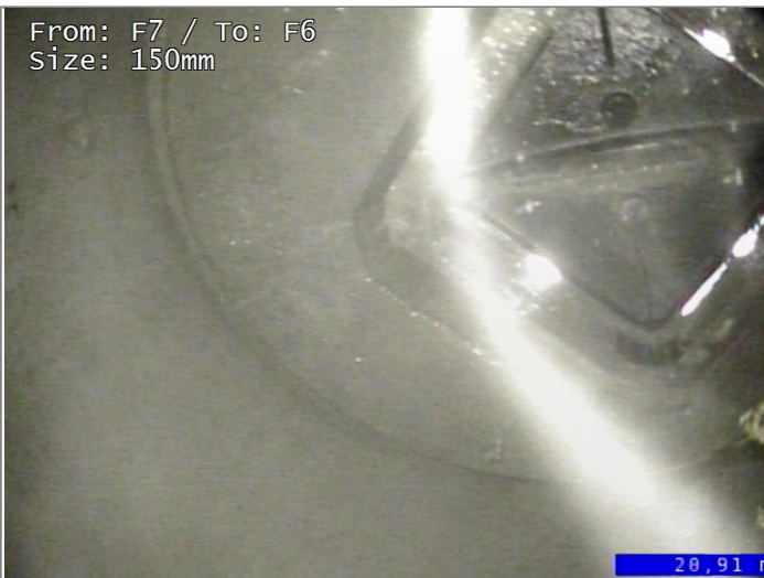
Finish node type, manhole, reference F6
