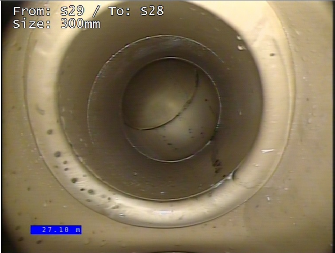
Junction at 2 o'clock, diameter 150mm
