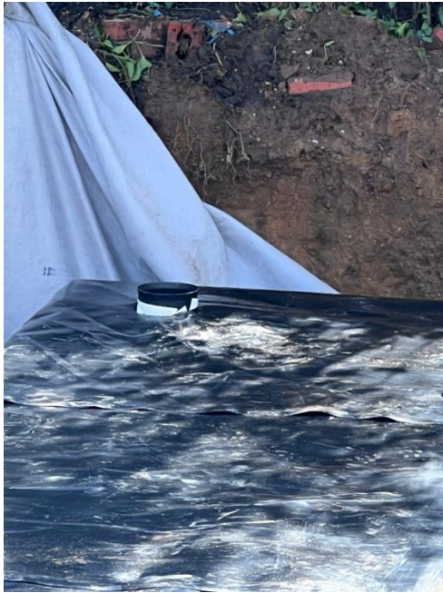
Installation of venting pipe to attenuation
