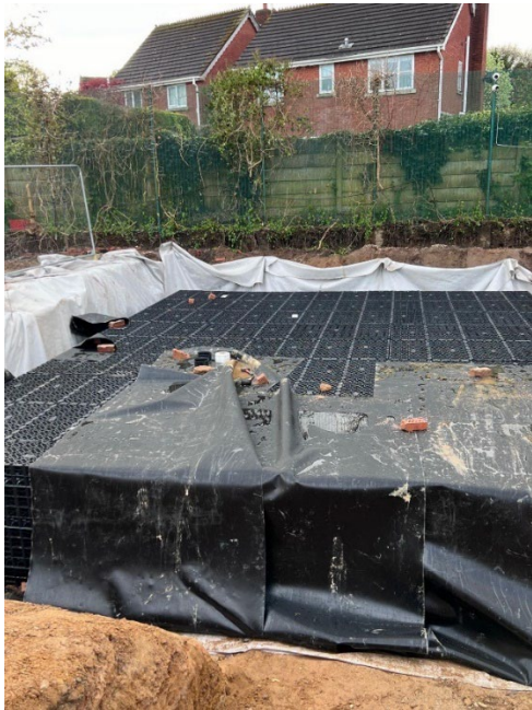
Installation of cellular attenuation
