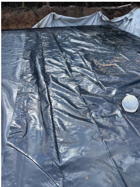
Installation of impermeable wrapping
