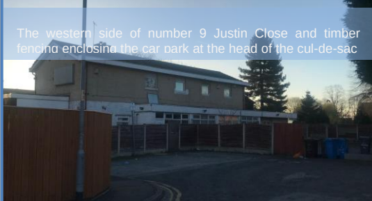
The western (front) elevation of number 9 Justin Close
