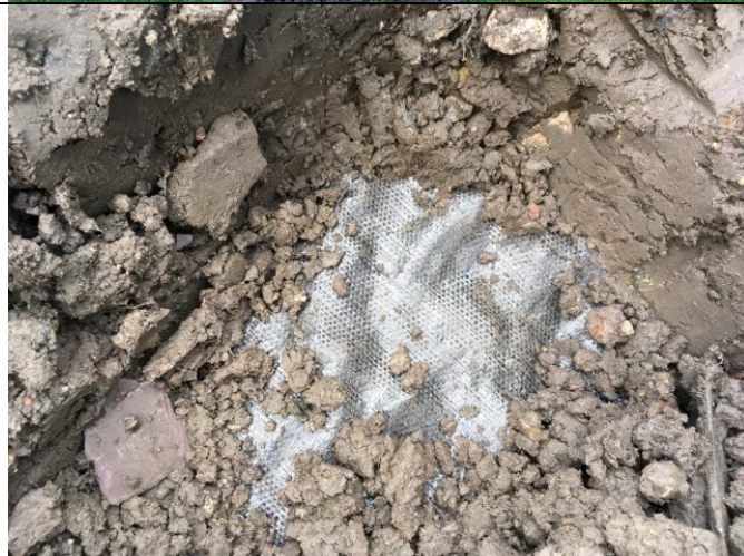
Photograph 11: View of soil in capping layer excavation in rear garden of Plot 34 with geotextile membrane visible.
