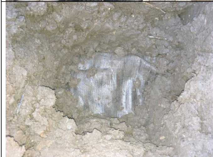
Photograph 14: View of soil in capping layer excavation in front garden of Plot 43 with geotextile membrane visible.
