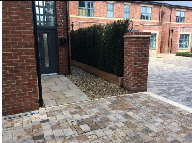
Photograph 9: View of front garden of Plot 34. To be fully hardstood.
