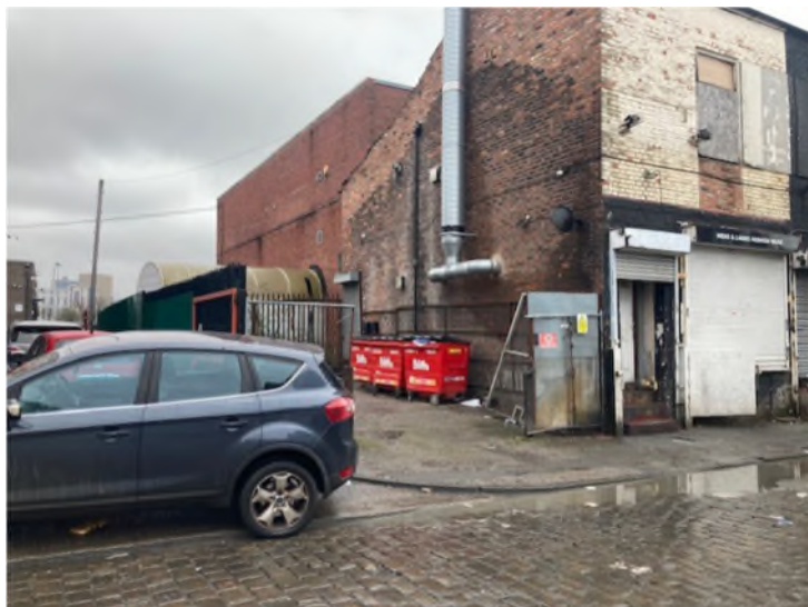
View of the rear of the premises
