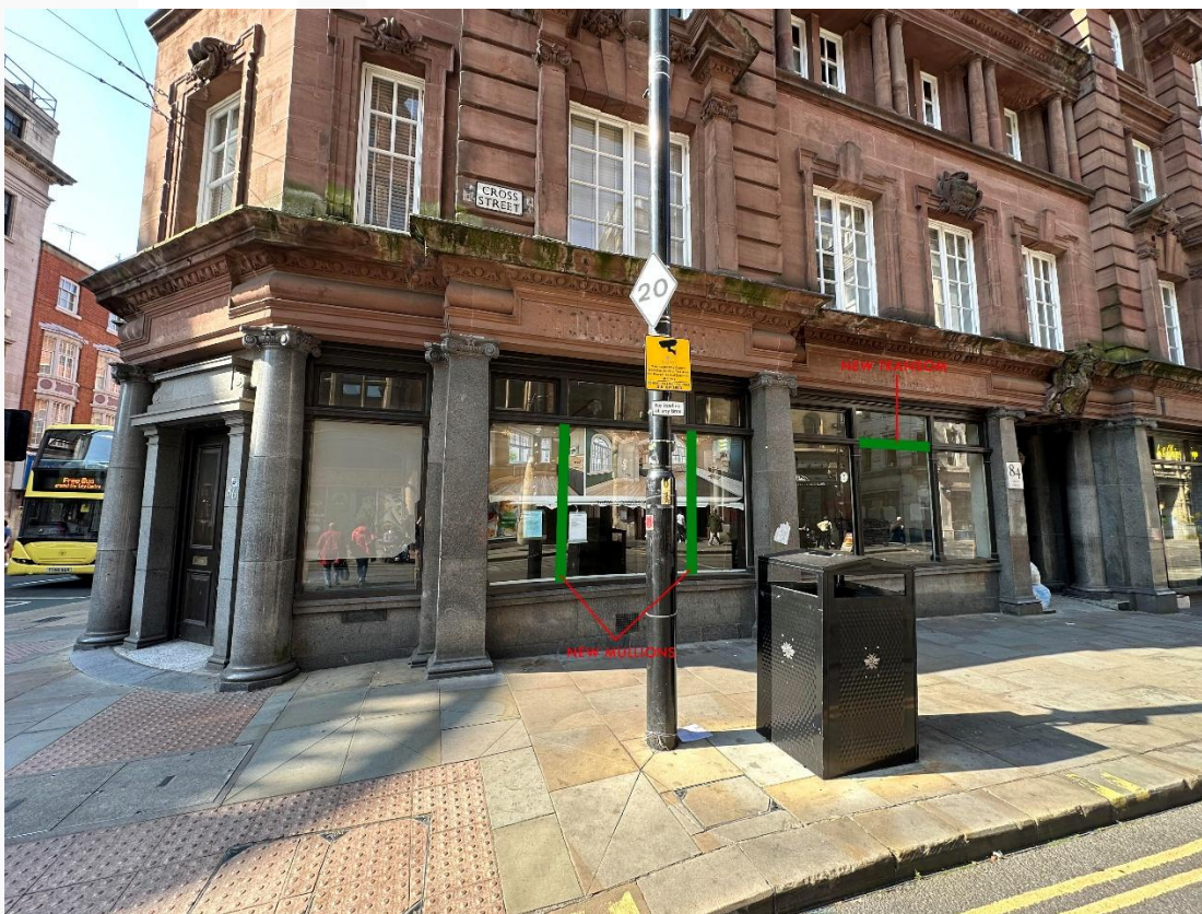
Photo showing the addition of mullions and transom to Cross Street Elevation windows
