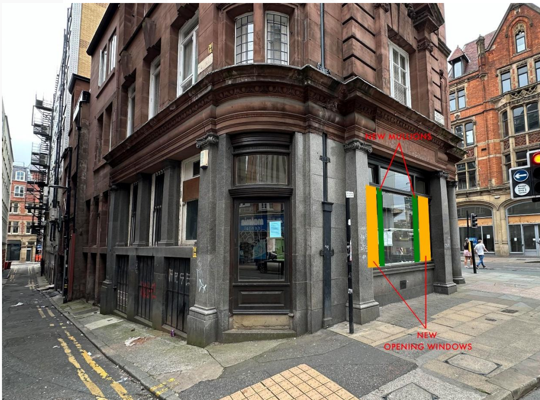
Photo showing the addition of mullions and opening windows to John Dalton Street Elevation windows
