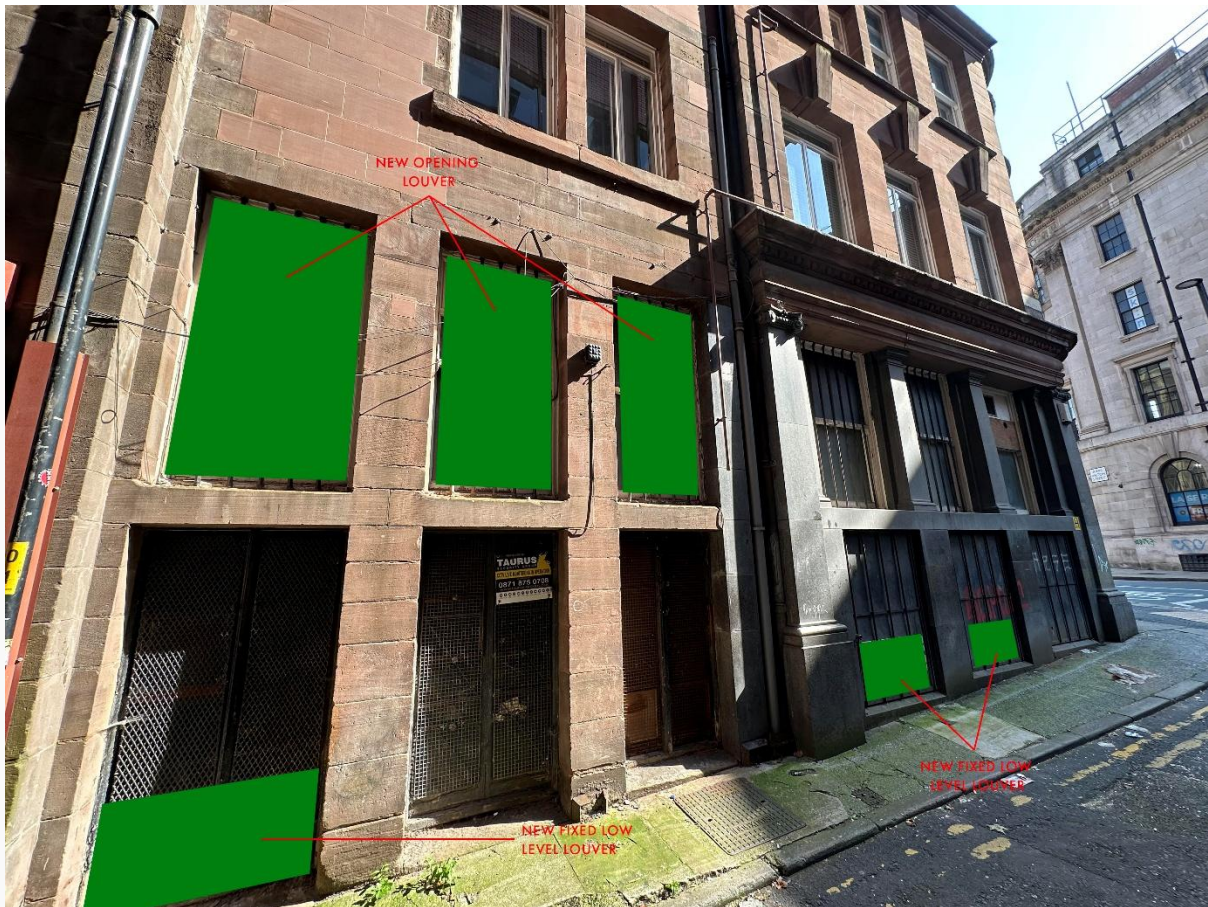
Photo showing the addition of louvers to Four Yards Elevation windows
