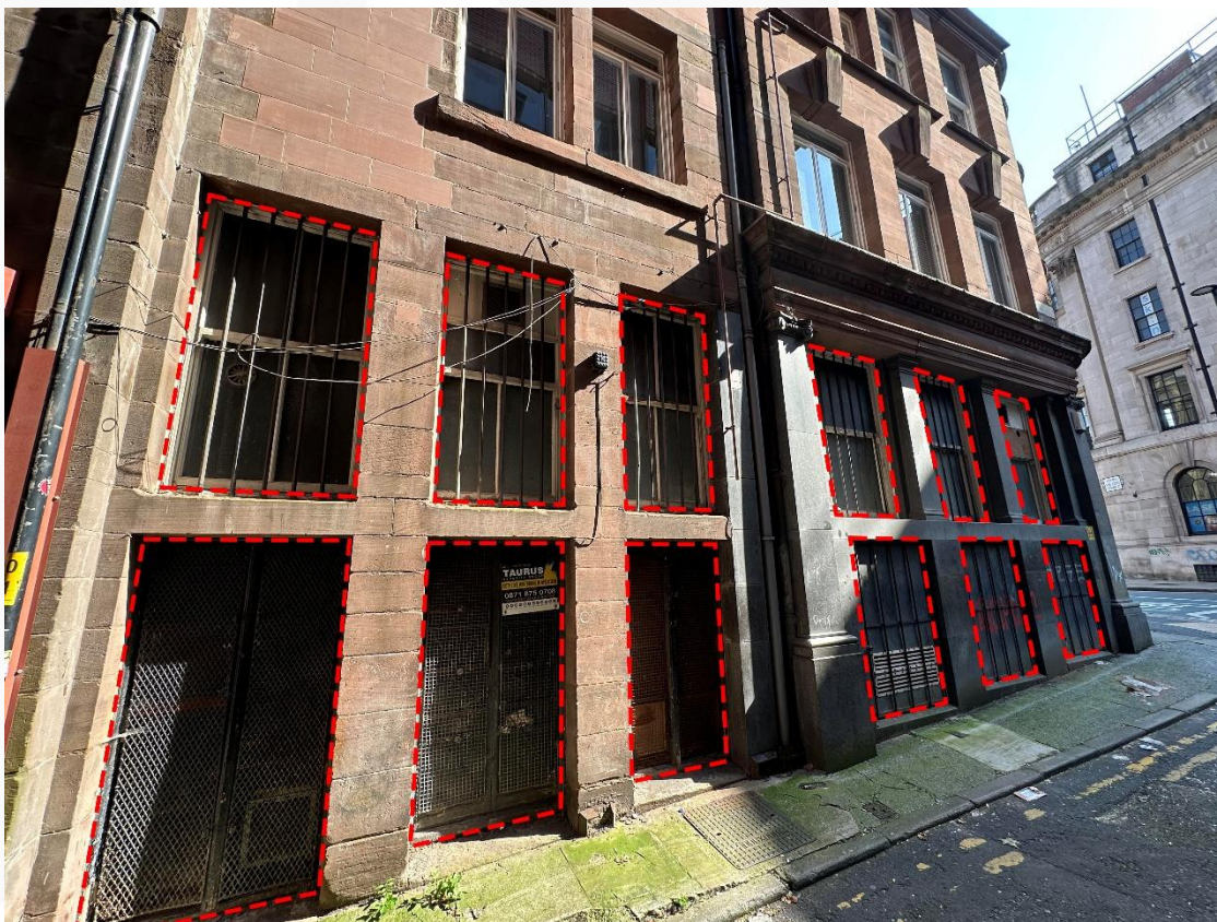
Photo showing Four Yards Elevation showing existing security bars and coverings
