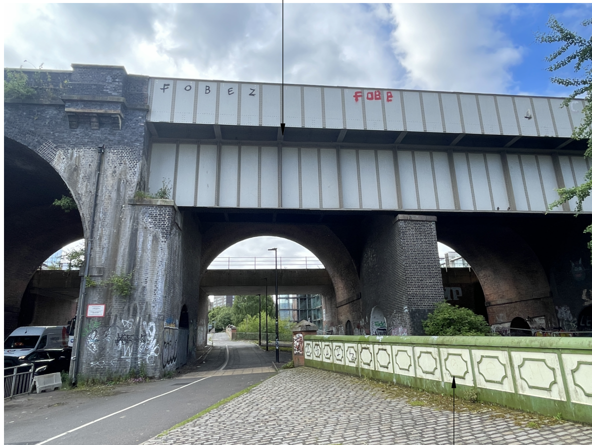
Metal parapet to late C20th bridge
