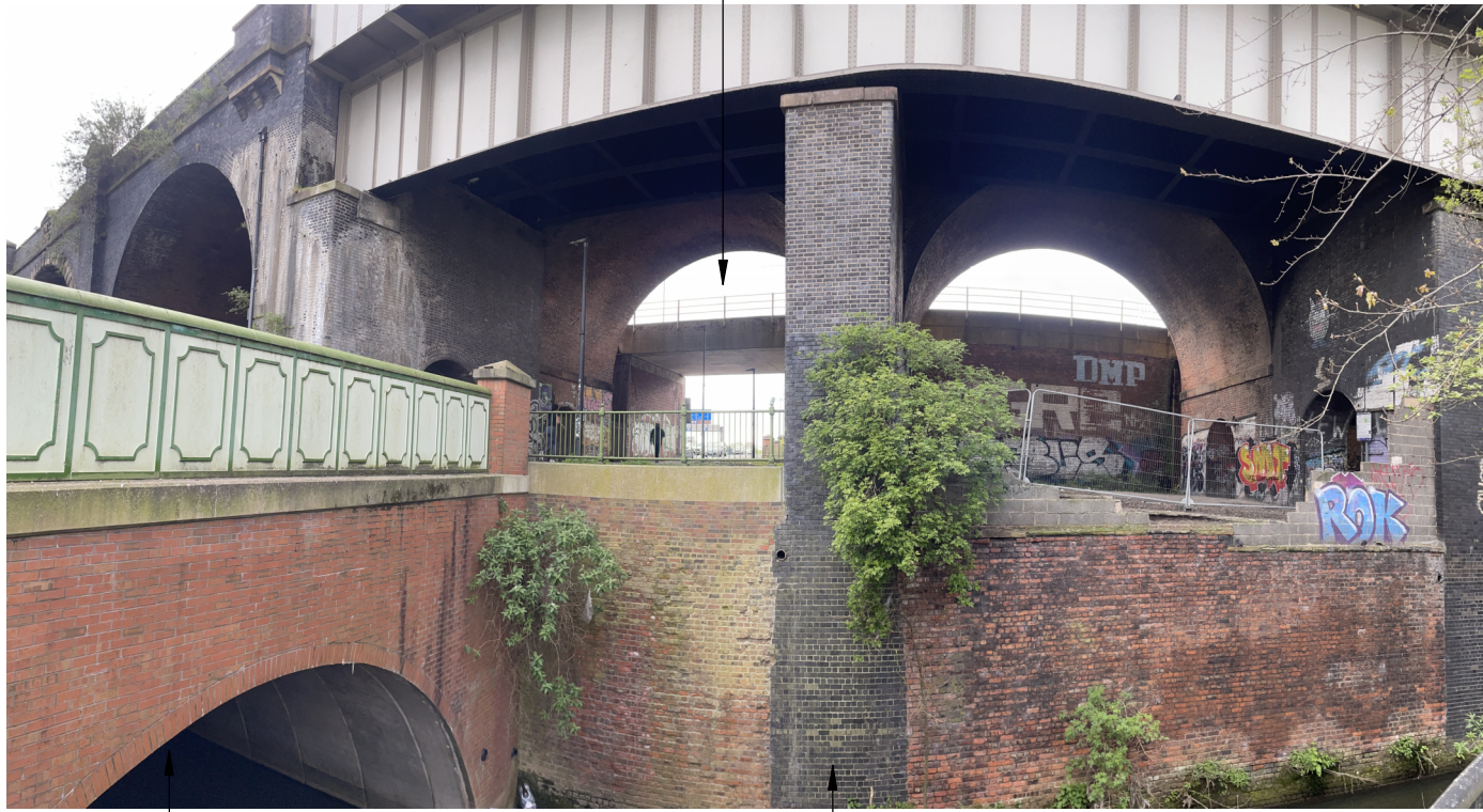
TfGM viaduct piers continue down; river wall brickwork stop-starts each side
