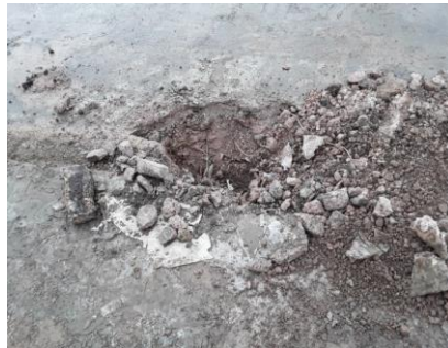
Item 5 - Trial pit 5 - Soil sample taken from the top 200mm layer, beneath the concrete layer
