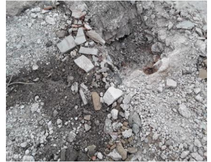
Item 21 - Concrete slab - Felt used as a damp proof course beneath the former walls throughout the site
