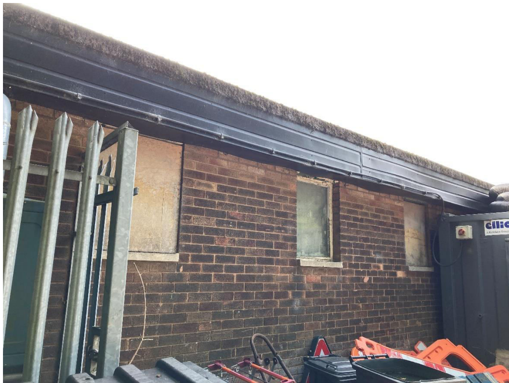
Image 02 – Ladder Access Location Nr.1
