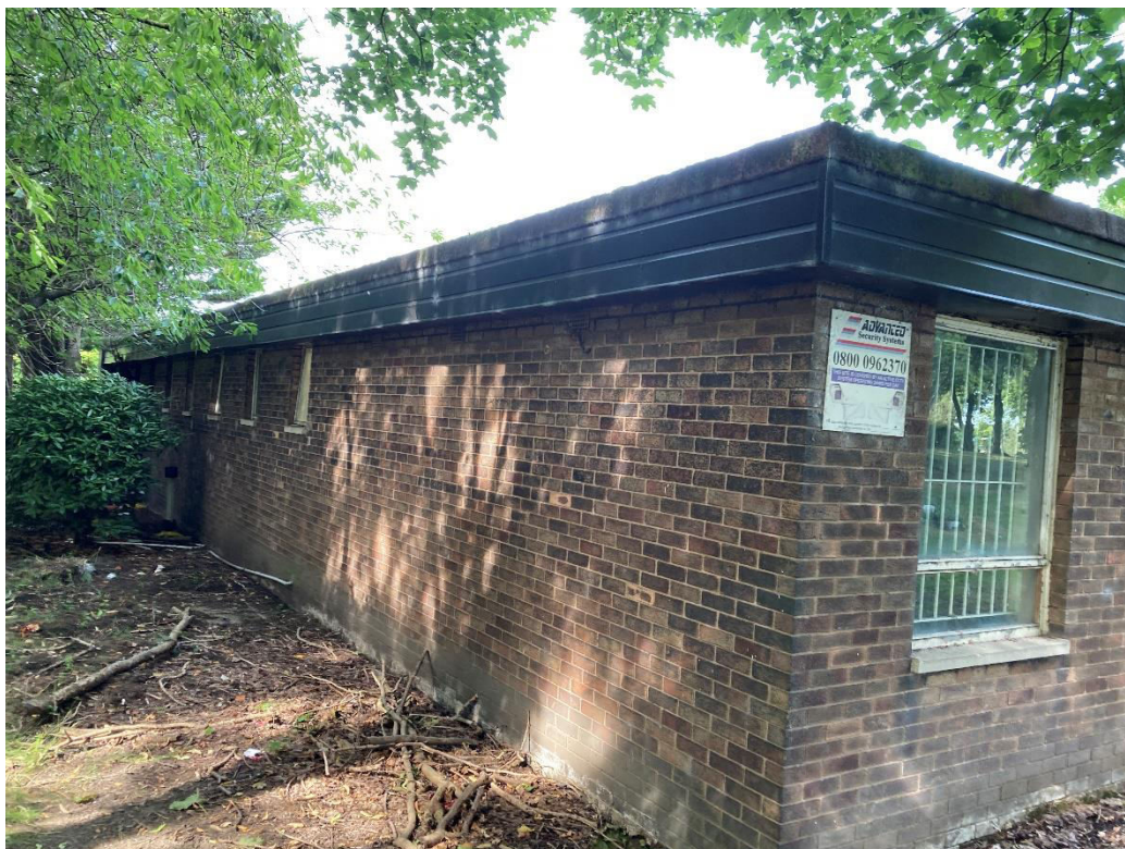
Image 04 – Outer wall to receive low level pipework and cable tray protrusions
