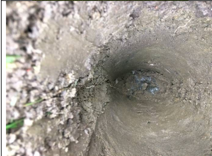
Photograph 11: View of soil in capping layer excavation in rear garden of Plot 41 with geotextile membrane visible.
