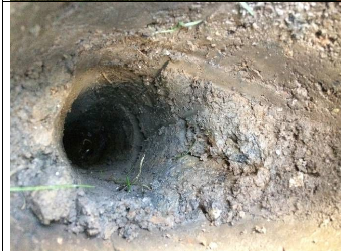
Photograph 17: View of soil in capping layer excavation in rear garden of Plot 42 with geotextile membrane visible.
