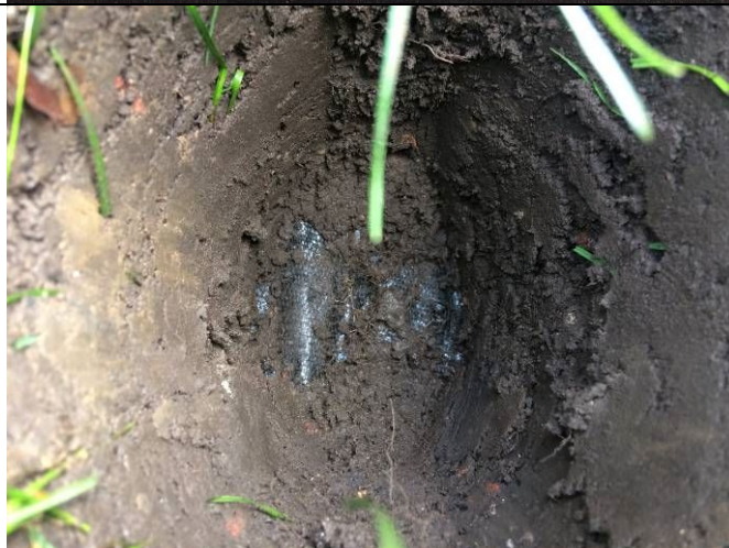
Photograph 14: View of soil in capping layer excavation in front garden of Plot 42 with geotextile membrane visible.
