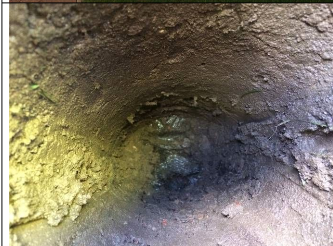
Photograph 2: View of soil in capping layer excavation in front garden of Plot 40 with geotextile membrane visible.
