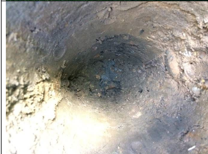
Photograph 5: View of soil in capping layer excavation in rear garden of Plot 40 with geotextile membrane visible.
