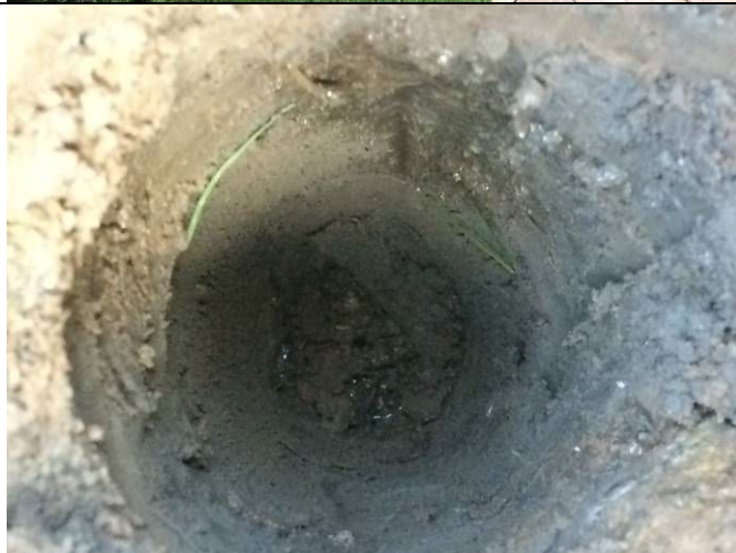
Photograph 8: View of soil in capping layer excavation in front garden of Plot 41 with geotextile membrane visible.
