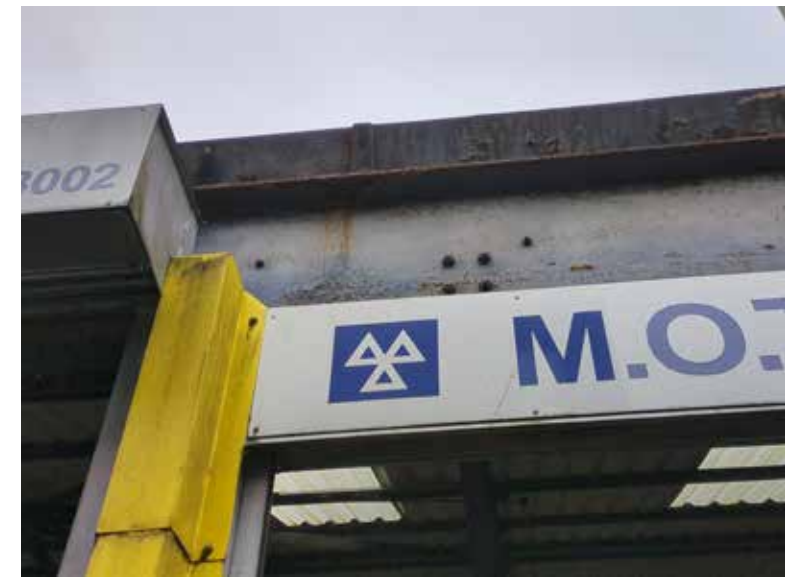
Existing facade to Henry Street
