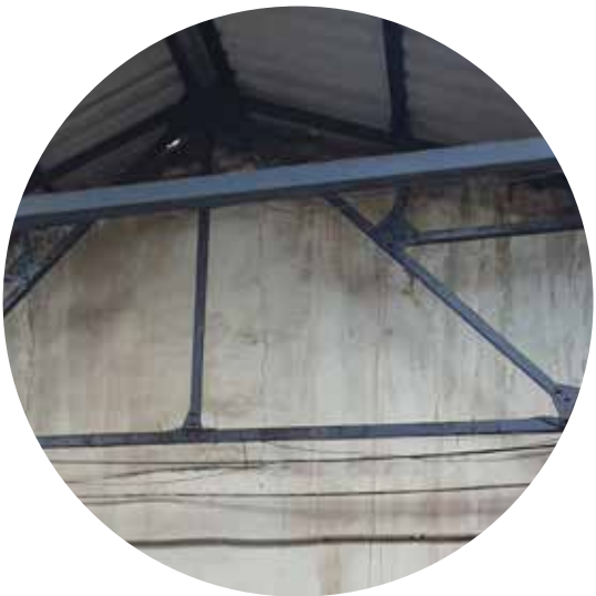
Existing steel framing
