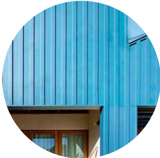
Coloured corrugated metal cladding
