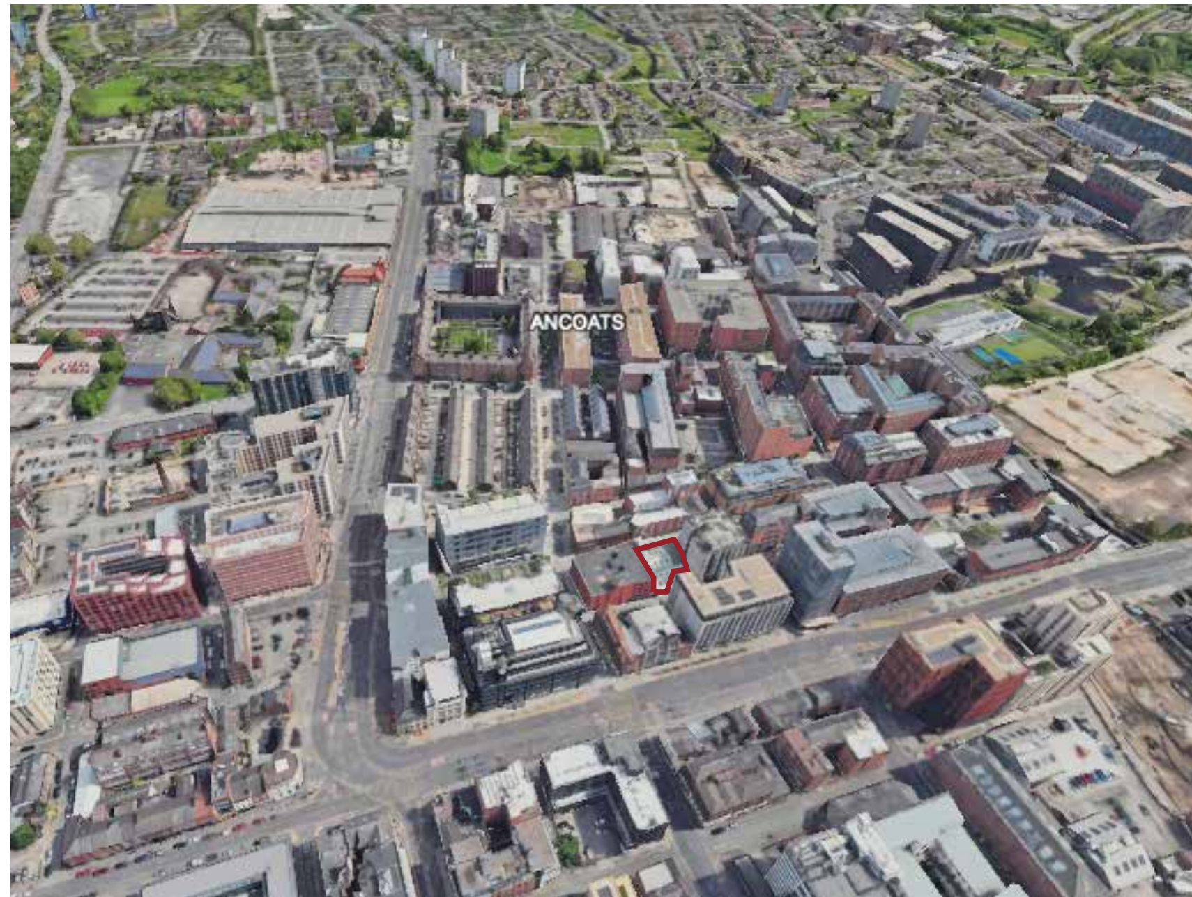
Aerial view of Ancoats and site looking Eastwards with approximate site boundary
