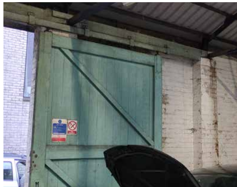
Existing timber sliding door
