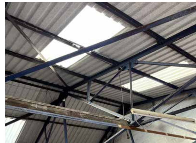
Existing structure and corrugated metal roofing
