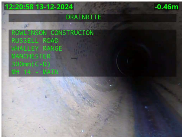
MH 14X_065e9c99-63dc-40ba-a226-db2774414a60_20241213_1 32147_427.jpg, 0.00 m Water level, 0% of the vertical dimension
