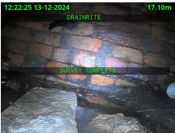
MH 14X_e907fa0c-6733-493b-bab0-421952fc6e6e_20241213_13 2940_886.jpg, 00:01:29, 17.10 m Finish node, manhole, reference: MAIN
