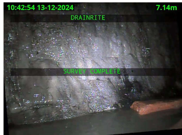
MH 25X_18025c35-1e8a-446b-a412-240a4fc0d8b0_20241213_13 1905_379.jpg, 00:00:43, 7.14 m Finish node, manhole, reference: MAIN
