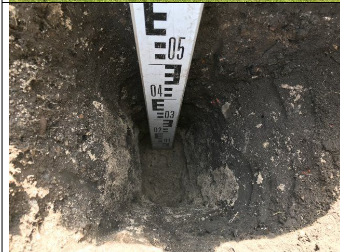
Photograph 30: View of soil in capping layer excavation in rear garden of The Lodge with MOT visible.
