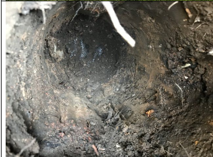
Photograph 24: View of soil in capping layer excavation in rear garden of Plot 39 with geotextile membrane visible.
