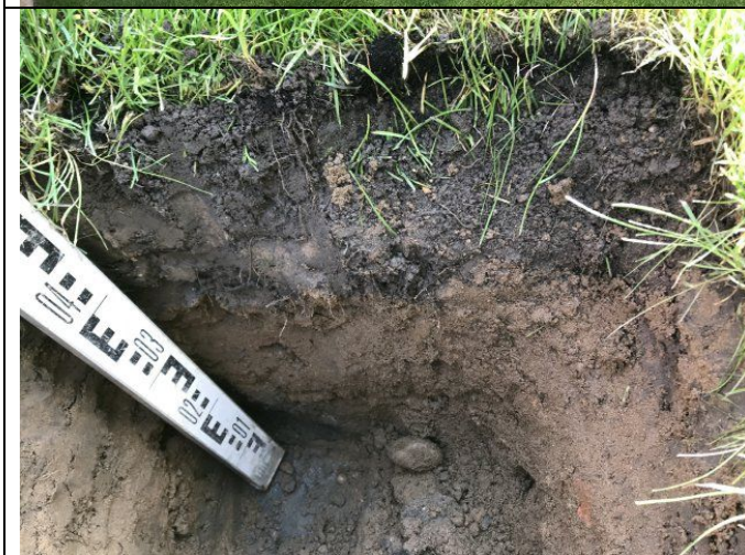
Photograph 3: View of soil in capping layer excavation in rear garden of Plot 19 with geotextile membrane visible.
