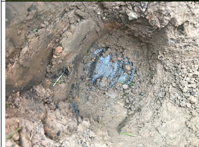
Photograph 21: View of soil in capping layer excavation in front garden of Plot 39 with geotextile membrane visible.
