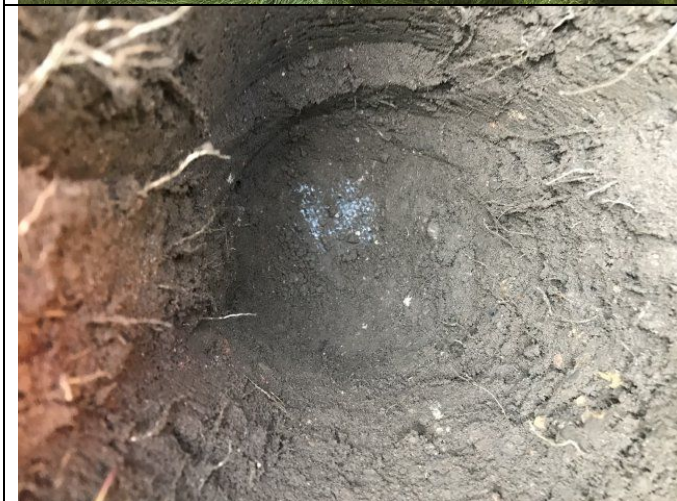
Photograph 18: View of soil in capping layer excavation in rear garden of Plot 38 with geotextile membrane visible.
