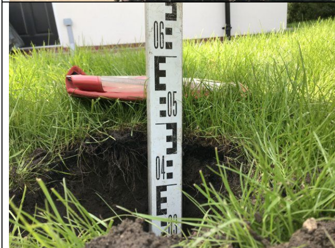
Photograph 27: View of soil in capping layer excavation in rear garden of Plot 801 with geotextile membrane visible.
