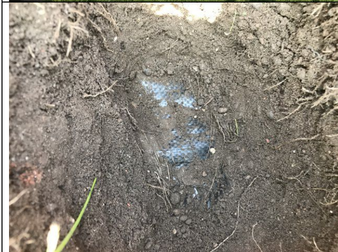
Photograph 11: View of soil in capping layer excavation in front garden of Plot 37 with geotextile membrane visible.
