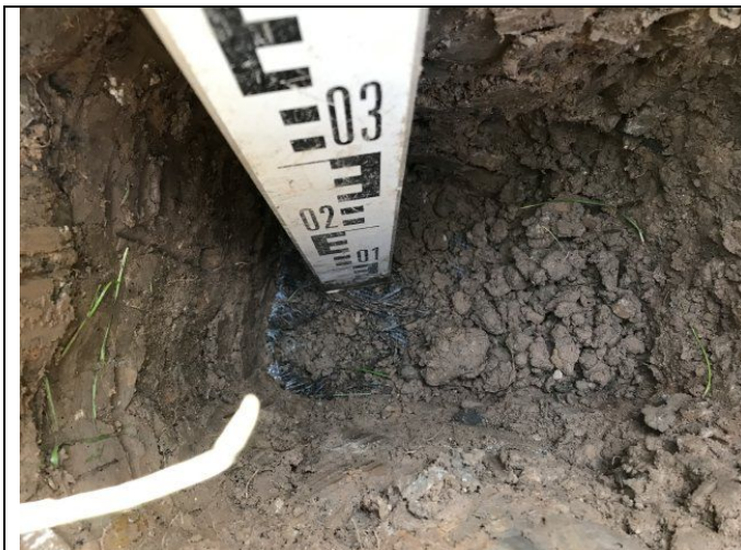
Photograph 8: View of soil in capping layer excavation in rear garden of Plot 25 with geotextile membrane visible.
