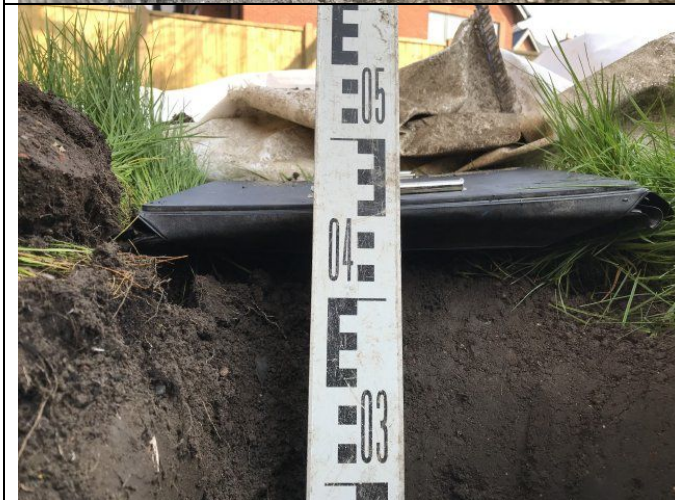
Photograph 15: Depth measurement in rear garden of Plot 37.
