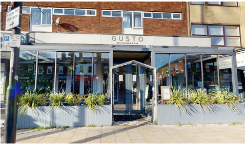
EXISTING SHOPFRONT PHOTO
