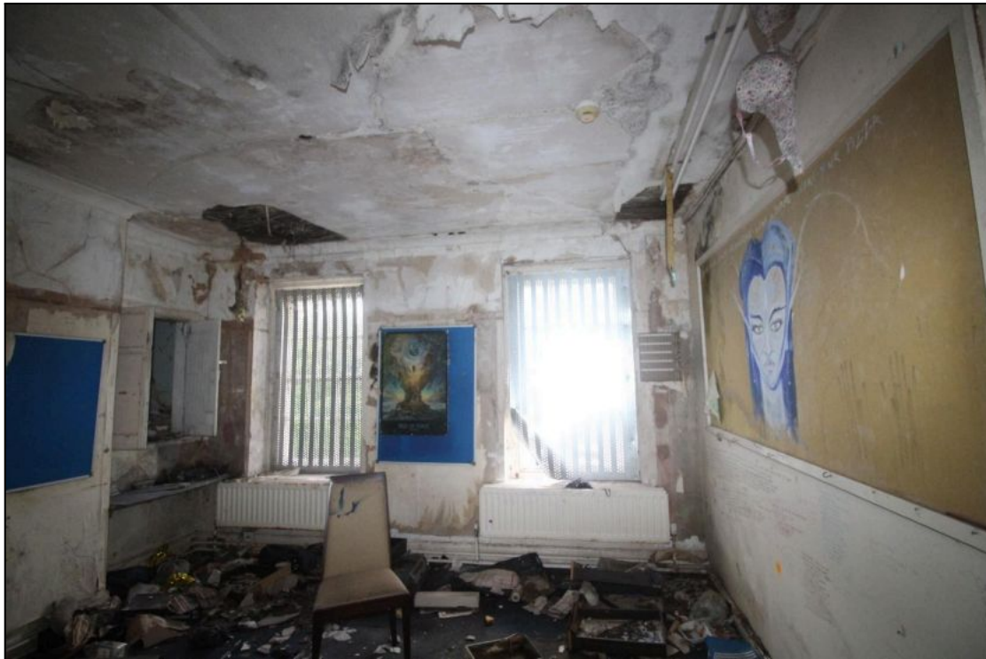
Plate 58: General view of Room 34 on the first floor of the office building, looking west
