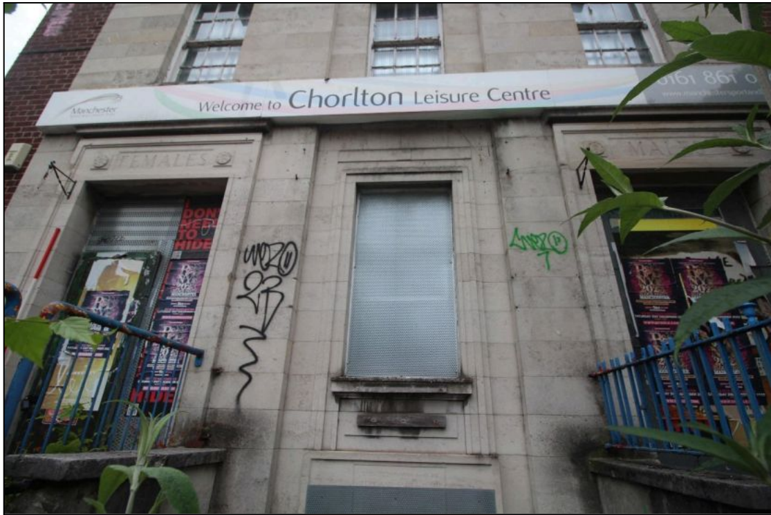
Plate 17: Detail of the central window aperture of the office building, looking west
