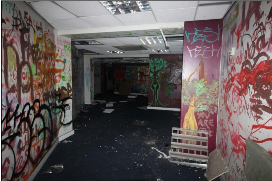
Plate 43: General view of the modified changing rooms (Rooms 6 and 7), facing north
