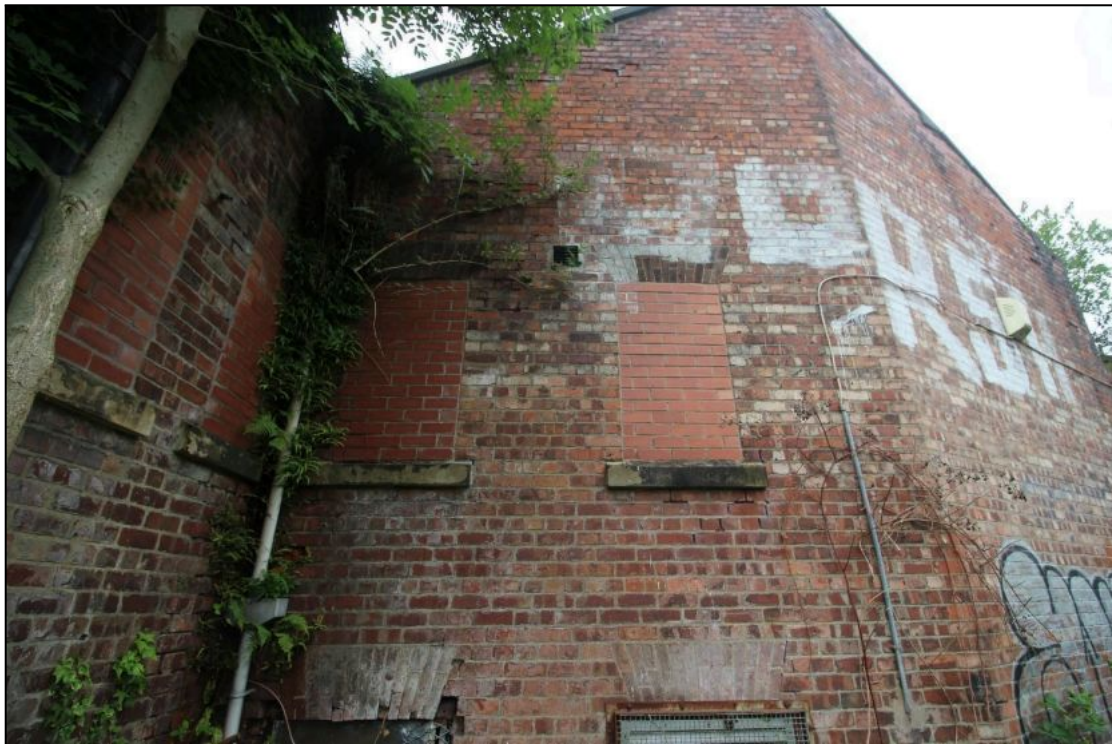
Plate 25: Detail of the blocked windows within the southern half of the gable walls, looking west
