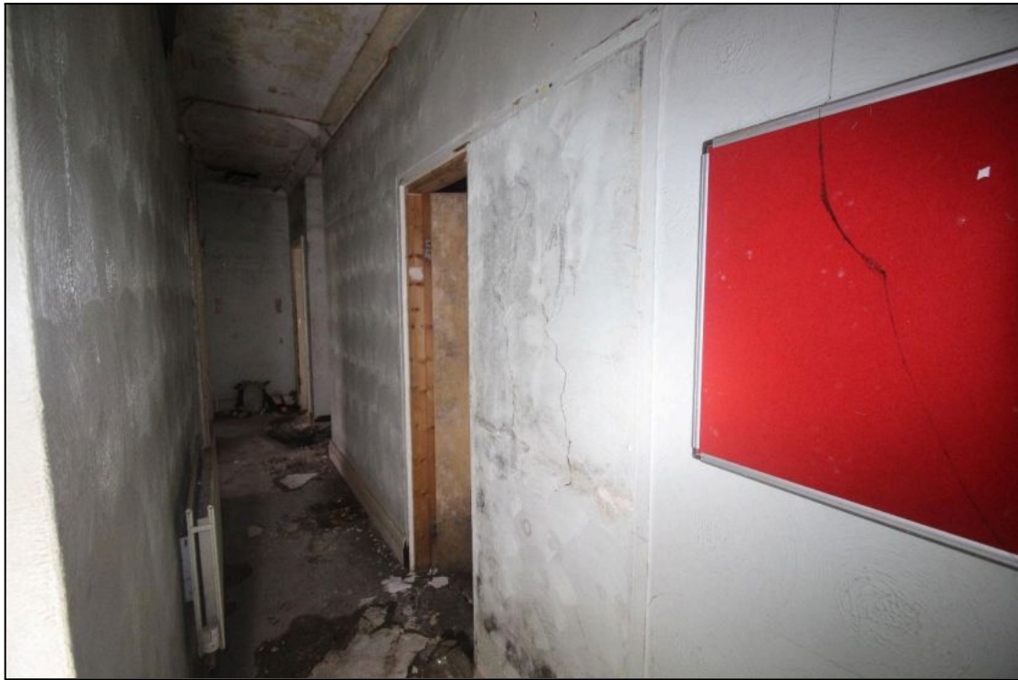
Plate 56: The first-floor corridor within the office building, looking east
