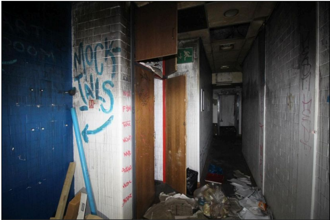
Plate 41: General view of the corridor affording access into the changing rooms (Room 4), facing east
