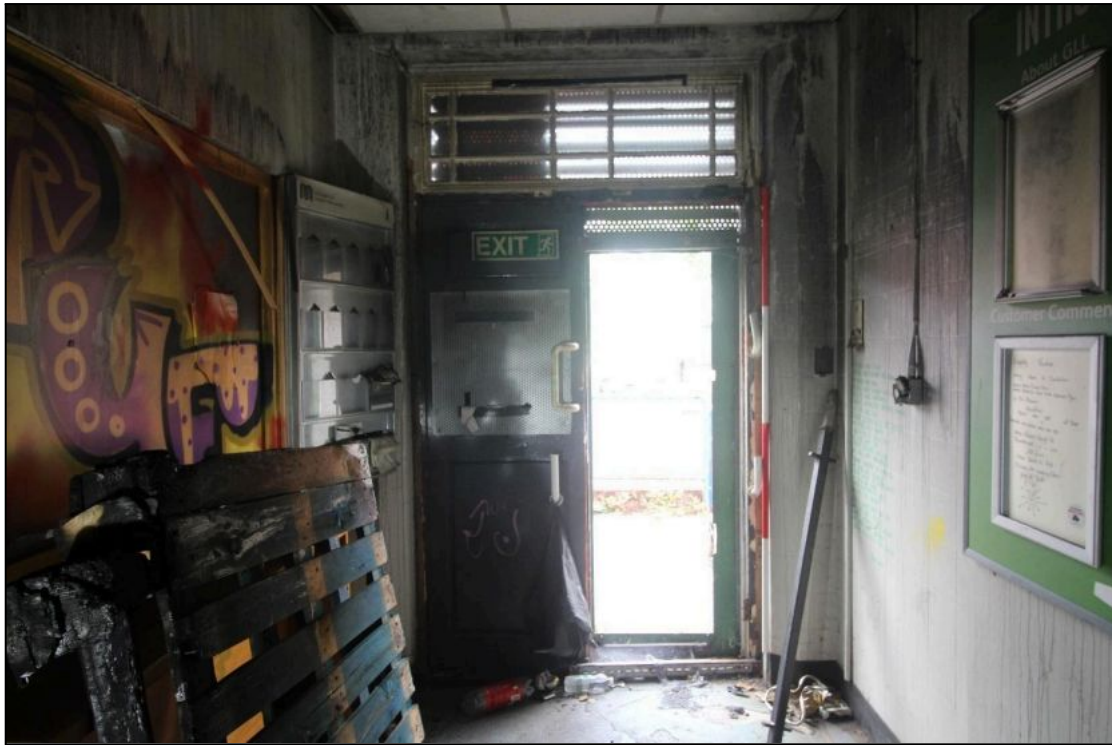
Plate 28: Detail view of the principal entrance into the leisure centre, looking west
