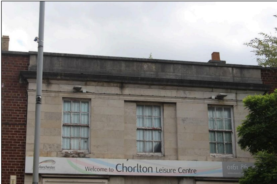
Plate 20: Detail of the first floor of the eastern elevation, looking west
