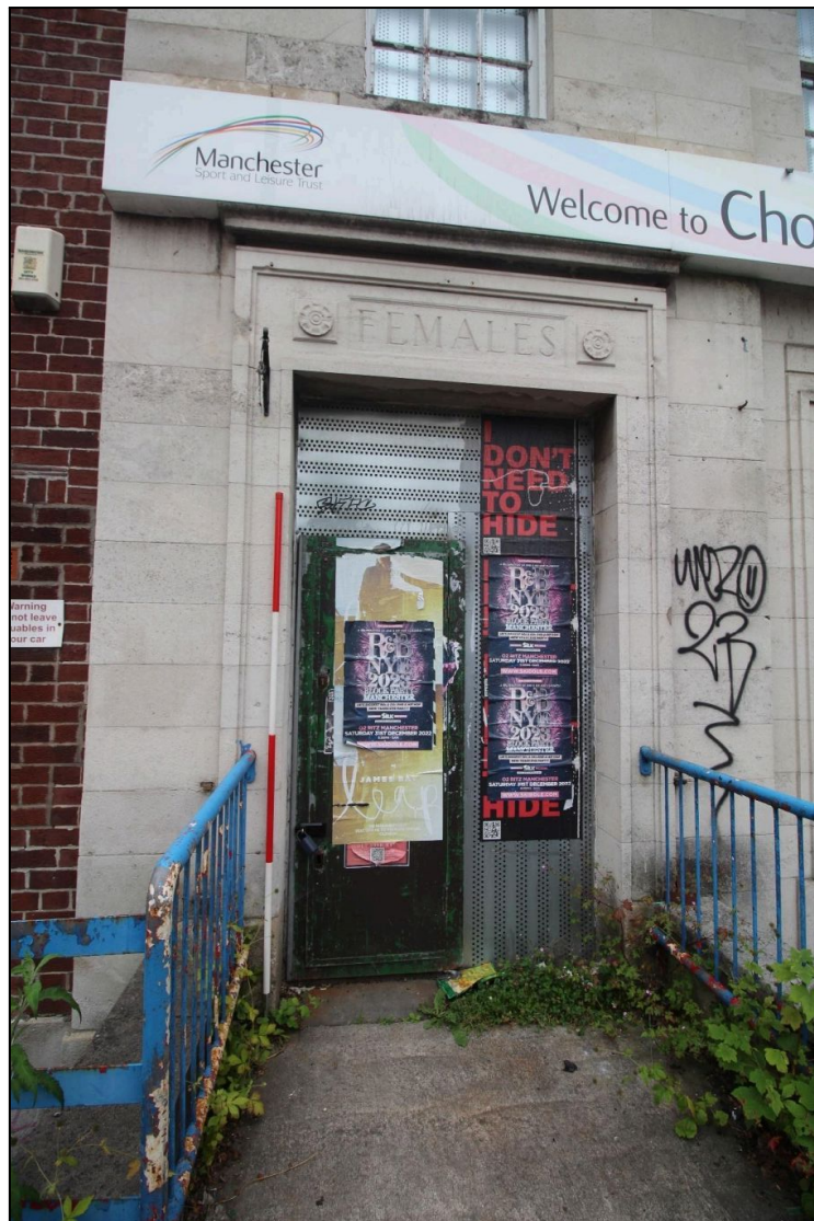
Plate 18: Detail of the northern doorway affording access into the female baths, looking west
