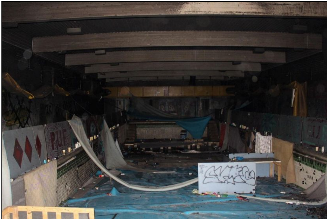
Plate 35: General view of the female pool (Room 3) prior to the demolition, looking north
