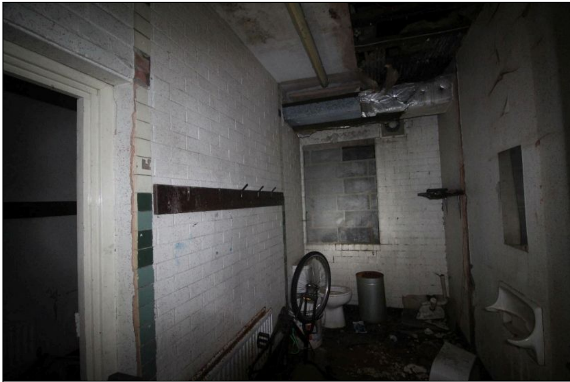
Plate 49: General view of Room 19, looking east
