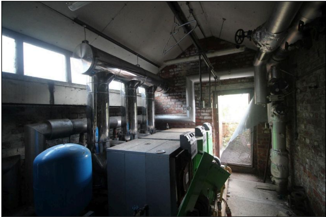
Plate 52: The eastern room of the plant room, looking east
