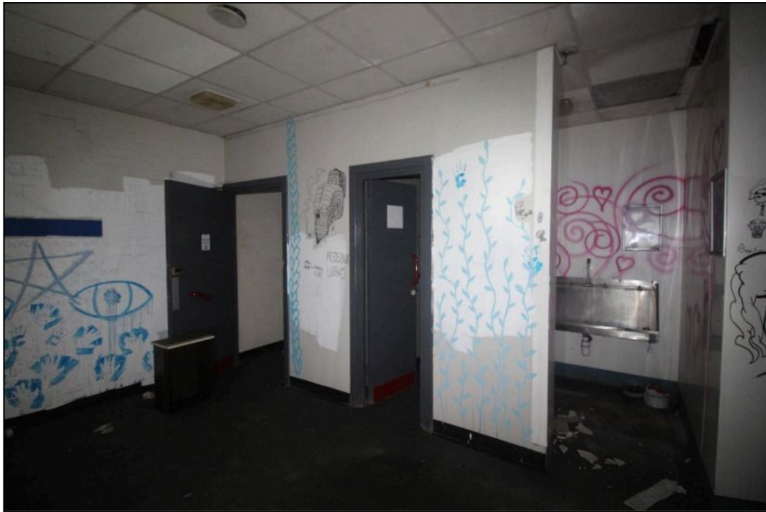
Plate 44: General view of the modified male changing rooms (Rooms 8), facing south-east
