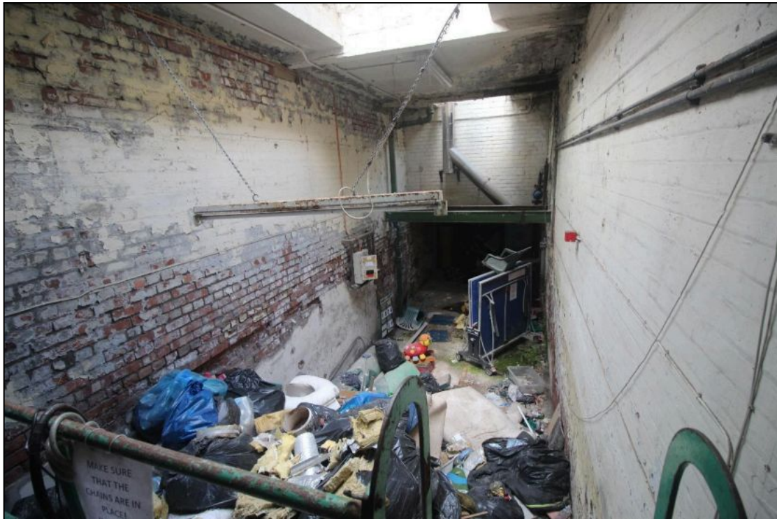
Plate 51: The western room of the plant room, looking west
