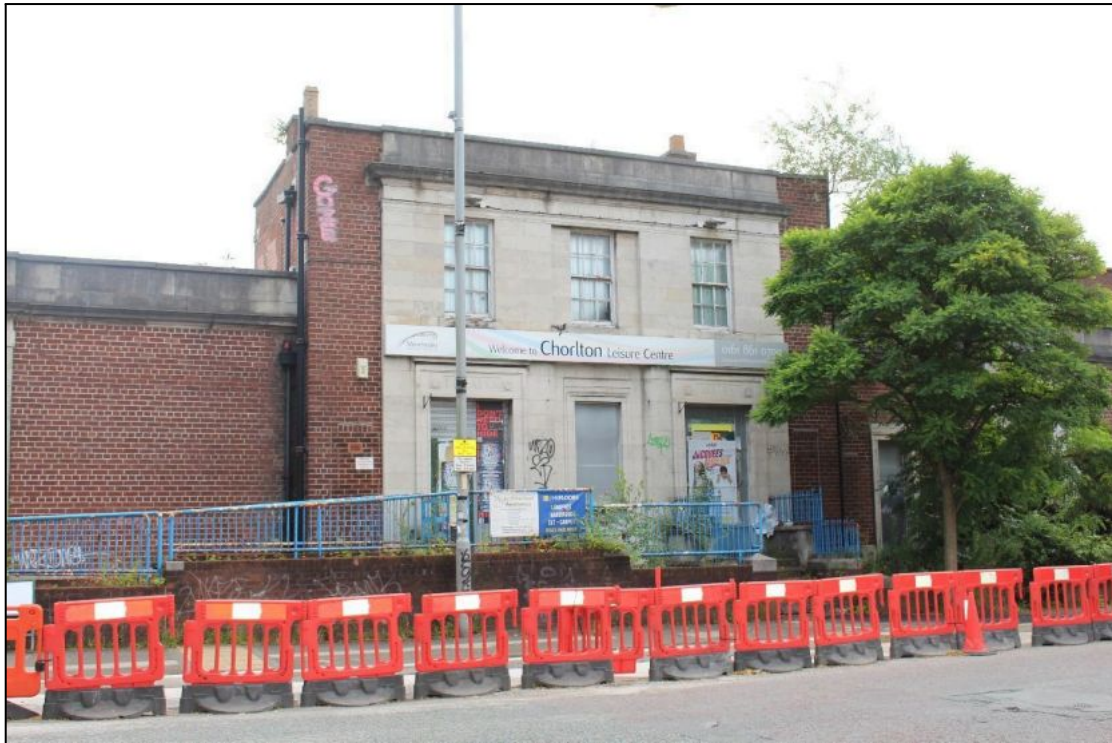
Plate 16: General view of the western elevation of the office and reception building, looking south-east
