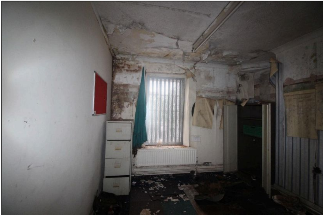
Plate 60: General view of Room 35 on the first floor of the office building, looking west
