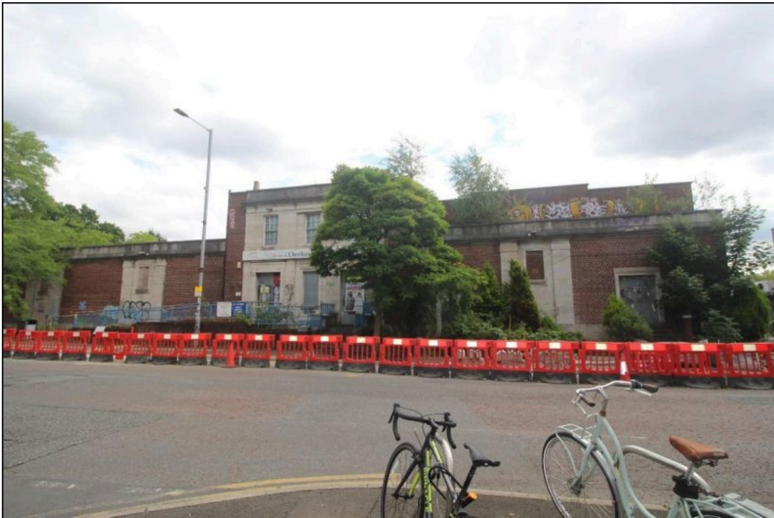
Plate 9: General view of the western elevation of Chorlton Leisure Centre, looking east
