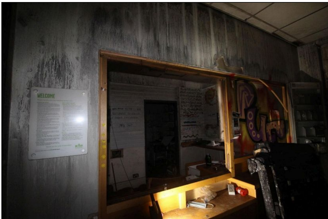
Plate 32: The inserted reception window within the southern wall of Room 1, looking south-west
