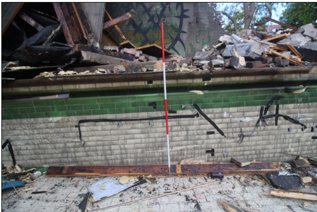
Plate 38: Detail of the female pools tiled wall and floor during the watching brief
