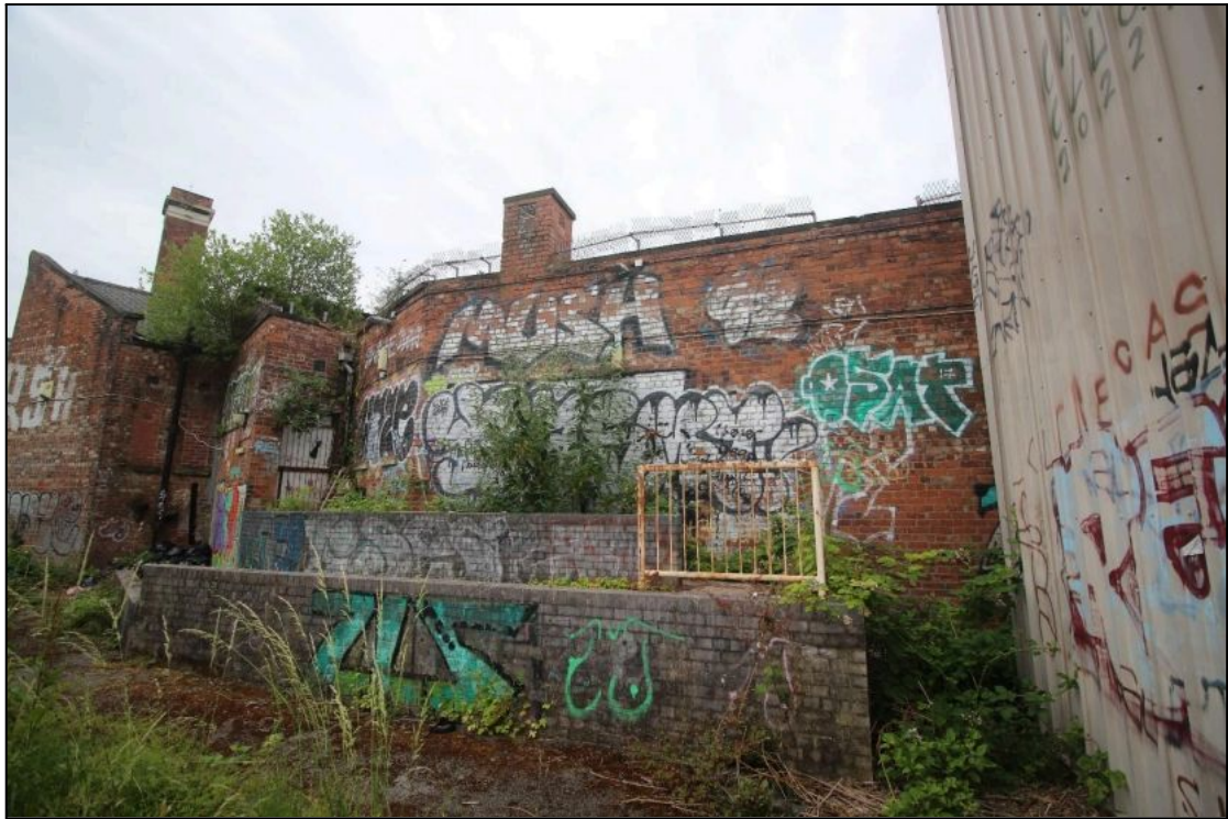
Plate 23: General view of the northern section of the eastern elevation, looking west
