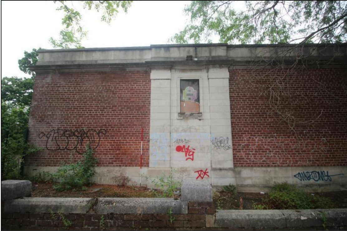
Plate 11: Detail of the Portland stone recessed panel at the northern end of the western façade, looking east
