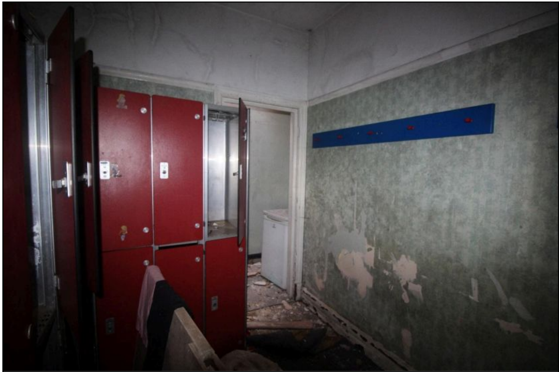
Plate 57: General view of Room 32 on the first floor of the office building, looking north-east
