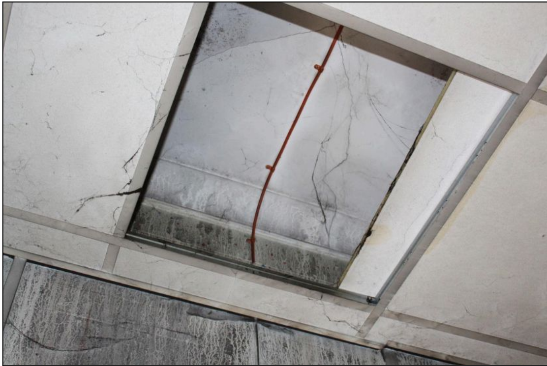
Plate 31: Detail of the original ceiling of Room 1
