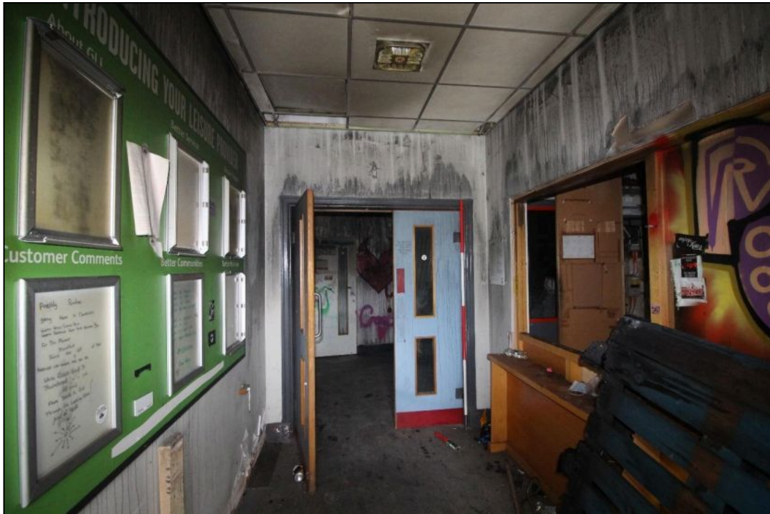
Plate 29: General view of Room 1, looking east
