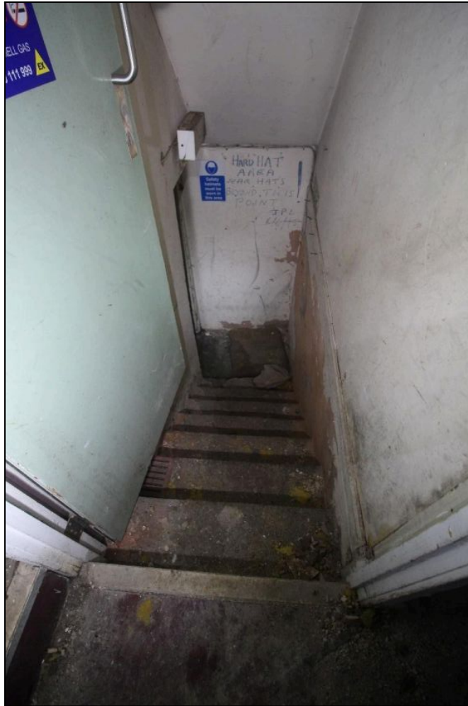
Plate 61: The stairwell descending to the basement, looking east
