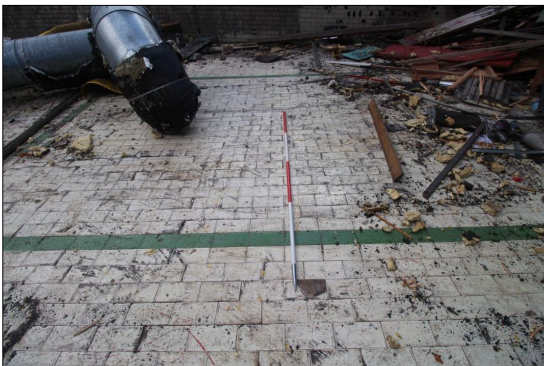
Plate 39: Detail of the female pools tiled floor during the watching brief
