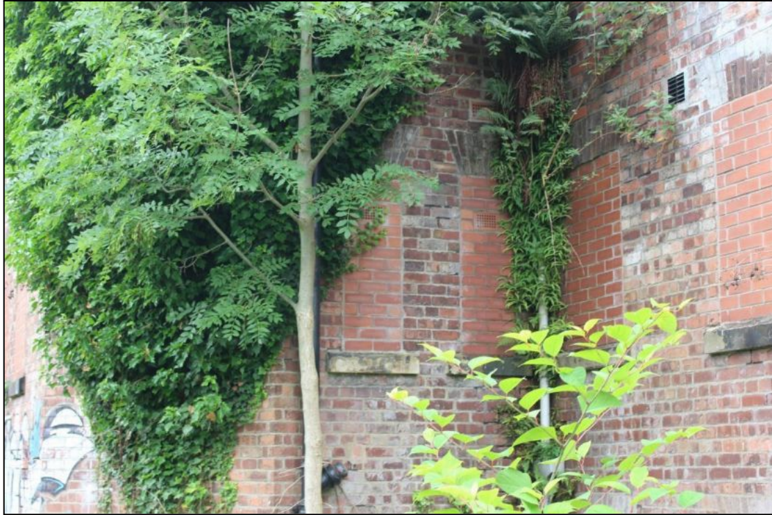
Plate 26: Detail of the blocked windows within the southern elevation of the southern bay, looking south
