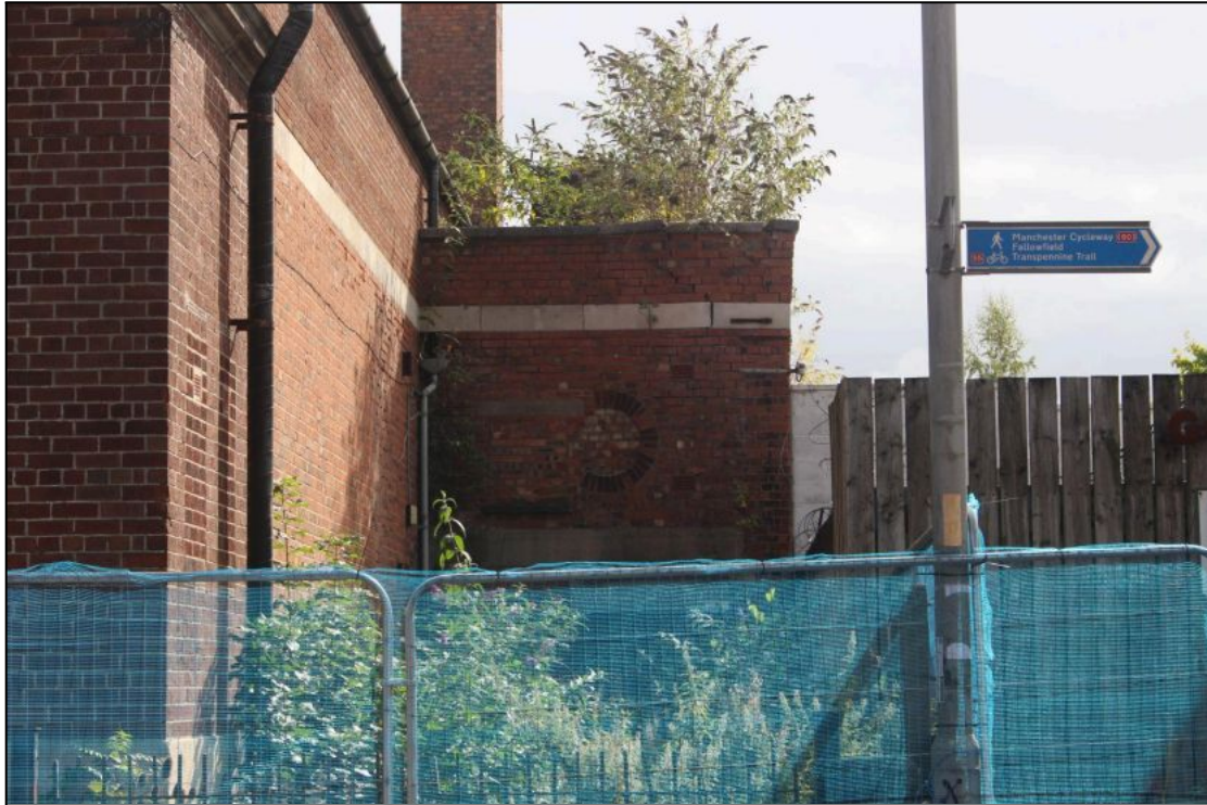
Plate 15: General view of the western elevation of the attached plant room, looking east
