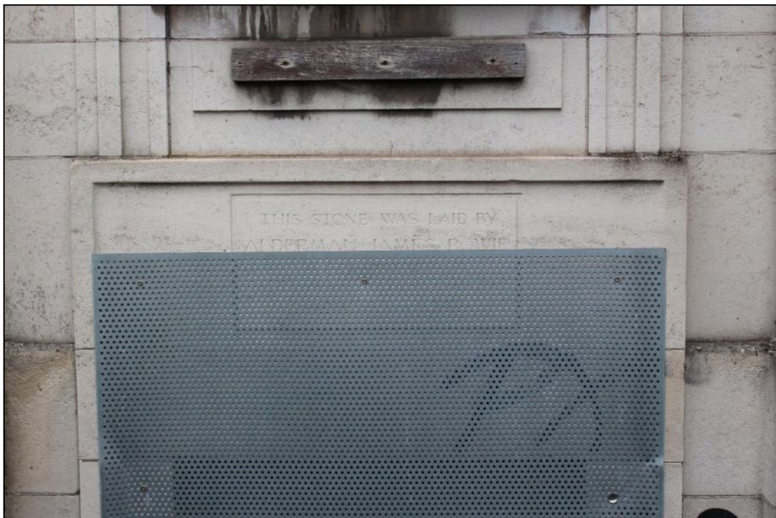
Plate 21: Detail of the inscription above the doorway affording access into the basement, looking west
