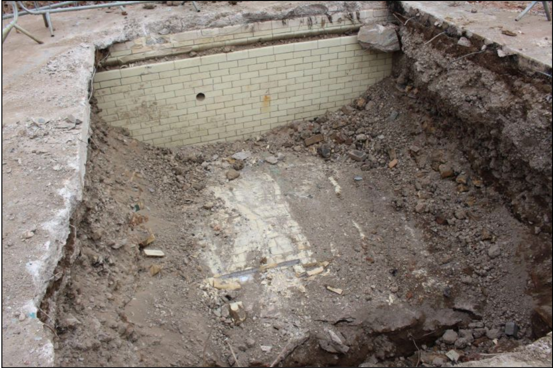
Plate 47: Detail of the male pool's tiled wall and floor during the watching brief, looking north
