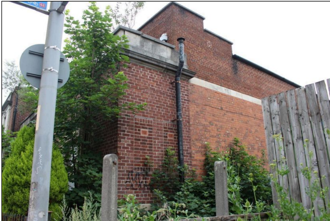
Plate 27: General view of the southern elevation of the male baths, looking north-east
