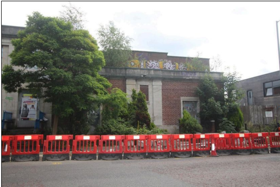
Plate 12: General view of the western façade of the male bath, looking east
