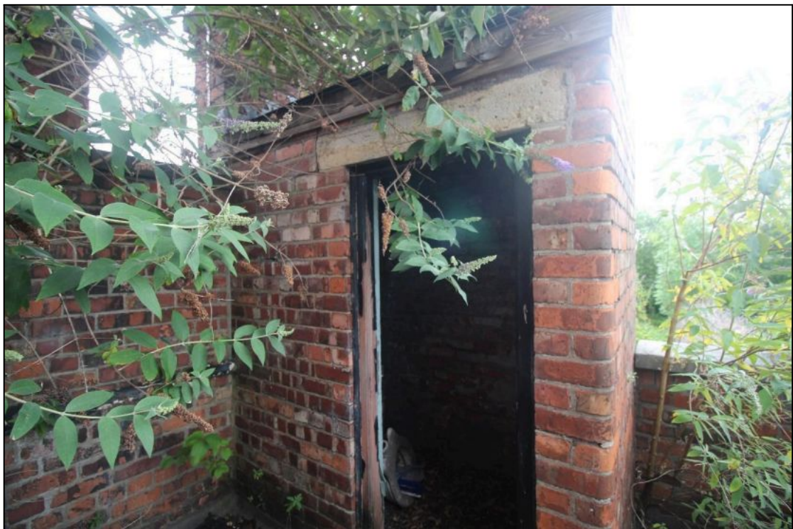
Plate 53: The outside privy at situated to the north-eastern corner of the plant room
