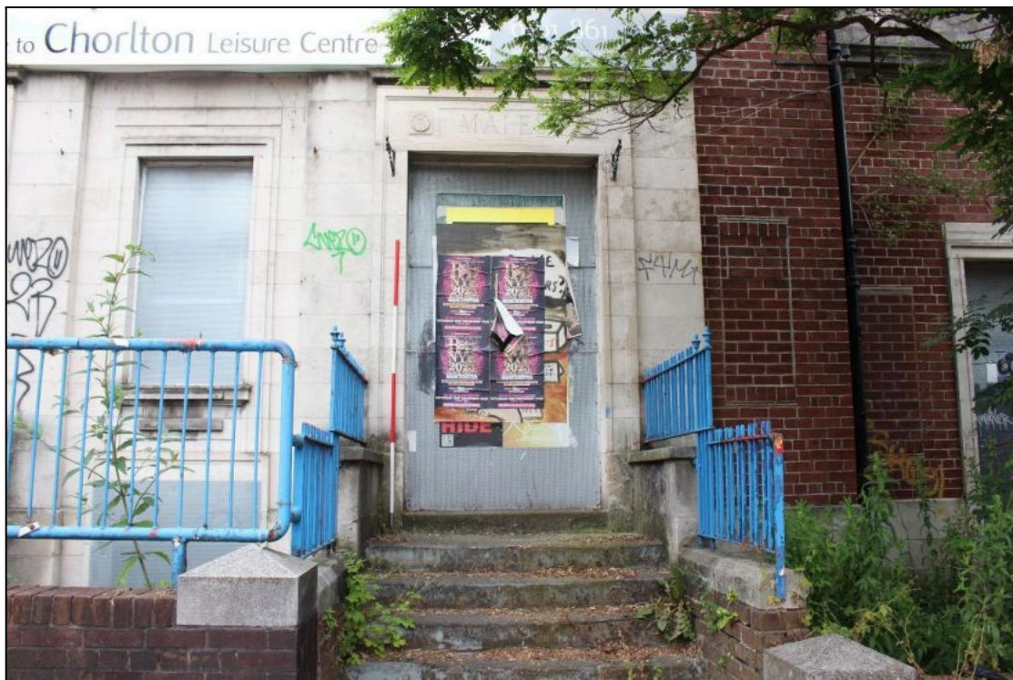
Plate 19: Detail of the southern doorway affording access into the male baths, looking west
