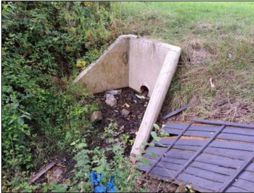
Photograph 11 showing the outfall
