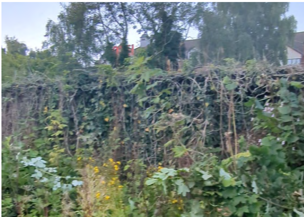
Photograph 16 – Building 4 heavily concealed by vegetation.
