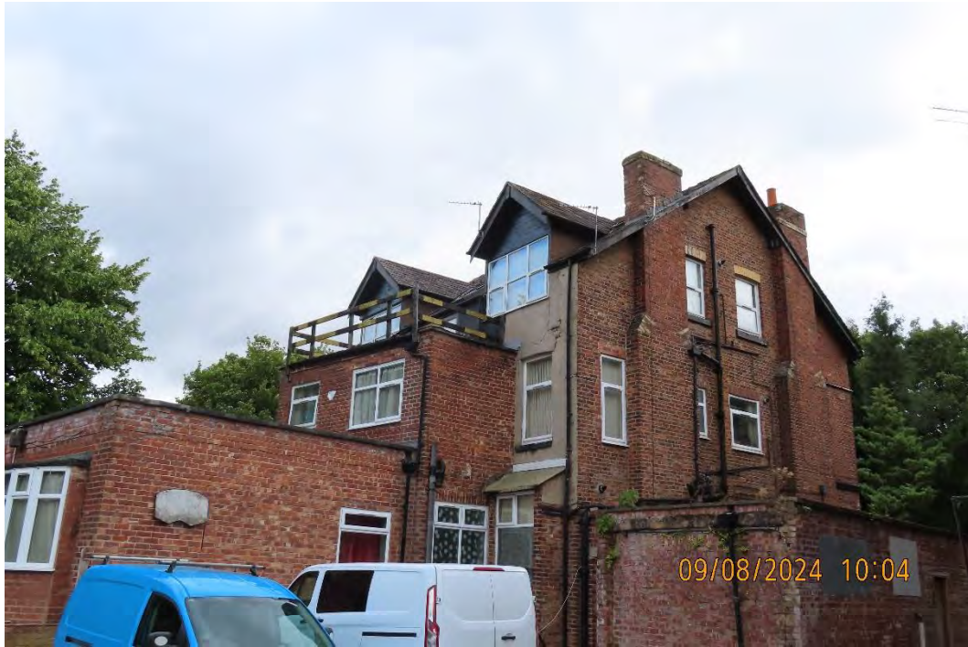
Photograph 11 – South-western aspect of Building 3, featuring the north-western extension and south-western garage.
