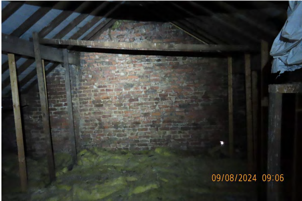
Photograph 17 – Internal loft space of Building 1.
