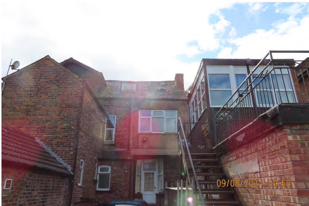
Photograph 6 – North-western aspect of Building 2 including the extensions.
