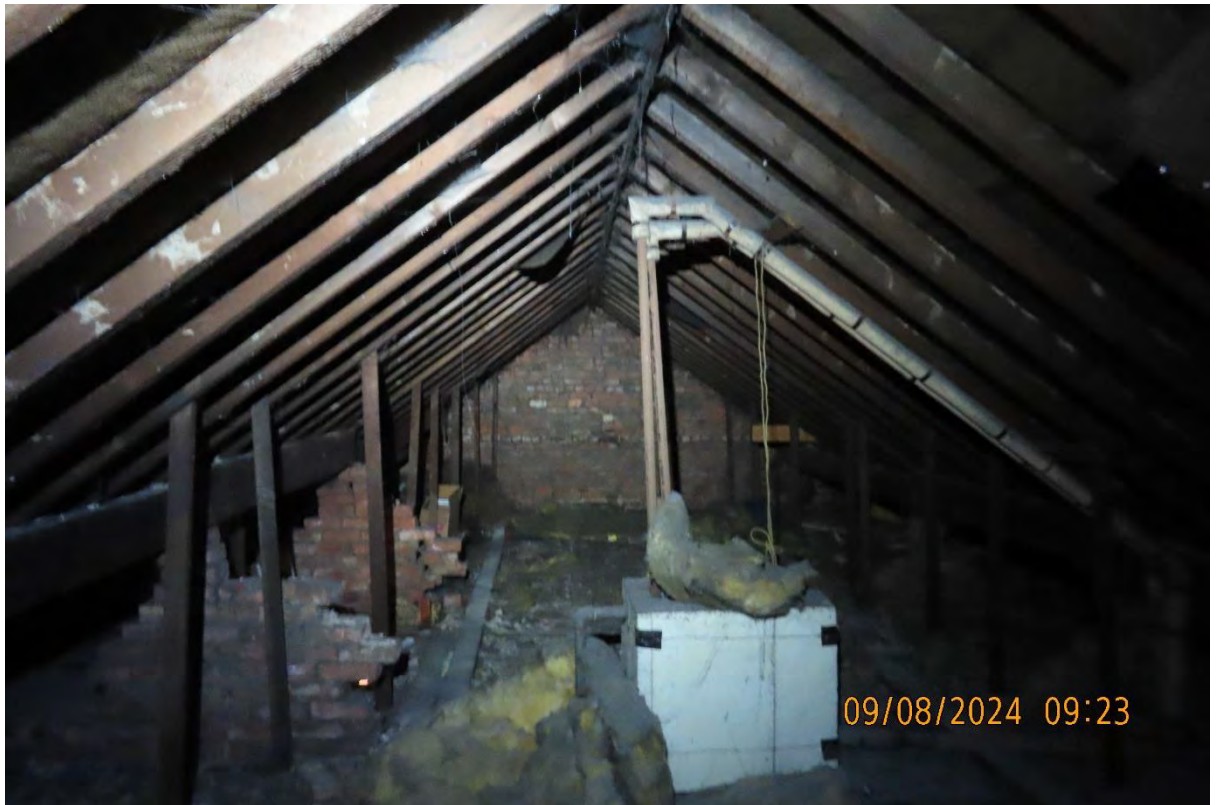
Photograph 21 – Internal loft void of Building 3.
