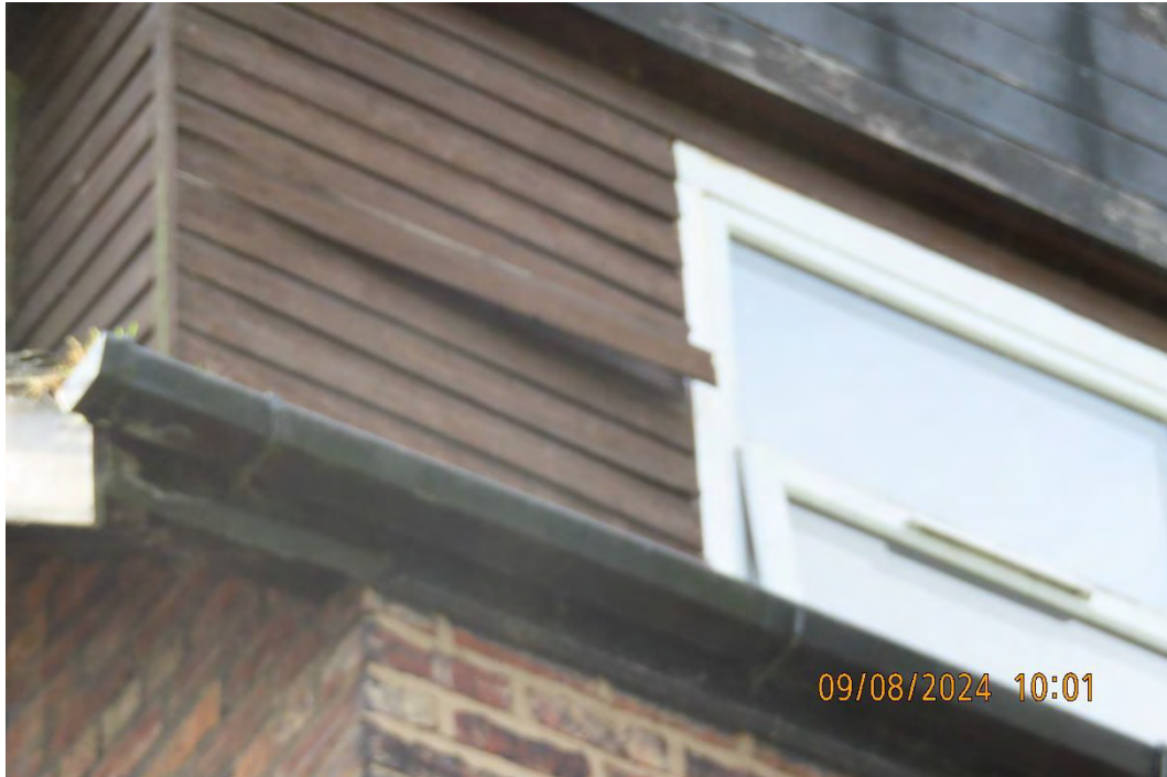
Photograph 7 – Timber cladding present on a dormer featuring raised slats at Building 2.
