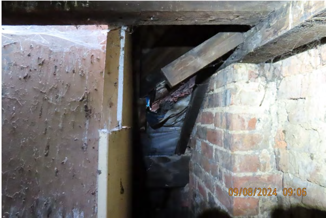
Photograph 19 – Access point at the southern aspect of the loft void of Building 1.
