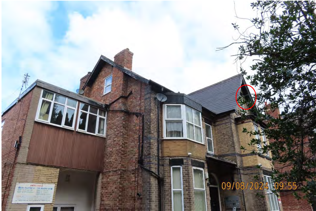
Photograph 5 – South-eastern aspect of Building 2. Roost 1 location highlighted.
