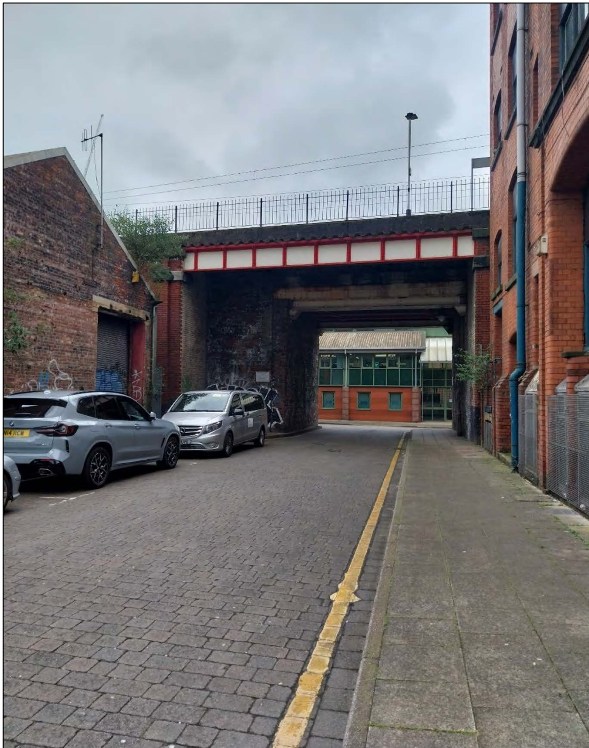
Plate 16 View of Rowendale Stret, looking broadly south, showing the Grade II Listed Manchester South Junction and Altrincham railway viaduct
