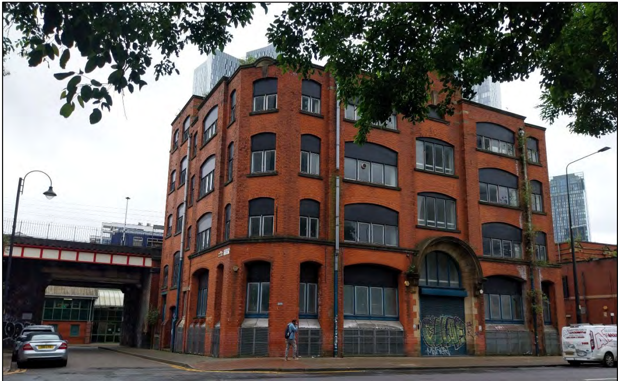
Plate 13 Photograph showing Wrendal House, looking south-west from Whitworth Street West
