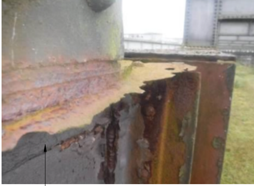
Example 2 - Span 4, south truss
