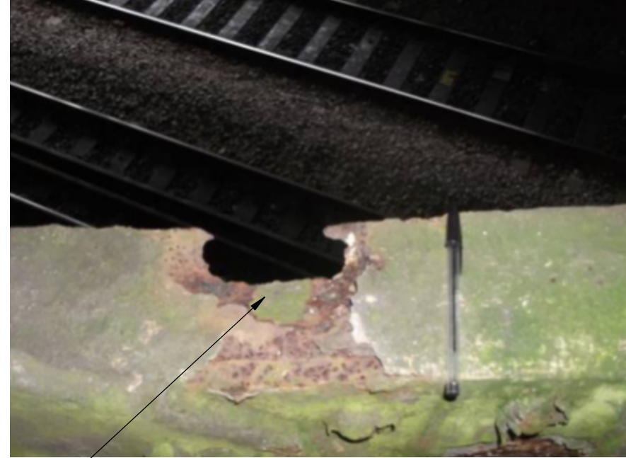
Example 2 - Span 1, south truss
