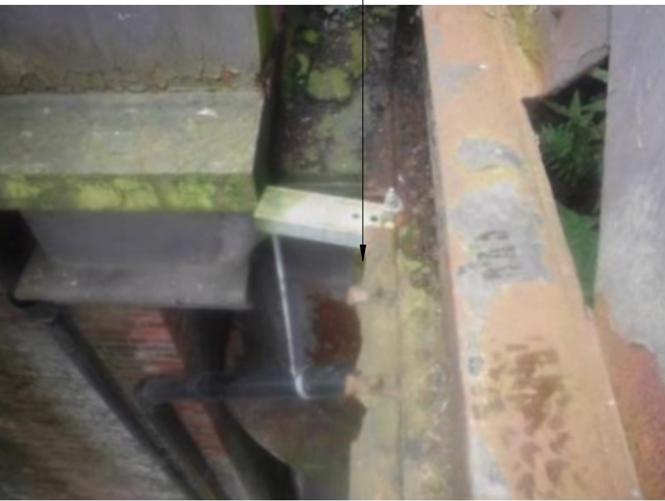
Example 4 - Span 7, south truss
