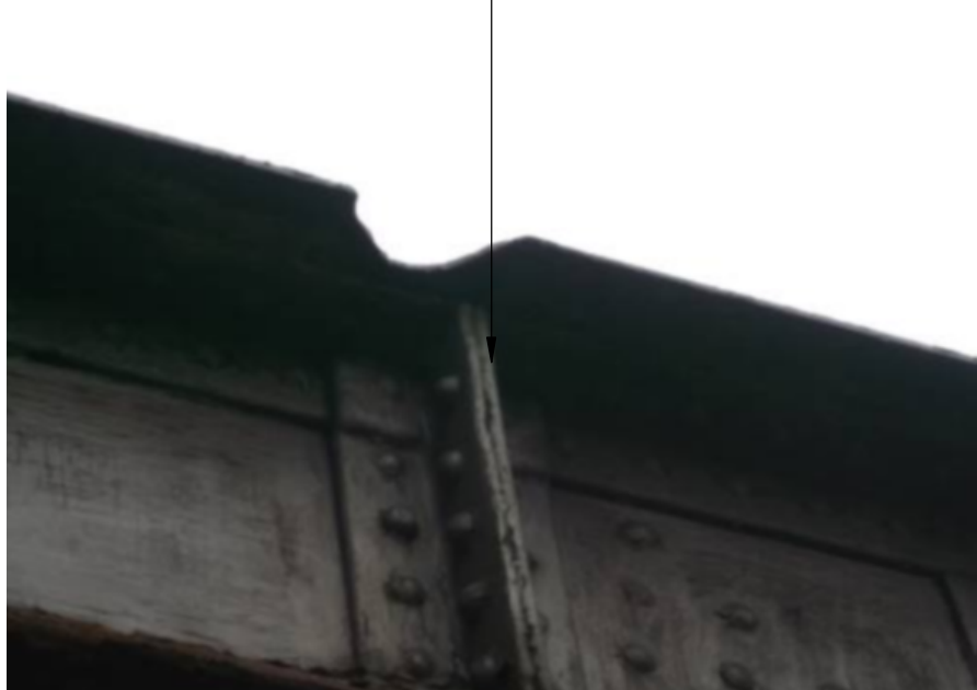
Example 6 - Span 6, north truss
