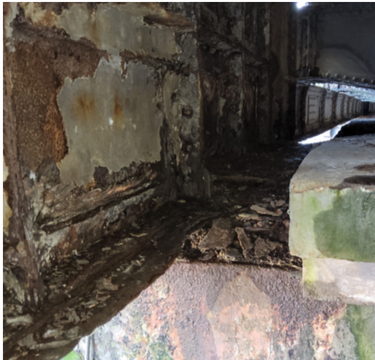
Example 5 - Span 3, north truss
