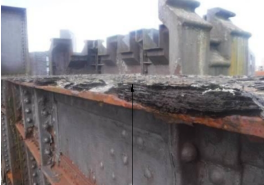
Example 1 - Span 5, north truss
