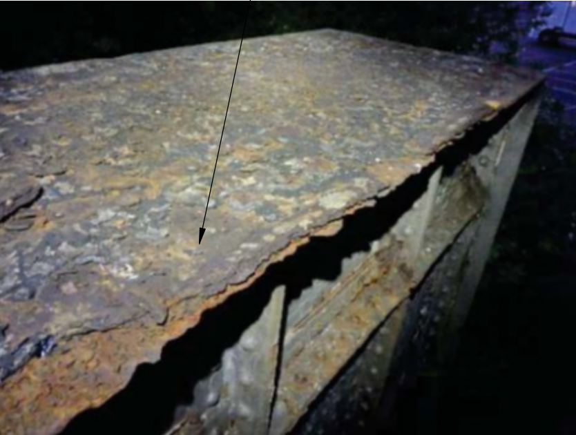
Example 5 - Span 1, south truss
