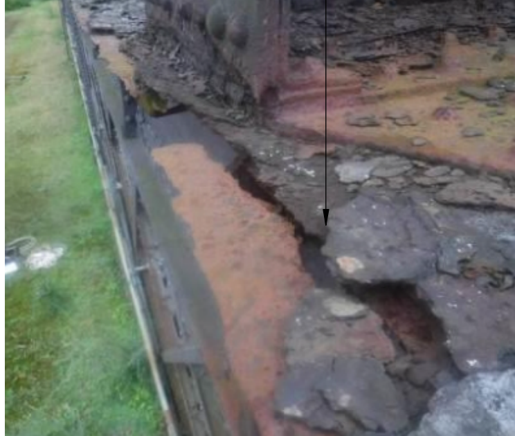
Example 4 - Span 2, south truss
