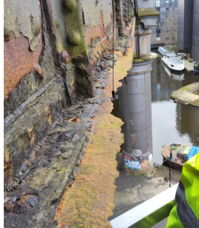
Example 6 - Span 4, north truss
