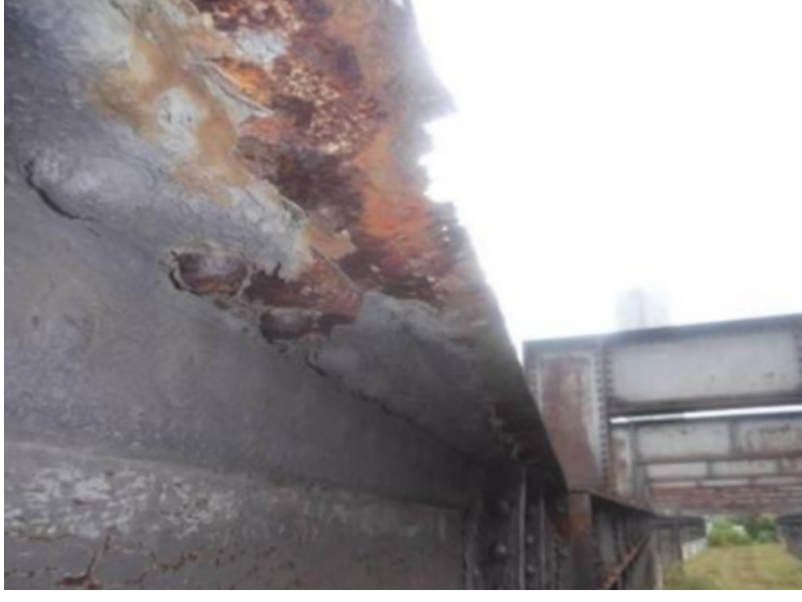
Example 3 - Span 4, north truss
