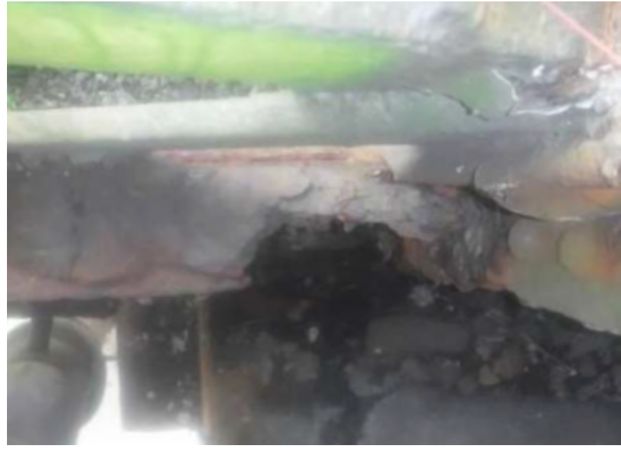
Example 3 - Span 4, south truss
