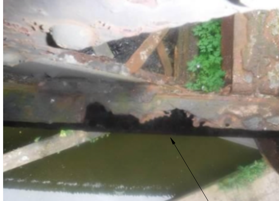
Example 1 - Span 3, south truss
